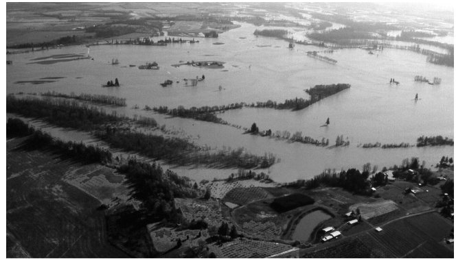
The Pacific Northwest was hit by an historic flood in February 1996. Willamette Valley System dams were put to the test and held back as much of the flood waters as possible, but too much rain fell in the valley below the dams. As a result, many communities in western Oregon felt the impacts of flood waters. Photo credit: U.S. Army Corps of Engineers
