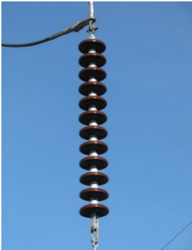
230 kV Riser Bus in Bridge
