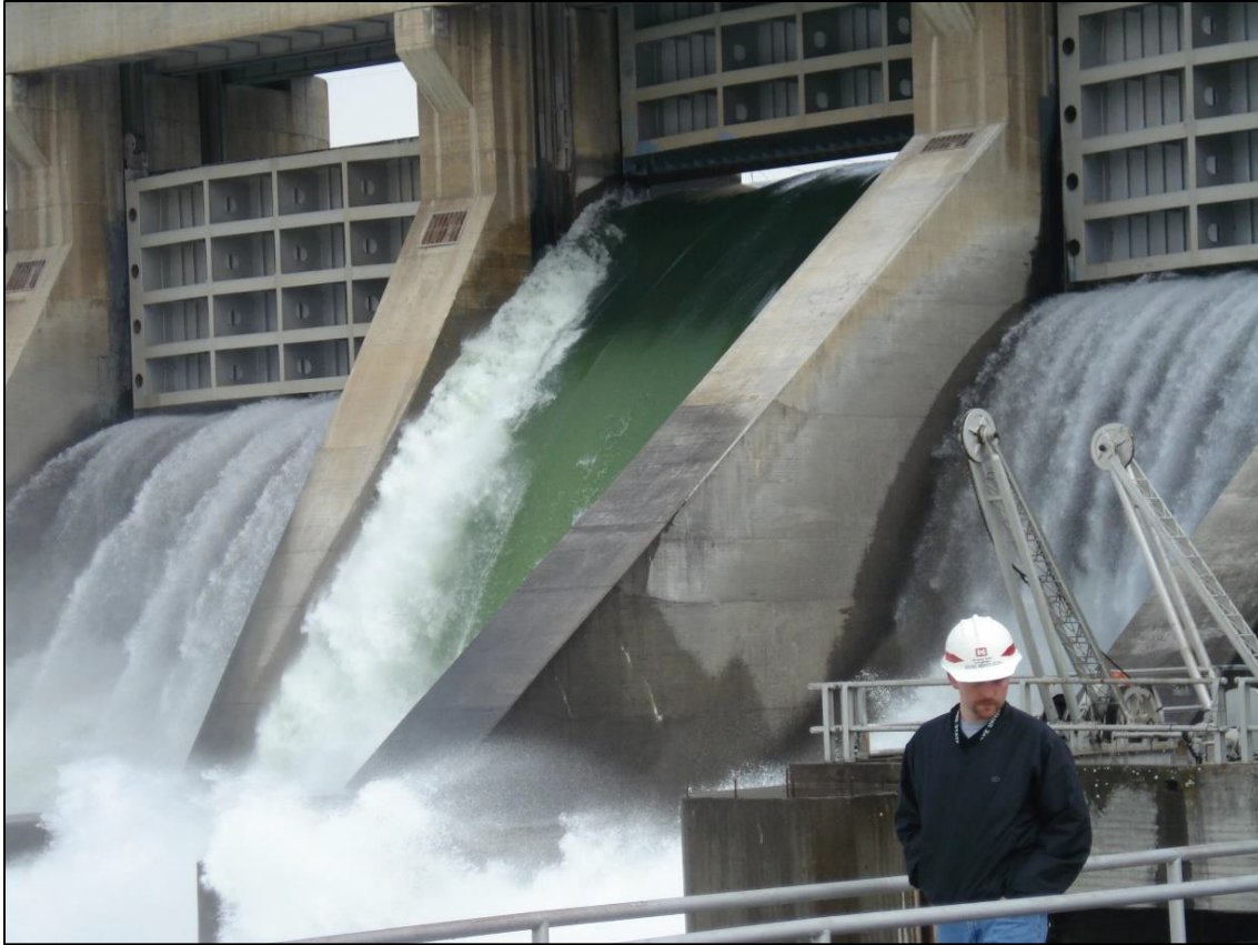
Figure E-3. A spillway weir in operation at McNary Dam (surface spill shown in middle, bottom spill to left and right)
