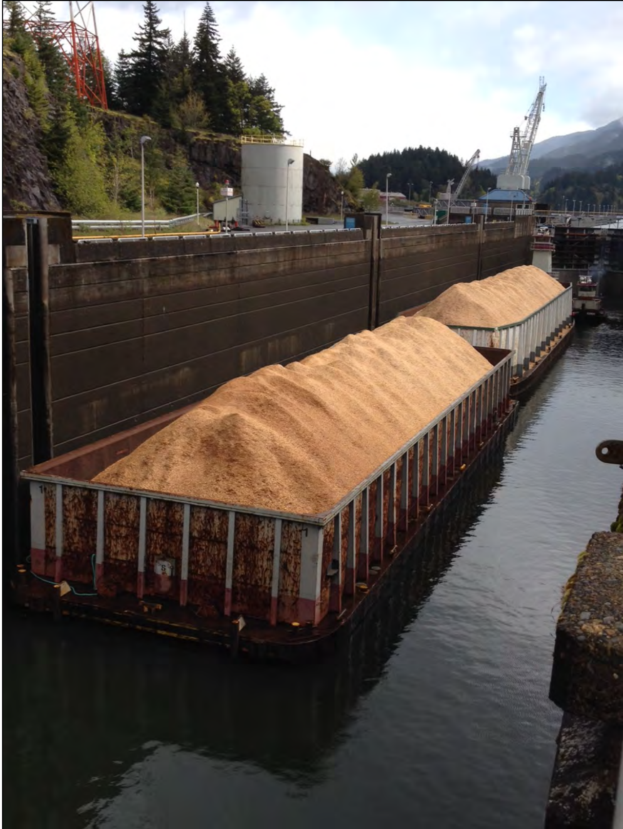
Figure 3-213. Vessels in Navigation Lock
