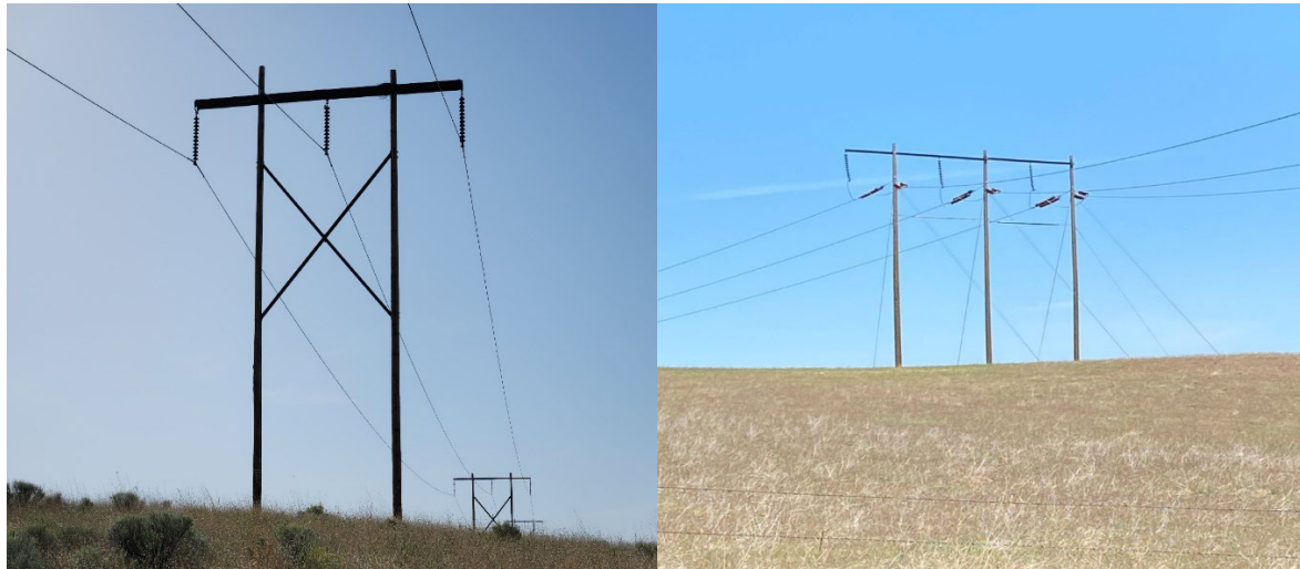
Figure 1-2. Existing Structures in the ROW
