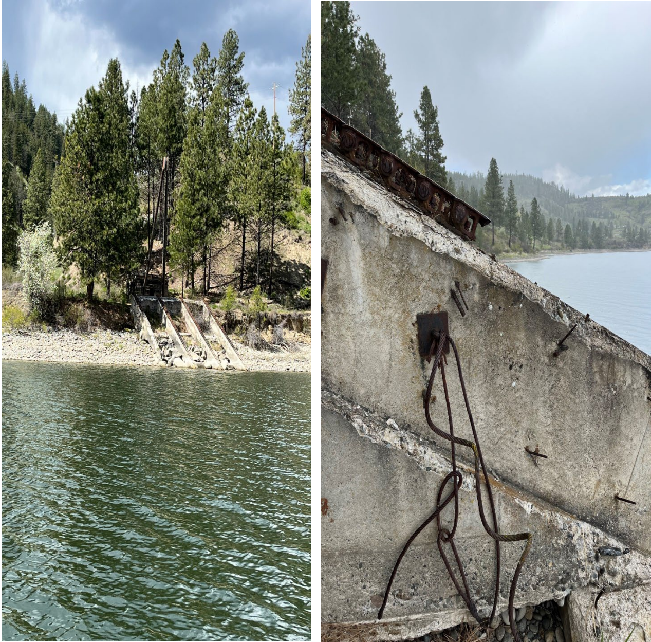
Figure B-5. Photo of the upper log landing, which is on Colville Tribal government-owned land on the Colville Reservation. The close-up side view shows an existing I-bolt with cable. The existing I-bolt may be usable as an attachment point if a shore-based anchor deployment is used at this site. A new I-bolt could also be attached to the concrete to serve as a new attachment point.
