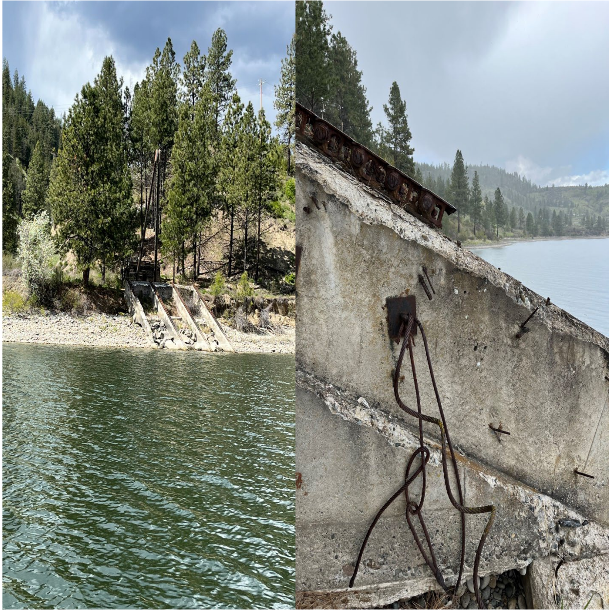
1 Figure B-5. Photo of the upper log landing, which is on Colville Tribal government-owned land on the 2 Colville Reservation. The close-up side view shows an existing I-bolt with cable. The existing I-bolt may be 3 usable as an attachment point if a shore-based anchor deployment is used at this site. A new I-bolt could 4 also be attached to the concrete to serve as a new attachment point.
