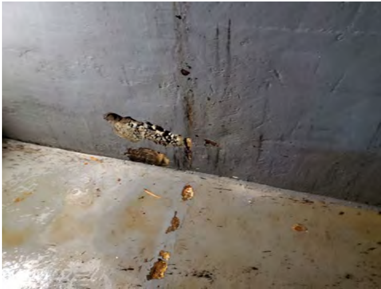
Figure 2.2-4. Photo of Cavitation Damage to Upper RO Tunnel
