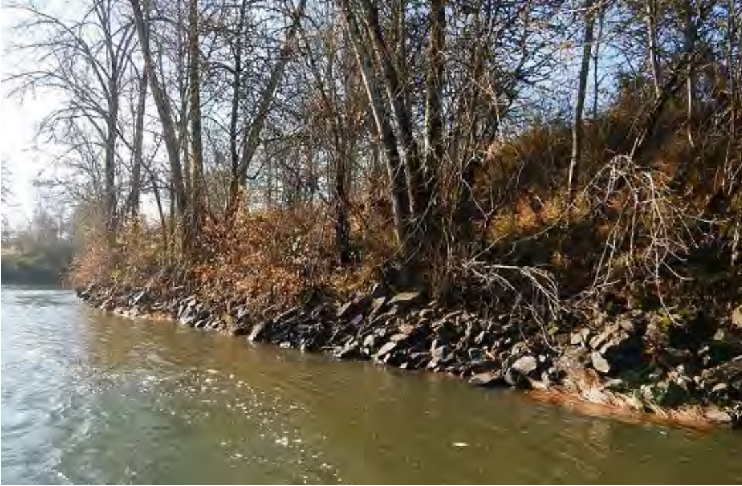
Figure ES-9. Riprap (a type of revetment) on the bank of the Willamette Mainstem near Corvallis
