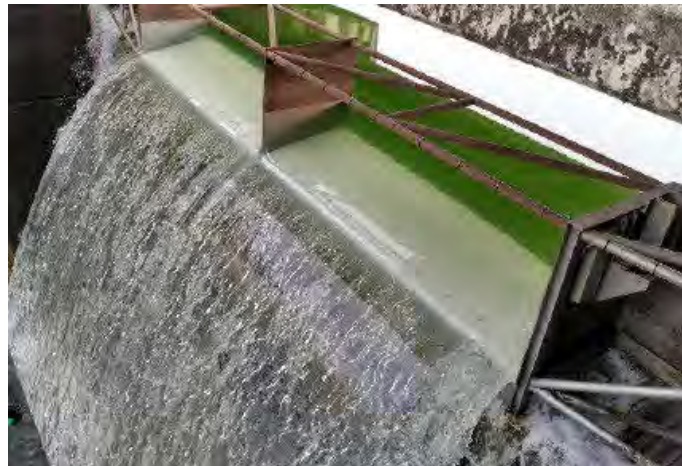
Foster Spill Weir for downstream fish passage - 2018
