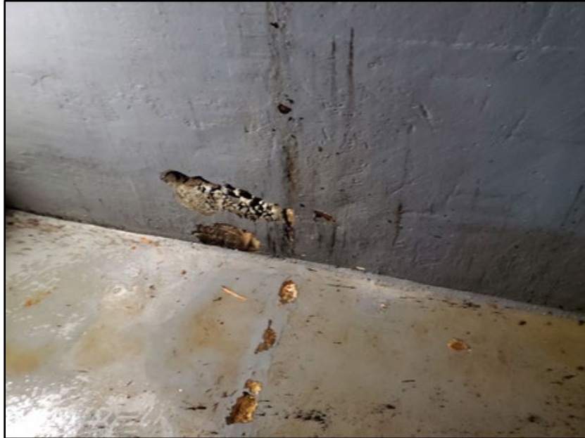
Figure 2.8-5. Photo of Cavitation Damage to an Upper Regulating Outlet Tunnel.
