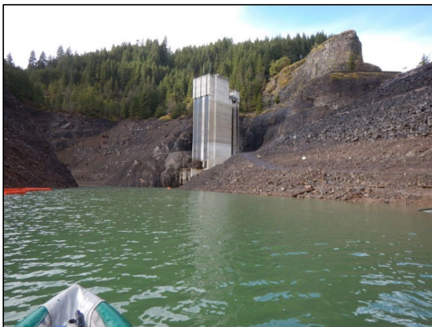
Figure 2.8-1. Water Temperature Control Tower at Cougar Dam and Reservoir.
