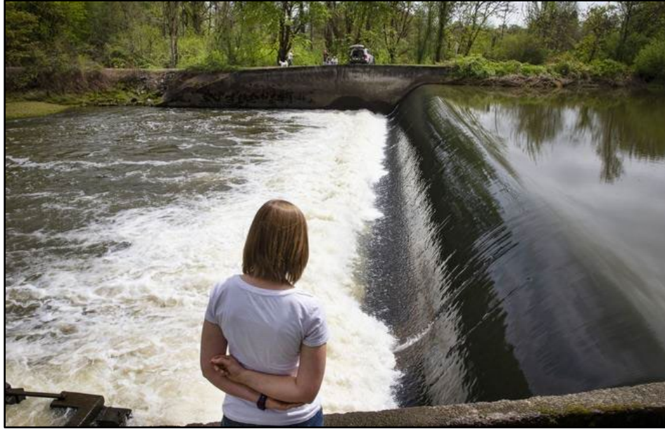
Figure 2.8-14. Drop Structure Downstream of the Fern Ridge Dam.
