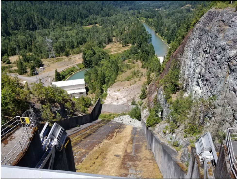
Figure 2.8-9. Hills Creek Dam Spillway Channel.
