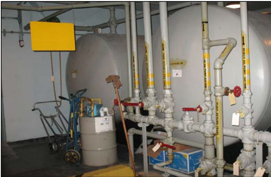
Figure 3.16-1. Primary Transformer Insulating Oil Stored in the Oil Treatment and Storage Room of the Detroit Dam Powerhouse.
