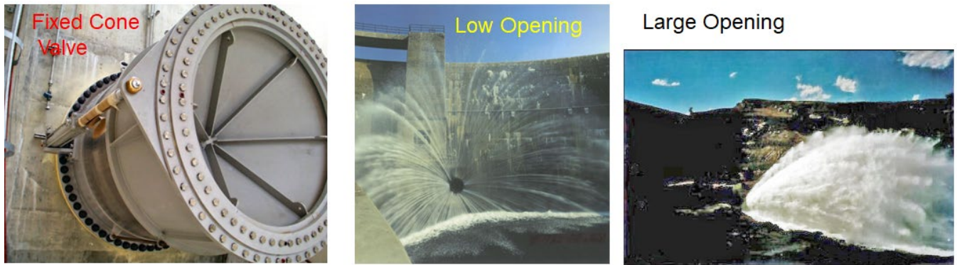
Figure 2-12. Standard Cone Valve with Conical Spray at Boulder Dam, Colorado
