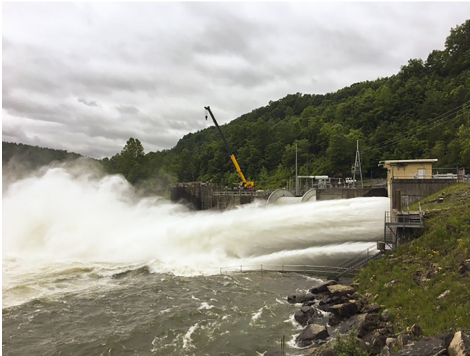
Figure 2-13. Hooded Cone Valve Operations at Summersville Dam, West Virginia
