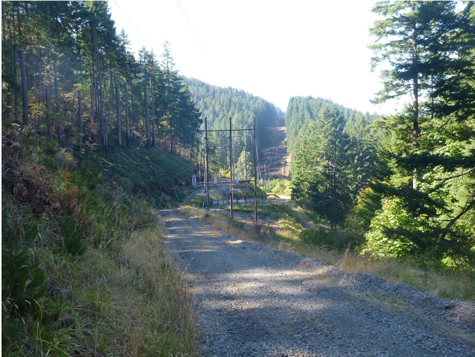
Figure C-27. View to West Showing Post-fire Conditions in Line Mile 7 of Right-of-Way.
