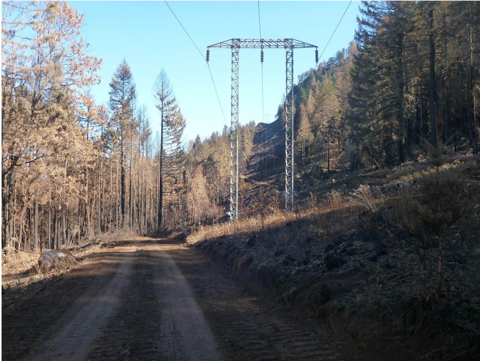
Figure C-26. View to East Showing Post-fire Conditions in Line Mile 2 of Right-of-Way.
