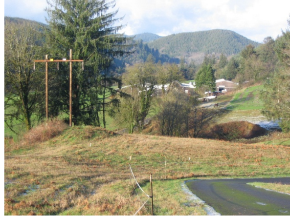
FIGURE 3-11. EXISTING TRANSMISSION LINE AT THE LOCATION OF THE ACCESS ROAD TO BE CONSTRUCTED NEAR STRUCTURE 17/1
