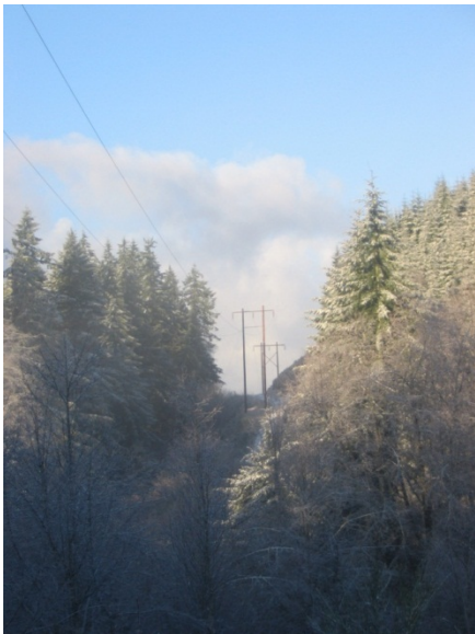
FIGURE 3-8. EXISTING TRANSMISSION LINE NEAR STRUCTURE 5/2
