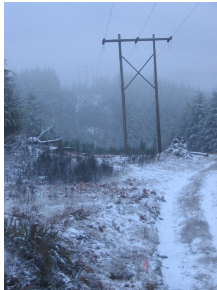
FIGURE 3-9. EXISTING ACCESS ROAD NEAR STRUCTURE 6/4
