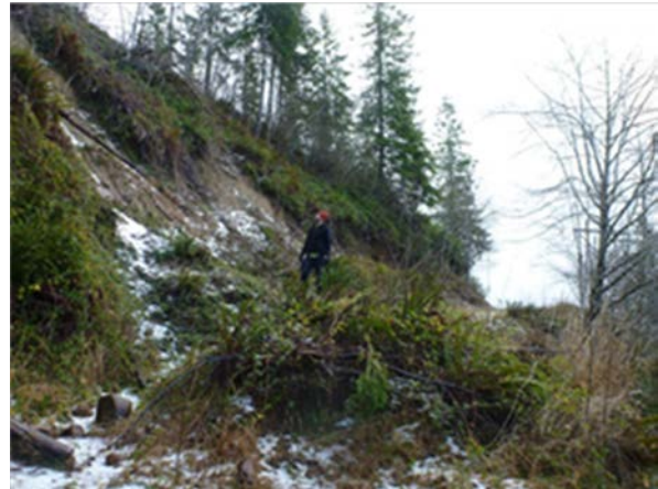
FIGURE 3-3. LANDSLIDE EVIDENCE ON A PROJECT ROAD NEAR STRUCTURE 14/1
