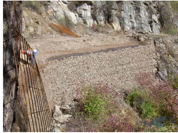
FIGURE 2-11. EXAMPLE OF RETAINING WALL CONSTRUCTION
