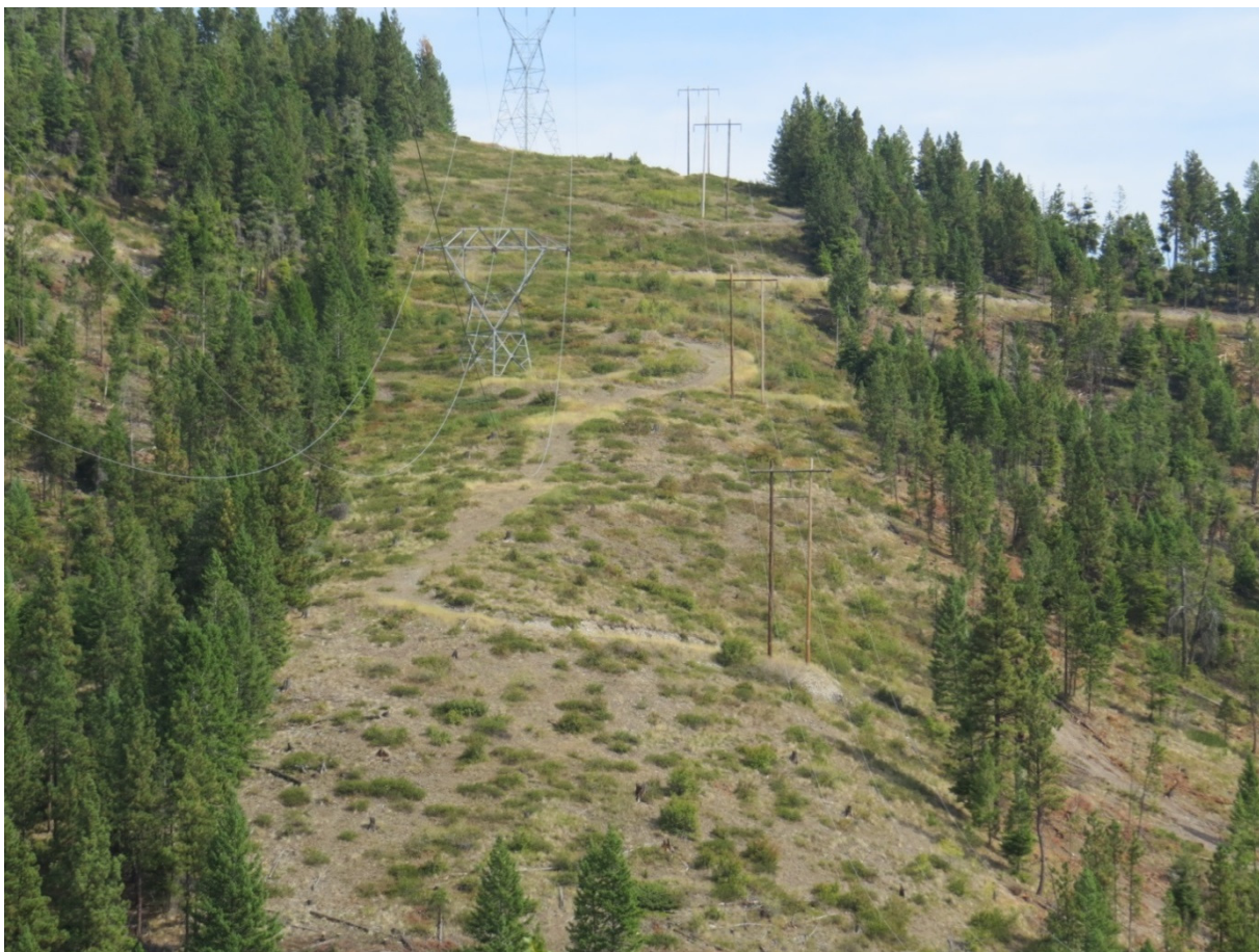
Figure 3.3-1. Looking North at Line Mile 20: Steep Slopes, Exposed Bare Ground, and Gravel Access Road Switchbacks Across the Transmission Line Right-of-Way
