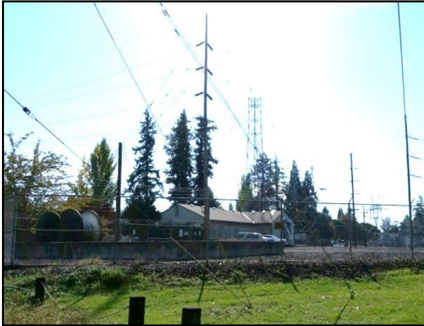
Photograph 2-11. BPA Albany Substation viewed from Hazelwood Park.
