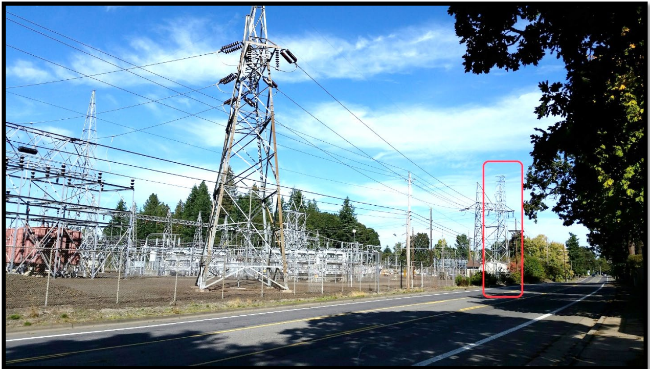
Figure F-2 (below): Looking north at the eastern chain link fence of BPA's Albany Substation; Queen Avenue in the forefront of the picture. Under Alternative 2A or 3C, new communications equipment would be installed on the steel-lattice structure in the red rectangle (same structure as pictured in Figure F-1).
