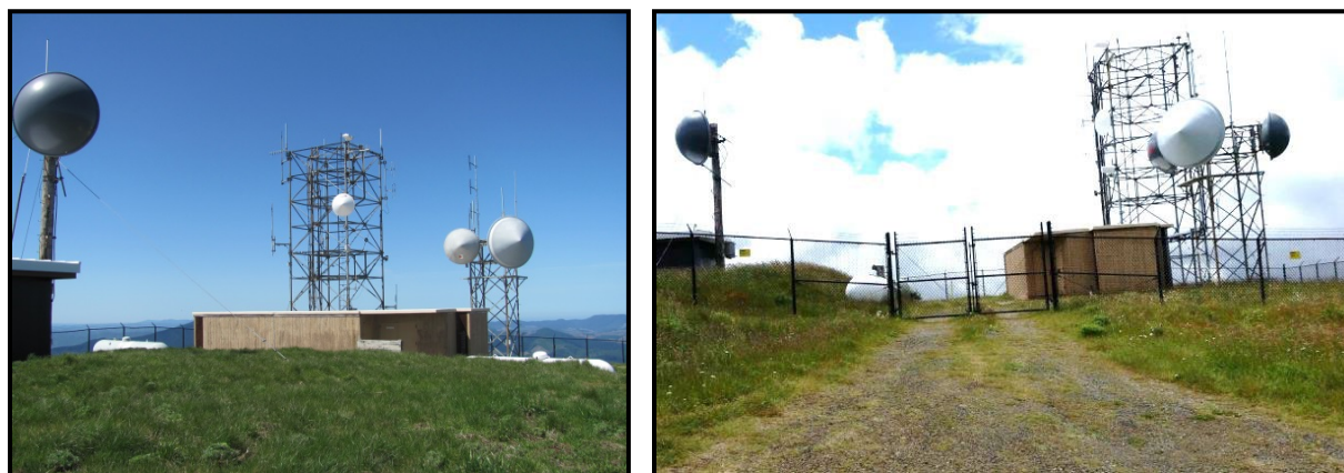
Photograph 2-9 (left). The USFS communications site (at right) and BPA communications site (left). Photograph 2-10. Double gate in north fence leading to USFS building parking area.
