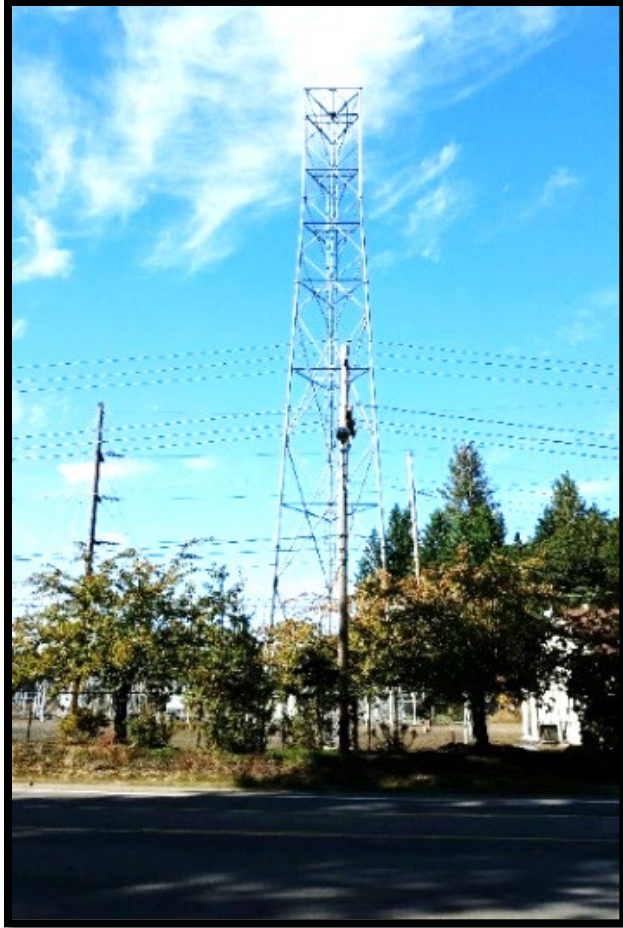
Figure F-1 (left): Mature trees and shrubby vegetation partially block the view of the Albany Substation, as seen from Orchard Lane SW at the entrance of the Chase Orchards subdivision (looking northwest).
