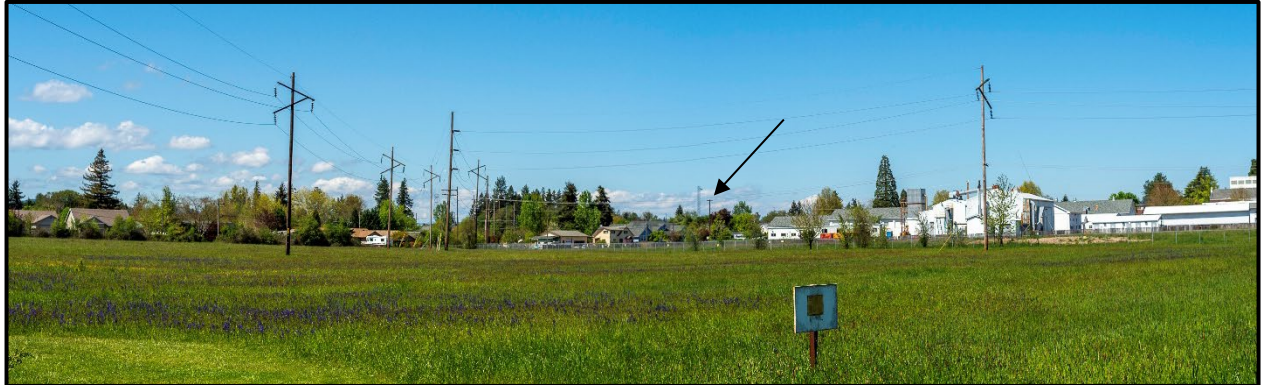
Photograph 3-31. View of the communications structure within the BPA Albany Substation from Liberty Street (KVA 16), looking west.
