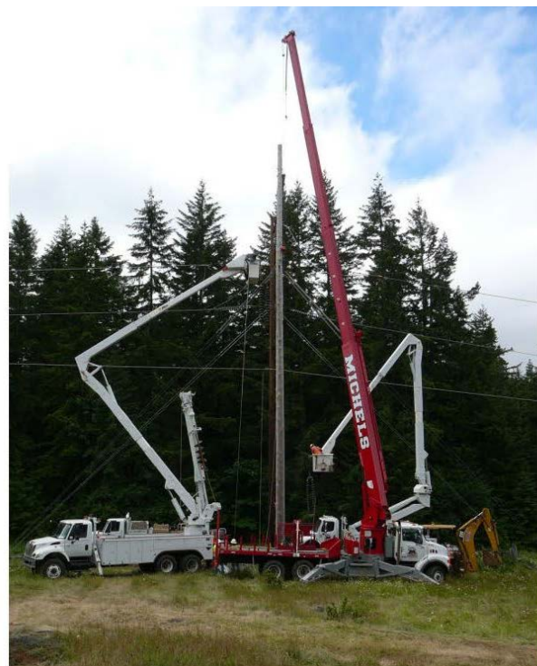
Figure 2-8. Installation of a Wood-Pole Structure
