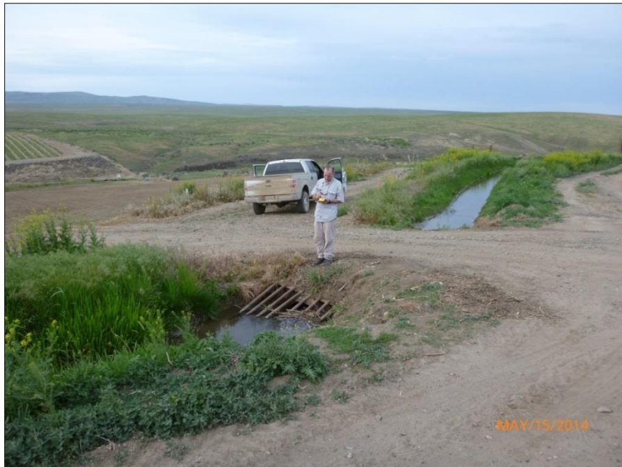
Figure 3.10-5. Photograph shows an existing culvert in an irrigation ditch between Structures 23/7 and 24/1 in Line Mile 23 that would be replaced. This ditch has been identified as a perennial waterway. (Source: Tetra Tech 2014d)
