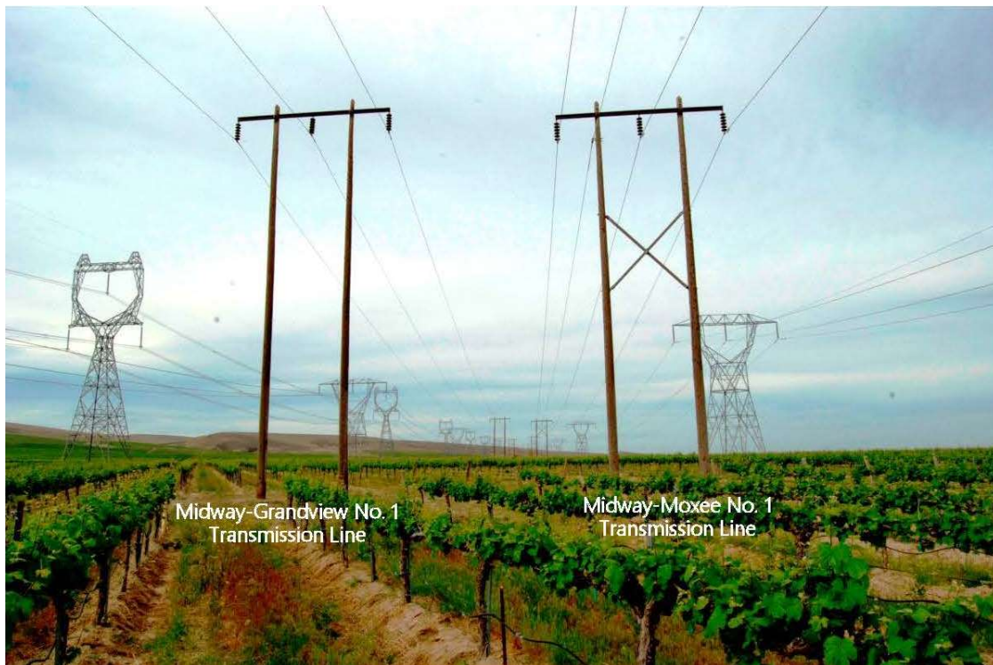
Figure 2-4. Existing Transmission Lines: Agricultural Area Near Midway-Moxee Structure 4/2 and Midway Grandview Structure 4/2
