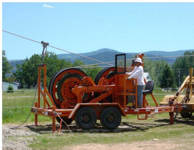
Figure 2-10. Tensioner Pulling Conductor
