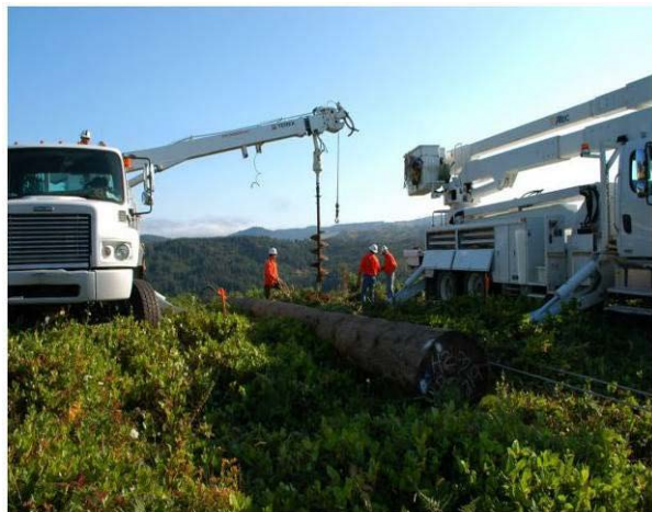
Figure 2-9. Augering a Hole for a Wood-Pole Structure
