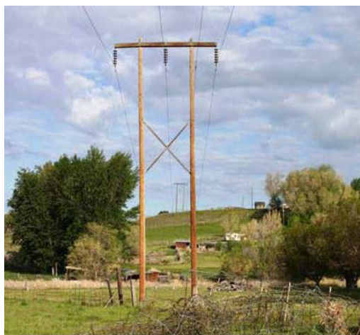
Figure 2-11. Danger Trees Near Midway-Moxee Structure 30/3
