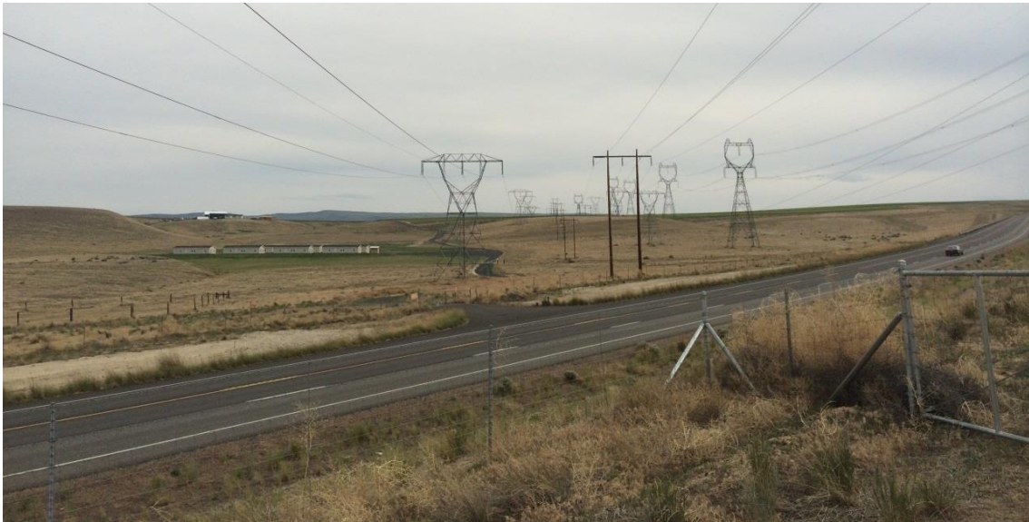
Figure 3.12-4. View of SR 24 from Midway-Grandview Line Mile 5
