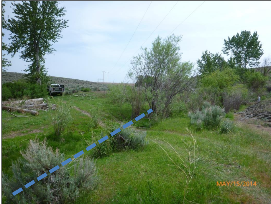
Figure 3.10-1. Photograph shows existing access road and ford in Sulphur Creek between Midway-Grandview Structures 18/7 and 19/1 in Line Mile 18 that would be improved under the Proposed Action. Sulphur Creek (location depicted by dashed line) is identified as an intermittent stream. (Source: Tetra Tech 2014d)
