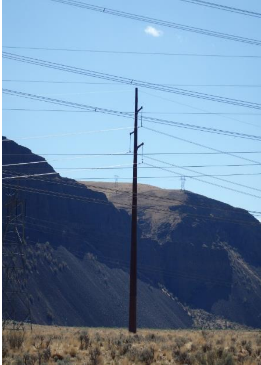
Photo 3.10-10. Recently constructed Douglas PUD transmission line with the same type of steel-pole structures that would be used for the proposed Rapids-Columbia transmission line
