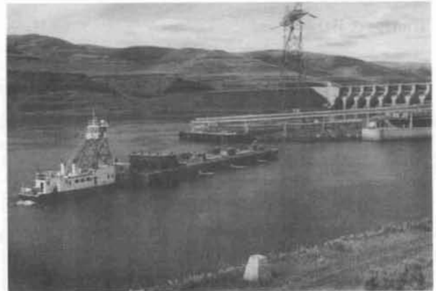
Figure 1-6. New juvenile fish transportation barge approaching new juvenile fish collection facilities at Little Goose Dam, 1990
