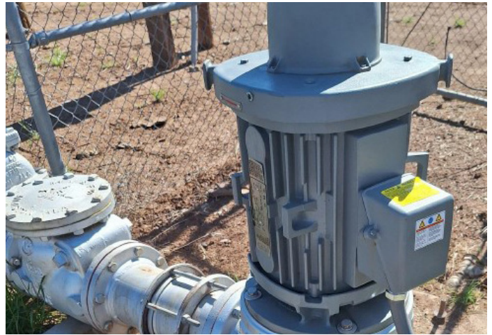
A Hudspeth pump installed in the Ochoco Irrigation District in Prineville, OR, replaced inefficient pumps with high efficiency models to save the irrigation district 51,700 kWh annually.
