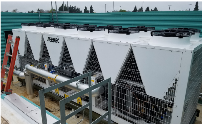
The heat pump chiller and other commercial upgrades installed at Sheldon Pool in Eugene, OR, reduced energy use by 40 percent.
