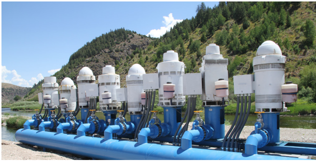
Eight new pumps installed at Schwendiman Farms.
