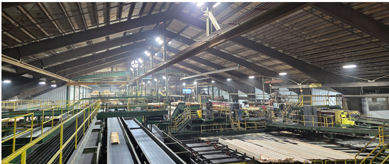
Lighting upgrades at Idaho Forest Group's LeClede sawmill.
