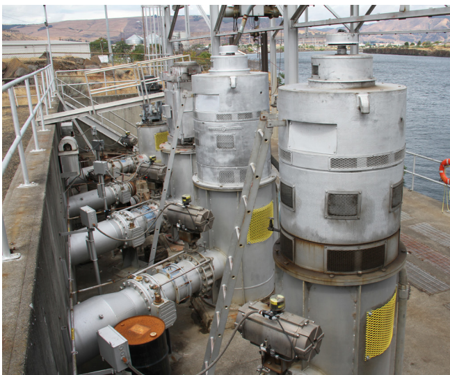
Dalles Irrigation District River Station pump upgrades.
