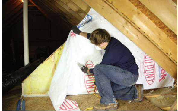
Walls in attic area: Cover new attic wall insulation with a durable, vapor-permeable air barrier to prevent air penetration of the insulation and to ensure that the insulation is held in full contact with the wall. Image courtesy of Energy Smart Academy
