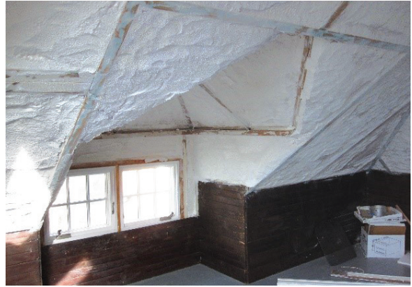
Unvented attic: Insulate the roof decking with an air-impermeable vapor barrier. Image courtesy of Neil Kelly
