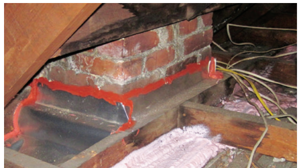
Air-sealed chimney with metal shield: Metal flashing bridges the gap between the chimney and the framing and a metal shield keeps the insulation 3 inches away from the chimney. Image courtesy of Advanced Energy
