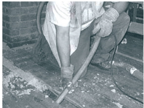
Finished attic floor: Find the large air leaks underneath the flooring and seal them before insulating the space between the joists.
