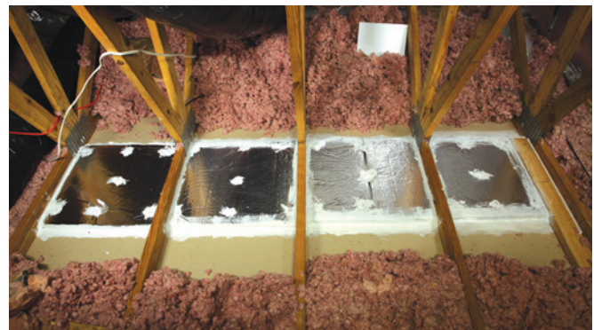
Kitchen soffits: The ventilated attic is connected to the soffit and the wall cavity through framing flaws. Any hole in the soffit creates a direct connection between the kitchen and attic. The photo shows a soffit sealed from the attic with foam board and 2-part spray foam. Image courtesy of Anthony Cox
