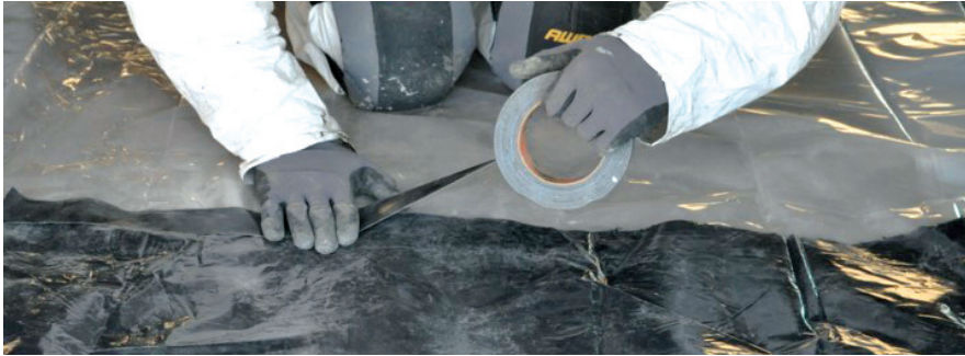
Ground moisture barrier: Ground moisture barriers prevent water vapor from saturating the air in a crawlspace.
