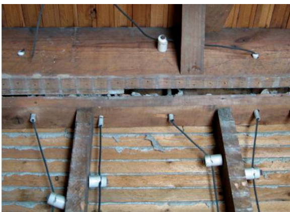
Knob and tube wiring: Obsolete and worn wiring should be replaced during energy retrofit work so that building cavities can be sufficiently insulated.
