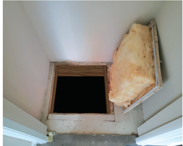
Indoor access door/hatch for underfloor areas: Weatherstrip and securely insulate all inside access doors. Image courtesy of Dan Wildenhaus
