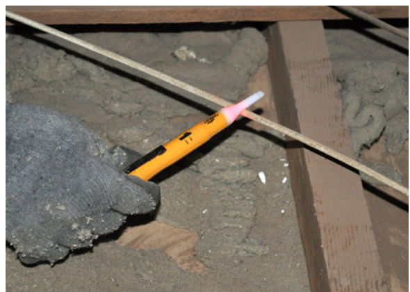
Non contact voltage tester: Test voltage wires near your work area and turn off the circuit if appropriate. Image courtesy of Energy Smart Academy
