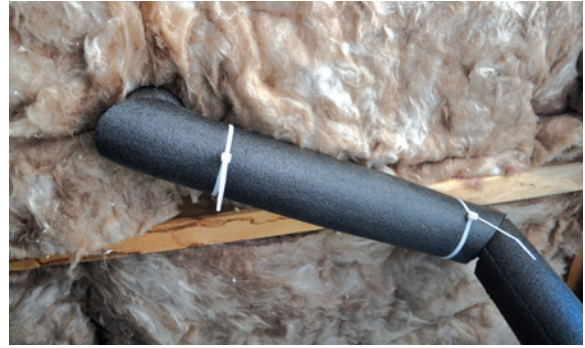
Pipe insulation: Draw bands clamp foam pipe insulation to a hot water pipe.
