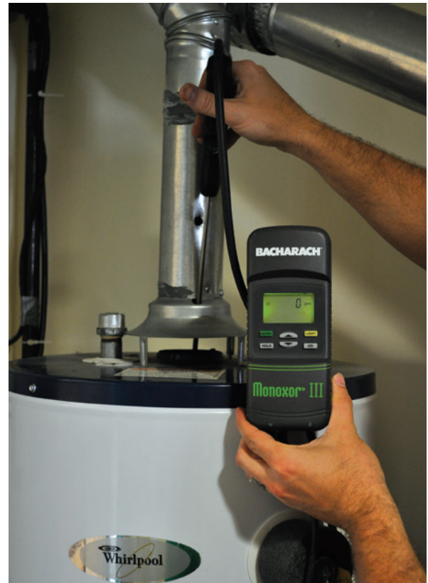
Measuring CO: Measure CO in undiluted combustion gases as they leave the heat exchanger.
