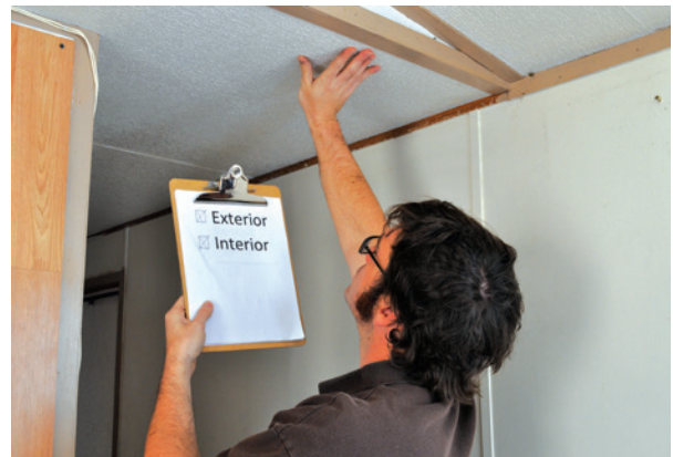
Preparing to blow a manufactured-home roof: Inspect the ceiling to be sure it can support the weight of more insulation. Image courtesy of Energy Smart Academy
