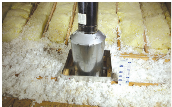
Attic insulation shield: Non-combustible material maintains 3-inch clearance around heat producing fixture and extends above insulation. Image courtesy of Advanced Energy
