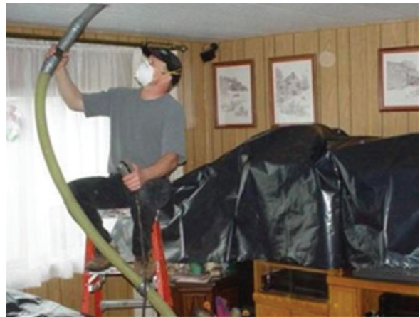
Blowing through the ceiling: The contractor pushes the fill-tube into the cavity and out near the edge of the roof. The holes are drilled in a straight line for appearance.
