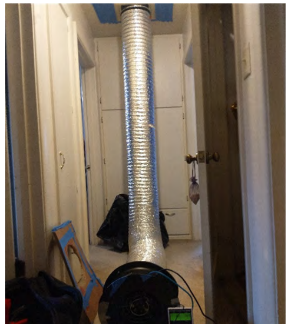
Figure 2. Duct Blaster test in progress.
