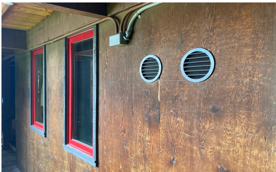
Two exterior ducts of an Ephoca heat pump unit.
