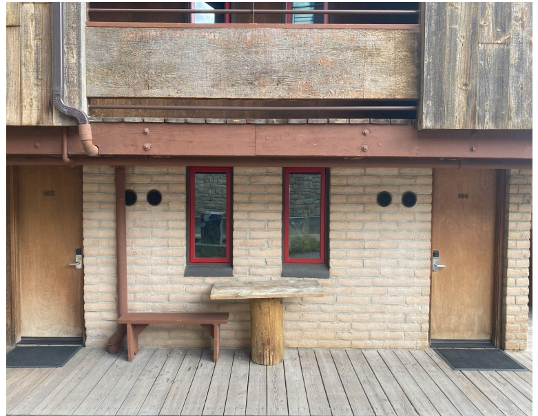
Each Ephoca appliance has two 6-inch exterior ducts.
