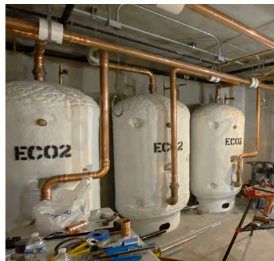
EC02 285-gallon insulated storage tanks
