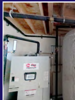
The control unit for the HPWH system
