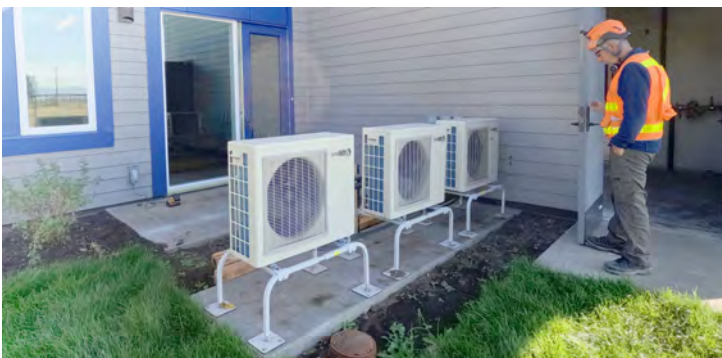
Monitoring the initial startup of the three SanCO2 heat pumps
