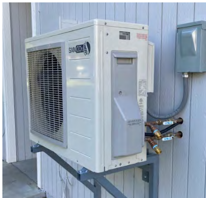
A SanC02 heat pump installed on an exterior apartment wall.
