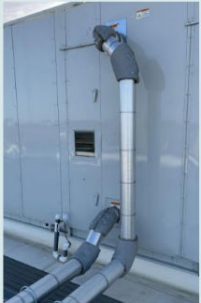
The Uranium Recovery Facility's HVAC unit with exhaust heat recovery loop.
