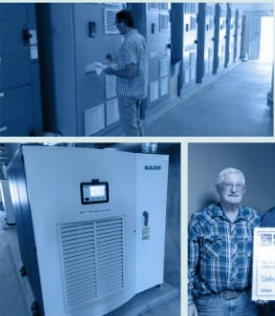
TOP LEFT: Recirculating pump VFDs. TOP RIGHT: Membrane skid. BOTTOM LEFT: One of the two installed turbo compressors. BOTTOM RIGHT: Incentive grant check ceremony image provided by the Sunnyside Sun.
