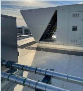
The Uranium Recovery Facility's HVAC unit with exhaust heat recovery loop.
