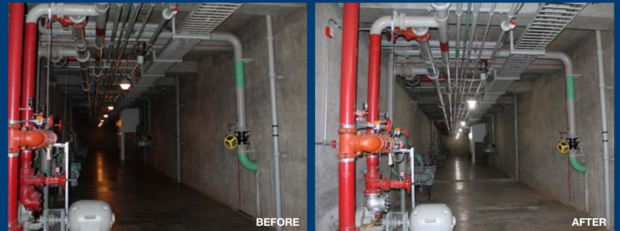
New corncob LED lights in the powerhouse pipe gallery
