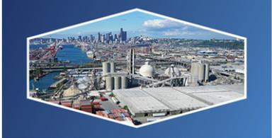
[Slide 29] Raw mill, mix products to make the cement...fairly complex process. Grinding, induction fans, cyclones separate large pieces to be re-rolled. Dust gets reheated and sent to bag house. Lots going on.
