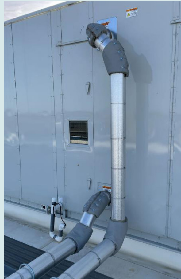
The Uranium Recovery Facility's HVAC unit with exhaust heat recovery loop.
