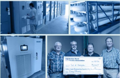
TOP LEFT: Recirculating pump VFDs. TOP RIGHT: Membrane skid. BOTTOM LEFT: One of the two installed turbo compressors. BOTTOM RIGHT: Incentive grant check ceremony image provided by the Sunnyside Sun.
