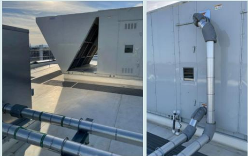
The Uranium Recovery Facility's HVAC unit with exhaust heat recovery loop.
