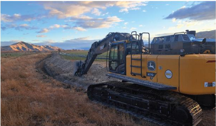
The pipeline project underway at Burnett Ditch.
