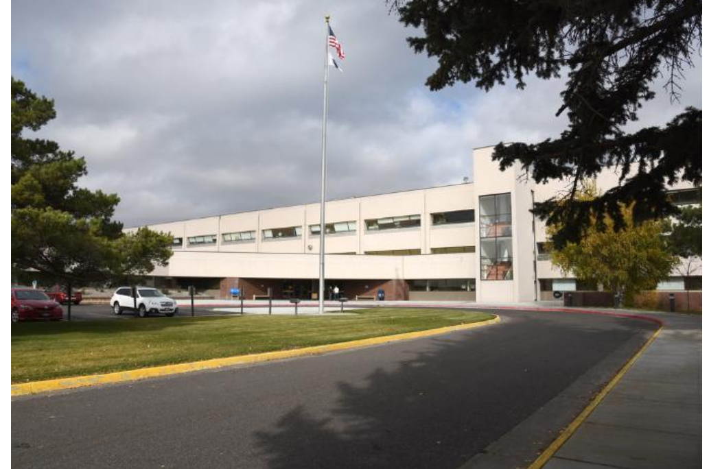
Idaho Falls Power: Idaho National Lab Willow Creek Building. 1,317,067 kWh.
