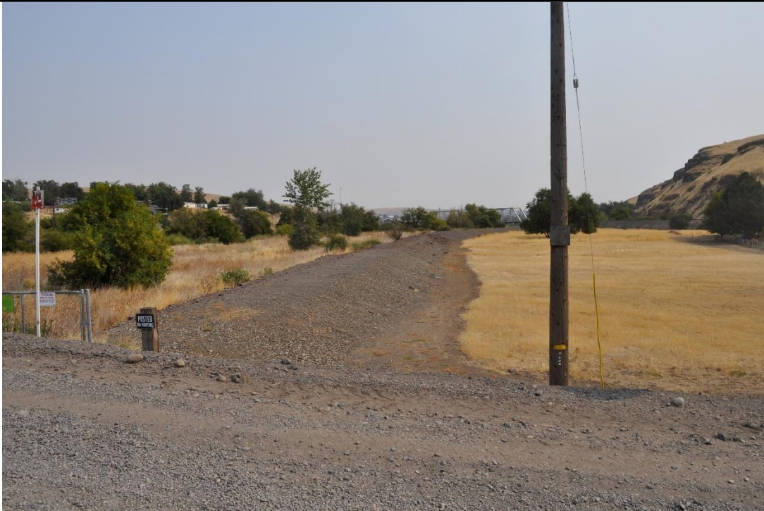
Figure 19: Top of the easternmost segment of Pendleton 2a Levee (left), looking east from Birch Creek Road (Gonzalez-Pereda, 2025).
