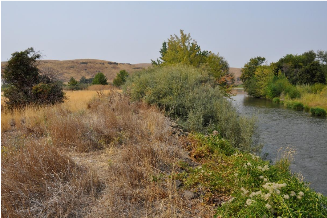
Figure 13: Middle portion of the Pendleton 2a Levee (left) along the Umatilla River (right), looking west (Gonzalez-Pereda, 2025).
