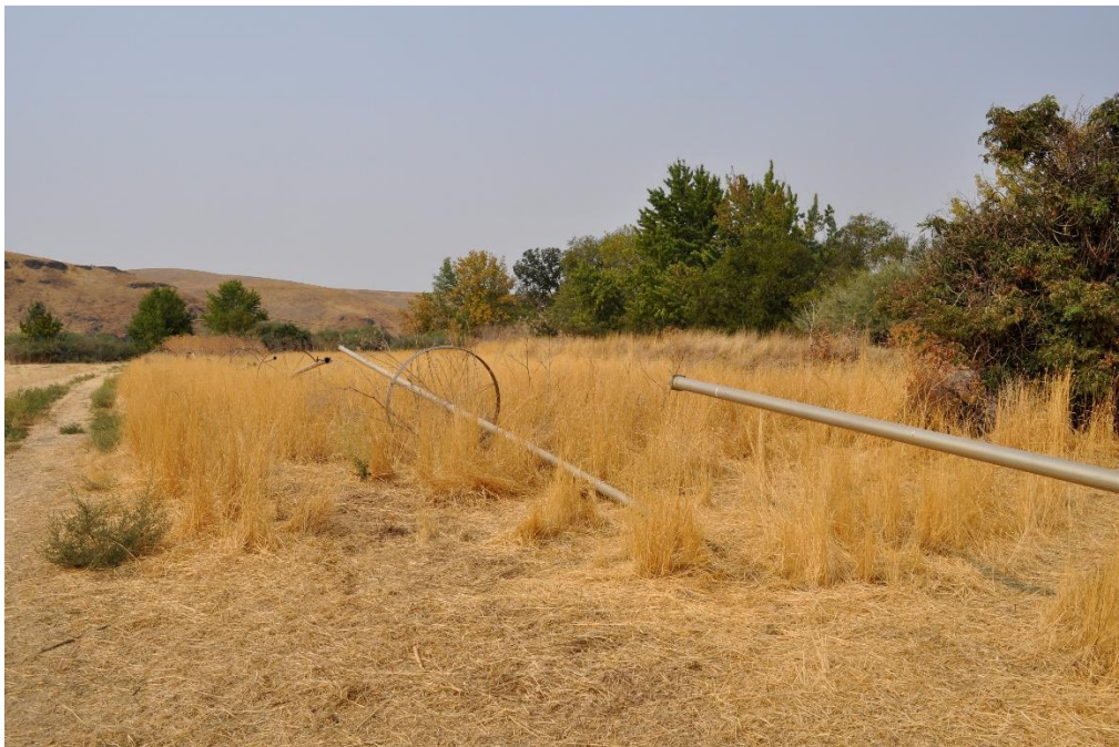
Figure 14: Top of Pendleton 2a Levee (right), looking west (Gonzalez-Pereda, 2025).
