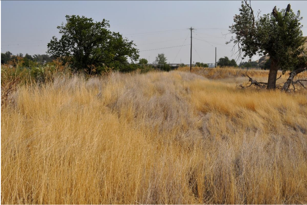
Figure 17: Pendleton 2a Levee (left), looking east toward Birch Creek Road (Gonzalez-Pereda, 2025).
