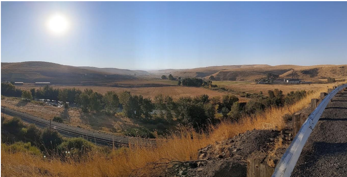
Figure 6: Panorama view of Pendleton 2a Levee, looking south (Duran, 2022).
