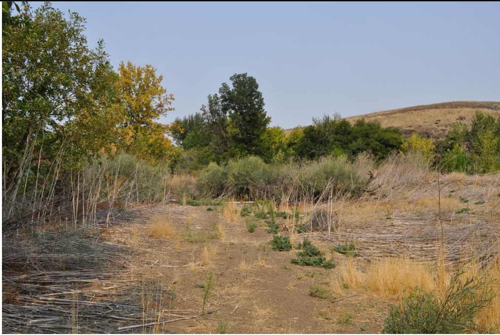
Figure 15: Top of Pendleton 2a Levee, looking east (Gonzalez-Pereda, 2025).
