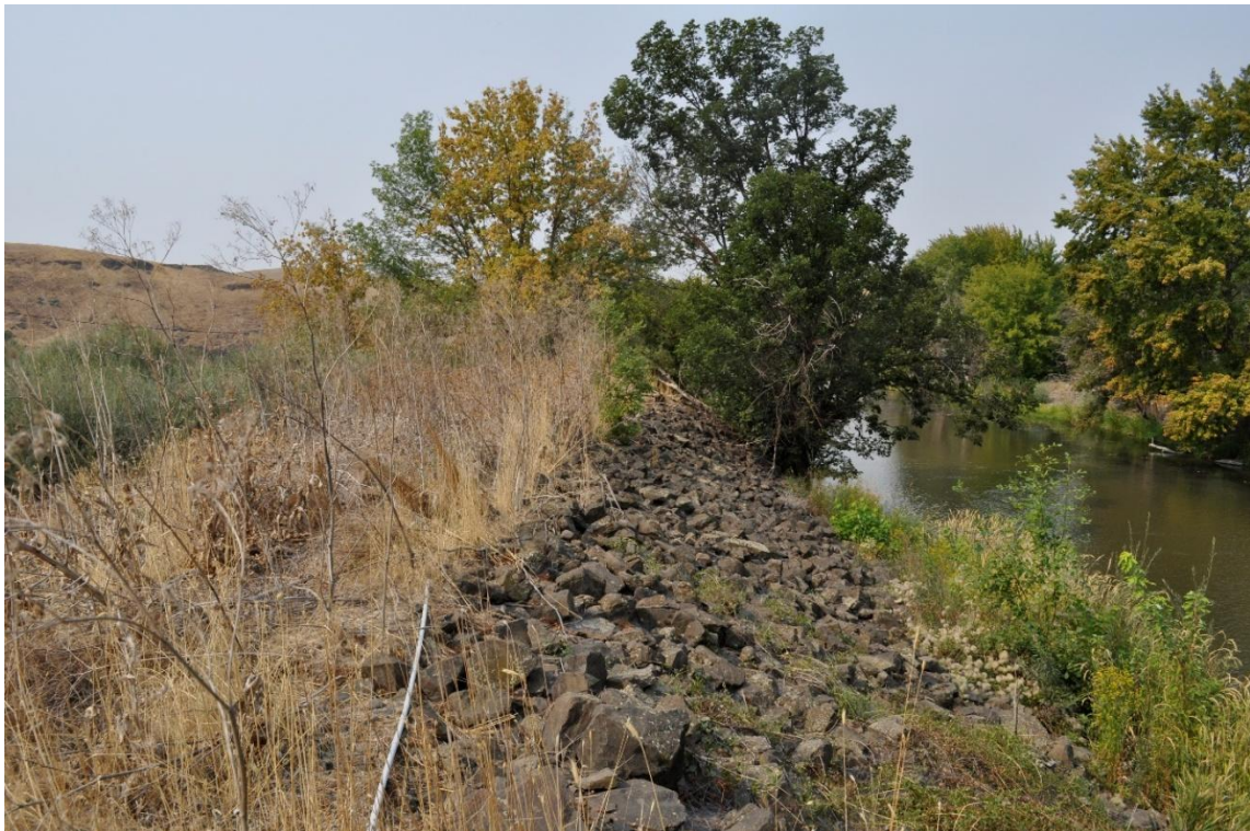
Figure 12: Example of riprap found along the length of the Pendleton 2a Levee, looking west (Gonzalez-Pereda, 2025).
