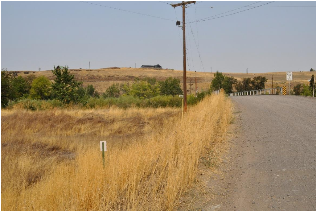
Figure 18: Birch Creek Road crossing over the Pendleton 2a levee, looking north (Gonzalez-Pereda, 2025)
