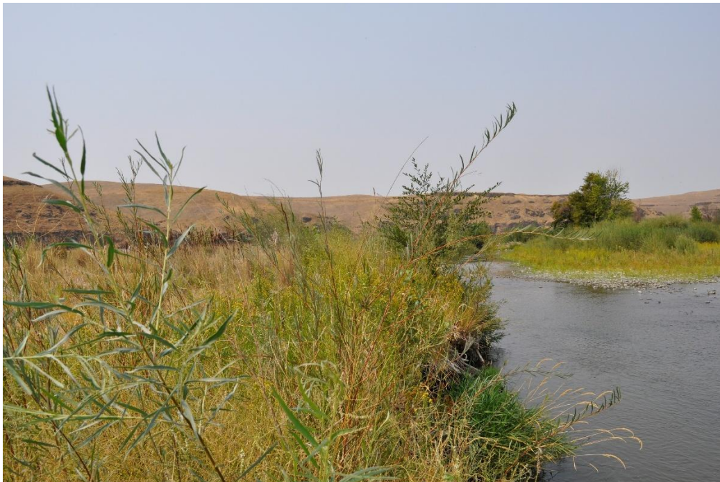
Figure 10: Western most portion of the Pendleton 2a Levee (left), looking west (Gonzalez-Pereda, 2025).
