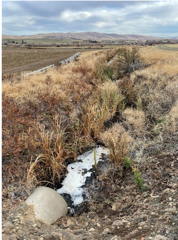
Figure 15: Overview of Purdin Ditch, looking south (Schiffman, 2024)
