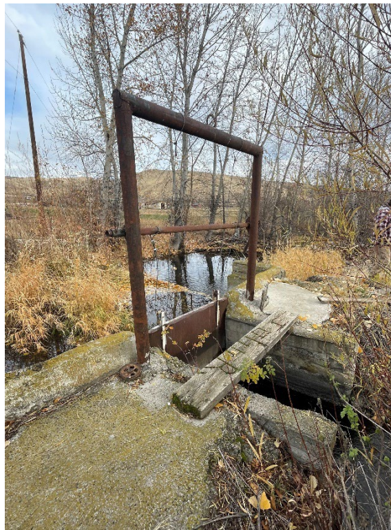
Figure 6: Metal headgate, looking northeast (Schiffman, 2024)
