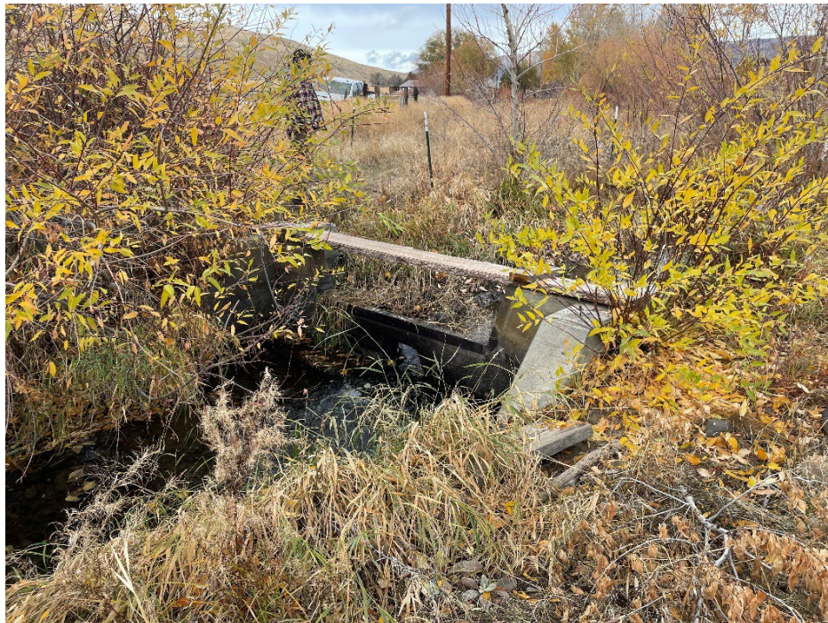
Figure 10: Concrete drop structure, looking north (Schiffman, 2024)
