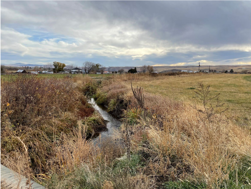
Figure 13: Overview of Purdin Ditch where it crosses Jenkins Road, looking south (Schiffman, 2024)
