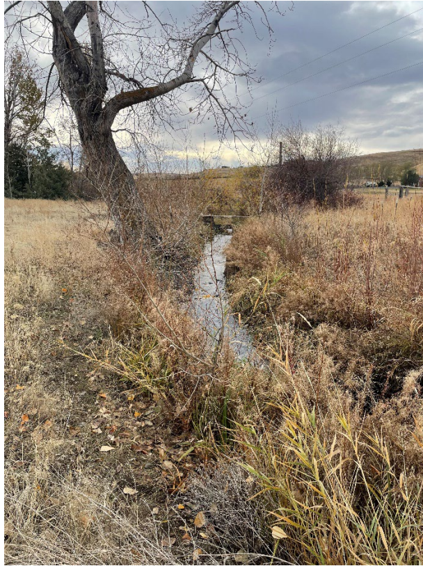
Figure 9: Purdin Ditch, looking south towards drop structure (Schiffman, 2024)
