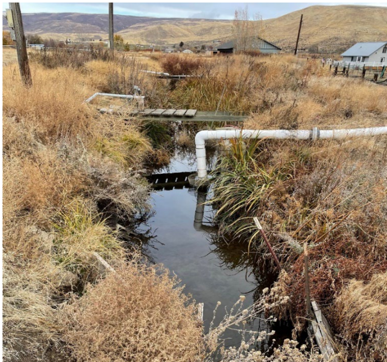
Figure 12: PVC pipes connected to pumps that deliver water from Purdin Ditch to landowners properties, looking north (Schiffman, 2024)
