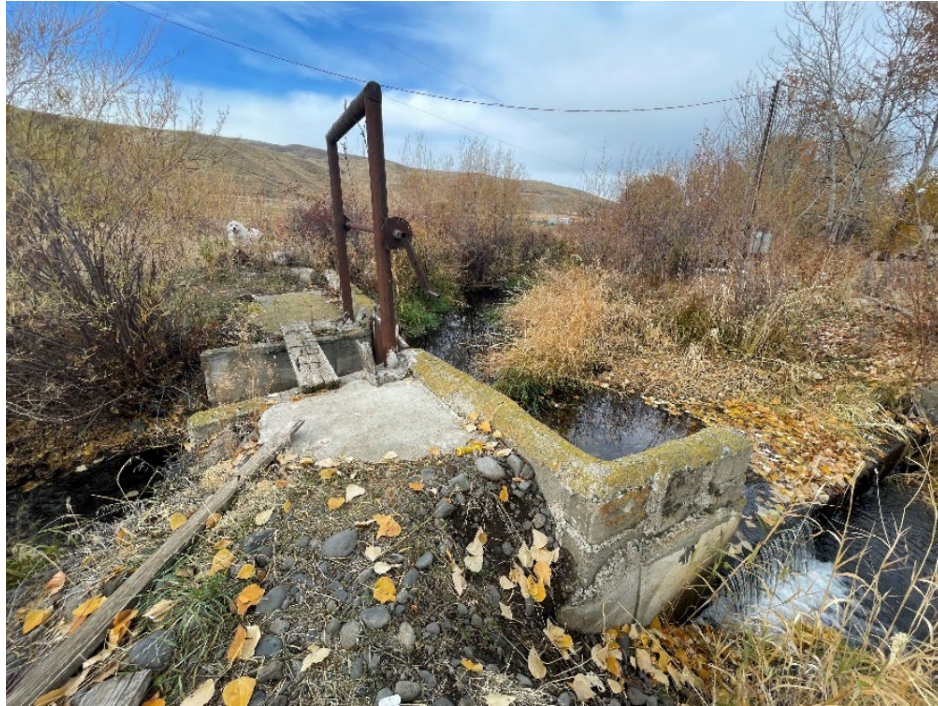
Figure 5: Metal headgate and drop dam where water is diverted from Dry Creek, looking northwest (Schiffman, 2024)
