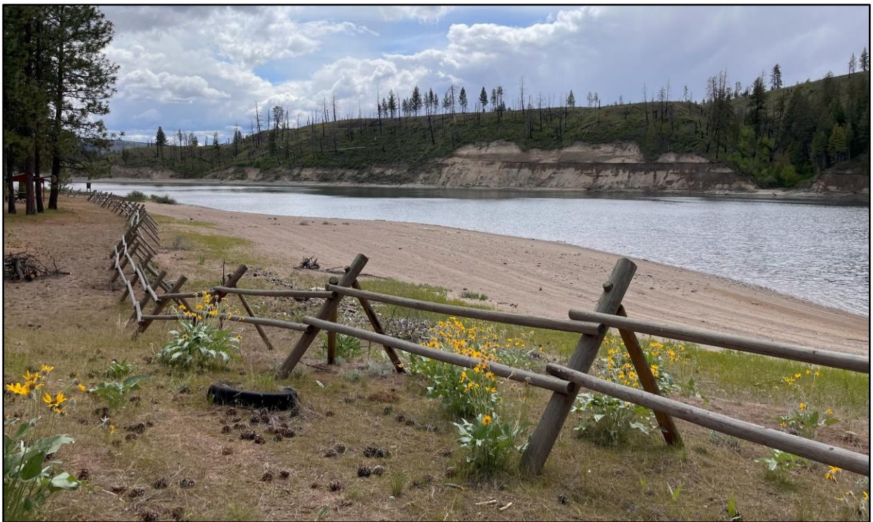
Figure K-8. Buck and pole fencing treatment in the Spokane Arm APE.
