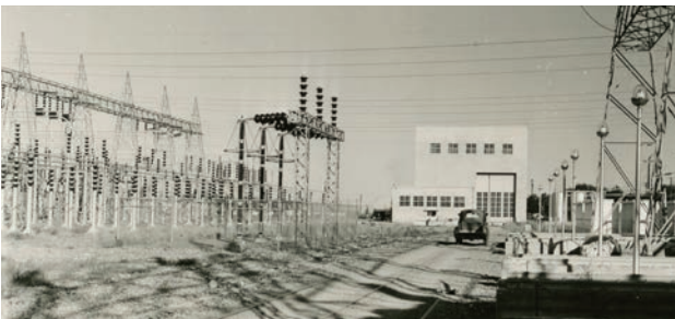
Tier I: Midway Substation. Historic photo.
