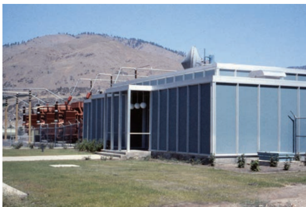
Sickler Substation in 1970. Historic photo.
