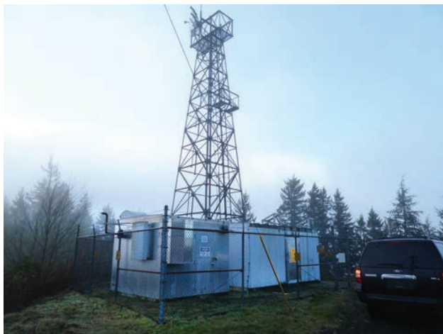
Tier II: Goodwin Peak Microwave Radio Station (1953) near Mapleton, Oregon, is significant in the area of Communications as a key component of BPA's early microwave communications network. It is also significant in the area of Industry for supporting regional industrial development. All National Register of Historic Places-eligible microwave radio stations are Tier II resources.
