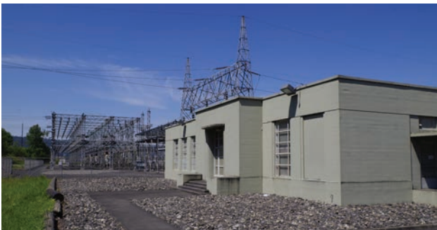
Streamline Moderne control house at St. Johns Substation in Portland, Oregon.
