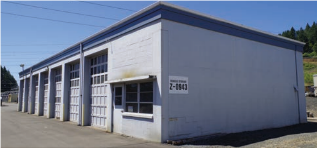
Automotive Shop (built 1953) at Alvey Substation and Maintenance Headquarters.
