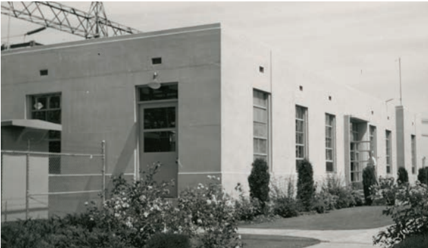
Alcoa Substation Control House. Historic photo.
