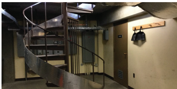
Modern circular stairwell. Hanford Substation Control House (1970)
