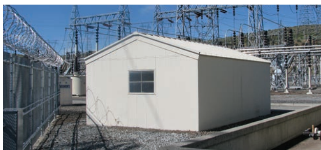
Oil house (presently storage) at Chief Joseph Substation (1958) in Bridgeport, Washington.
