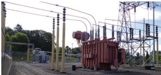
The transfer track at Salem Substation (1942) is mostly obscured by switchyard gravel.
