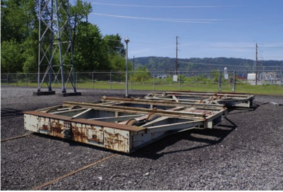
Transfer Cart for moving heavy equipment on transfer tracks in a switchyard.
