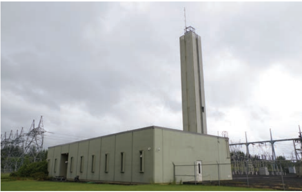
Control house at Alston Substation (1969).
