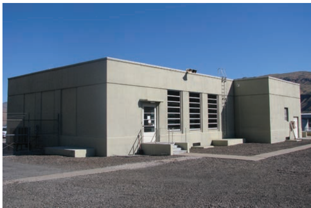
Streamline Moderne control house at Valhalla Substation (1953) in Malaga, Washington.
