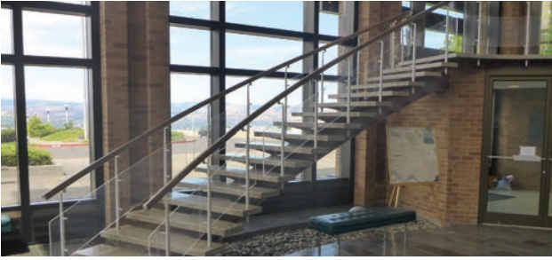
Cello Converter Station Control House (1970).
