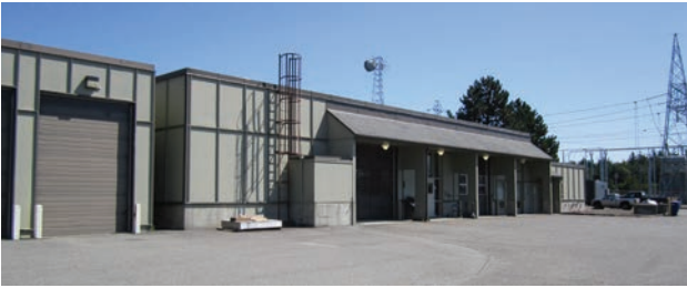
Maintenance building at Custer Substation (1967) in Ferndale, Washington. Overall the Custer Substation is not eligible for the National Register of Historic Places, due to alterations to the control house; although the maintenance building retains integrity.
