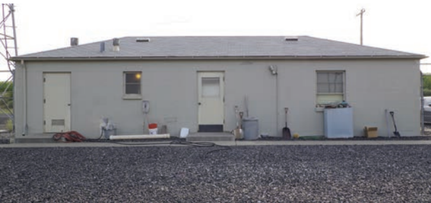
Grandview Substation Control House (1954), in Grandview, Washington, reflects the Minimal Traditional style, characterized by its lack of architectural ornament. BPA employed this style for certain control house from the 1940s to 1960s.
