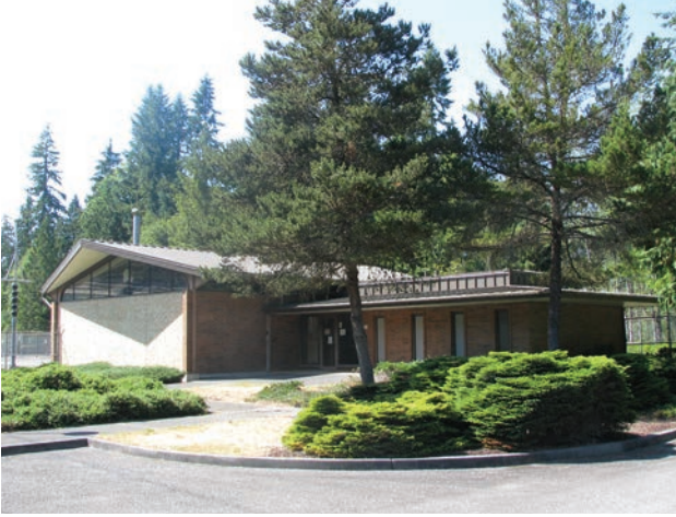
Tier I: Murray Substation Control House (1972) in Arlington, Washington is an example of the Contemporary architectural style and Beauty design concepts deployed by BPA during the System Expansion Period.
