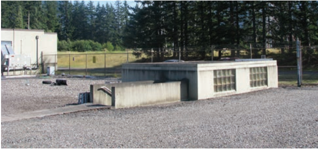
North Bonneville Substation Oil House (built 1940).
