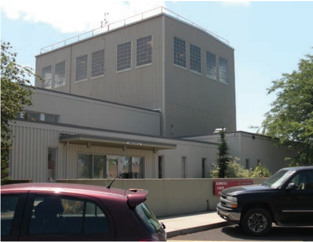
Spokane District and East Regional Headquarters Building at Bell Substation (1942) in Mead, Washington. This building, and the Bell Substation overall, are not eligible for the National Register of Historic Places due to alterations.
