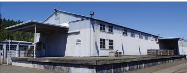
Maintenance building (built 1952) at Alvey Substation and Maintenance Headquarters.
