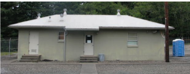
Minimal Traditional control house at Tahkenitch Substation (1963) near Gardiner, Oregon.
