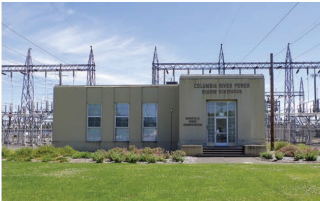
Eugene Substation (1940) in Eugene, Oregon, was built during BPA's Master Grid Period as the terminus for the Vancouver-Eugene transmission line. The 115 kV line served the City of Eugene and its vicinity. The Eugene Substation Control House, built in the Streamline Moderne architectural style, is the only remaining example of its type (BPA Type 100) in the BPA system.
