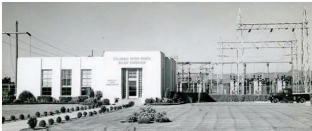
The Eugene Substation Control House's character-defining features are its single-story, concrete construction; flat roof with parapet; curved walls at main entrance; curved metal railing; and original brass signage above and adjacent to the main entrance. Historic photo.
