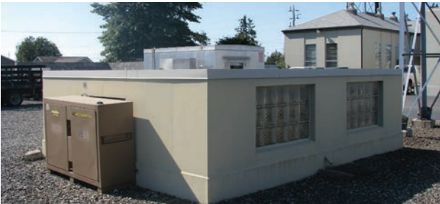
Oil house at Port Angeles Substation (1950) in Port Angeles, Washington.
