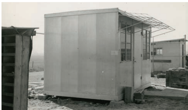
Tier III: Lookingglass Substation Control House. Historic photo.
