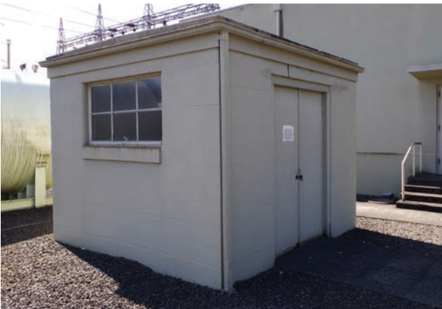
Oregon City Substation (1943) with 1953 pump house.
