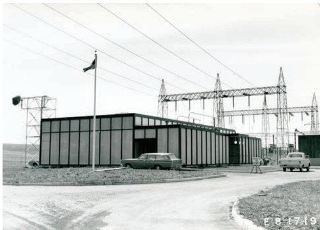
John Day Substation (1966), near Rufus, Oregon, is associated with the Pacific Northwest–Southwest Intertie and part of the first 500 kV transmission subsystem to serve the Portland area.
