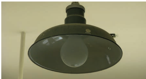
Utilitarian light fixture. Midway Untanking Tower (1941)
