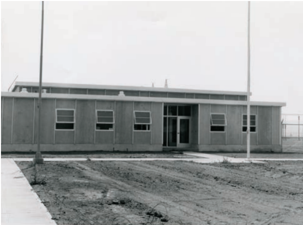
Lane Substation Control House during construction.
