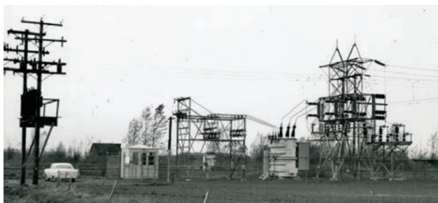
Tier III: Harrisburg Substation in 1963. Historic photo.
