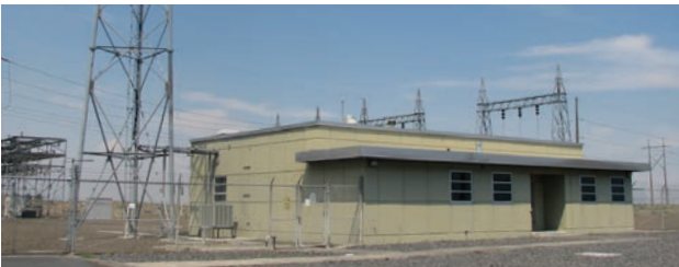
Potholes Substation Control House (1958).
