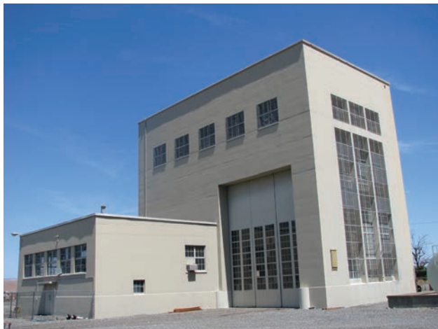
Tall, concrete untanking tower at Midway Substation (1941) built in the Streamline Moderne style.
