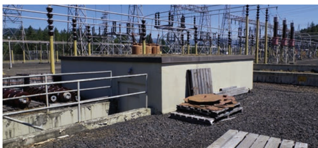
Although Utilitarian oil houses generally have steel-frame construction, some, such as the oil house at Santiam Substation (1954) near Stayton, Oregon, have concrete construction.
