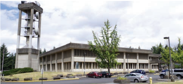
Dittmer Control Center (1974).
