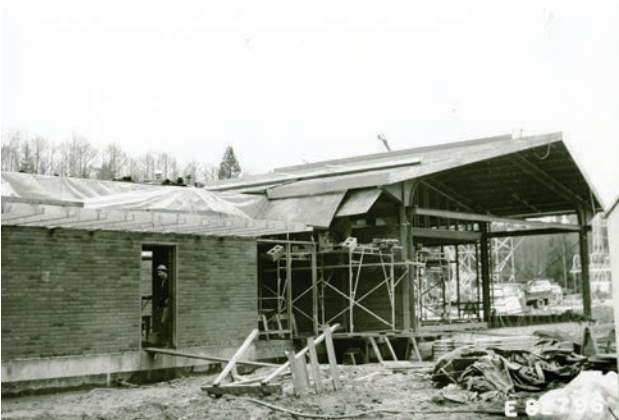
Tier I: Murray Substation Control House under construction in 1971. Historic photo.
