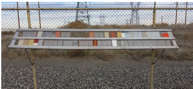
Paint Test Panel at Franklin Substation.
