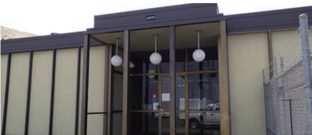
Modern style globe lights at John Day Control House entrance.
