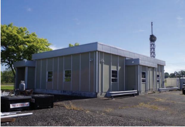
Lane Substation Control House (1967) in Eugene, Oregon, was designed by BPA architect C. Tetherow with features of the International S style of architecture. The substation was a terminus of the Marion–Lane transmission line, a 72-mile, 500 kv line that served customers in Eugene.
