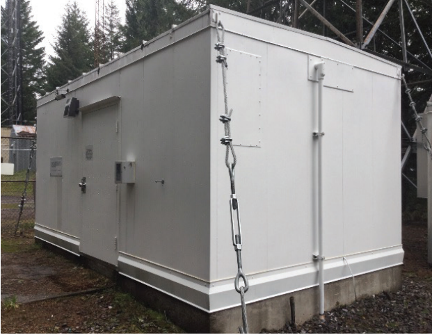
Noti Microwave Radio Station building (1954).
