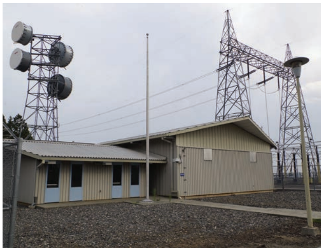
Dworshak Substation (1972) was built near the end of the System Expansion Period. The substation contains a historic control house, maintenance building, engine generator building, and switchyard, all of which contribute to the Dworshak Substation historic district.
