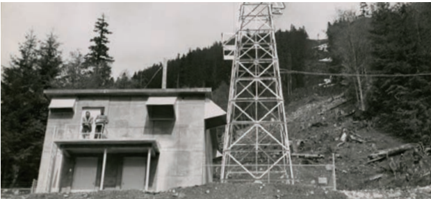
Rockdale Microwave Radio Station (1955) with ladder enabling entry at second story during deep snowfall events. Historic photo.
