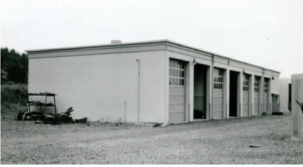
Alvey Automotive Shop (1953) is one of the substation's historic buildings. Formerly called Goshen Substation, Alvey Substation's other historic buildings include the maintenance, Engine Generator, Automotive Storage, and Customer Service Engineering buildings, all of which contribute to the historic district. Historic photo.
