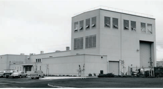
Bell Substation (1942) was built in Mead, Washington, to help meet the increasing power demands of war industries, particularly aluminum. Bell Substation's numerous changes render it "not eligible" for the National Register of Historic Places. However, the substation's tall untanking tower is still important as a rare BPA building type.
