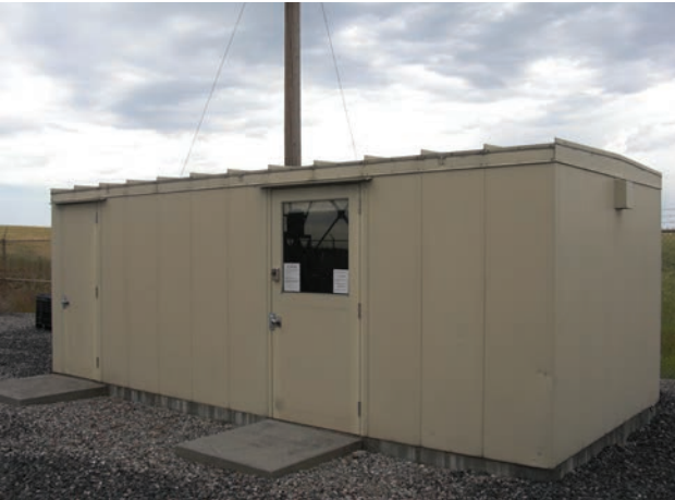
Wagner Lake Substation Control House (1974), in Wilbur, Washington, is one of the many control houses assembled at BPA substations in the 1960s and 1970s that consisted of prefabricated, aluminum-panel construction. The substation is historically significant for its association with BPA's rural electrification efforts
