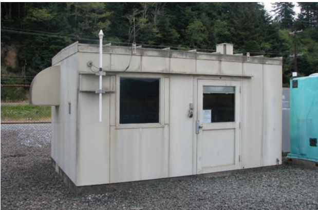
Tier I: Gardiner Substation Control House (1963) in Gardiner, Oregon, retains excellent architectural integrity as an example of BPA's Standard Aluminum Control House Type 193 design and is historically significant in the area of Government for its association with rural electrification.
