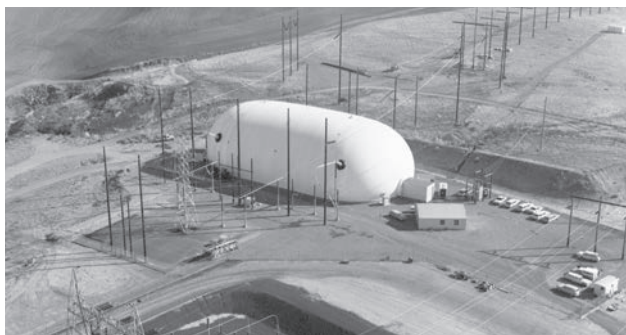
HVDC Test Center at Big Eddy. The Test Center was used until 1996 and was removed in 2018.
