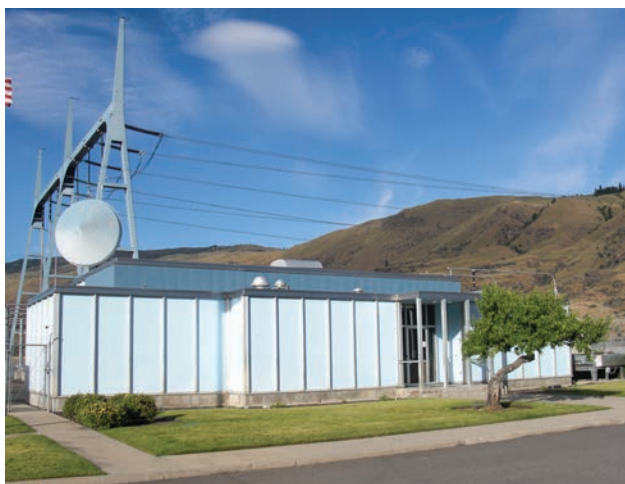
Sickler Substation (1969) was built in East Wenatchee, Washington, during BPA's System Expansion Period (1946–1974) and is part of BPA's 500 kV transmission subsystem. The substation's control house is significant in the area of Architecture for its International design and adherence to BPA's beauty principles.
