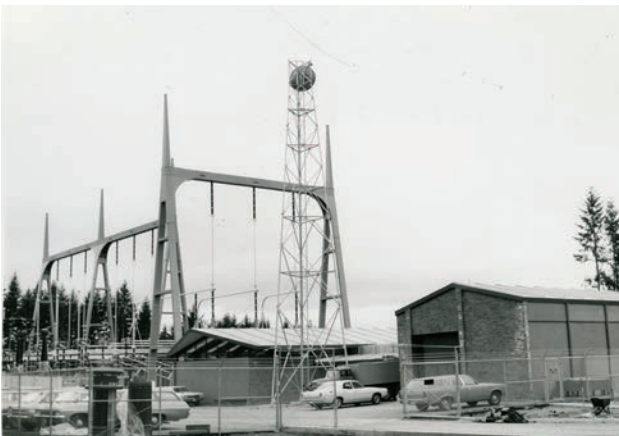
C.W. Paul Substation (1971). Historic photo.
