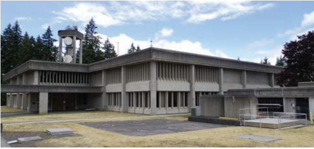
William A. Dittmer Control Center (1974) at Ross Substation in Vancouver, Washington.
