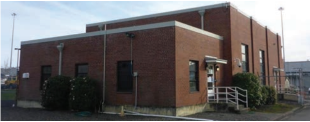
Brick-clad control house at Troutdale Substation (1943) in Troutdale, Oregon.
