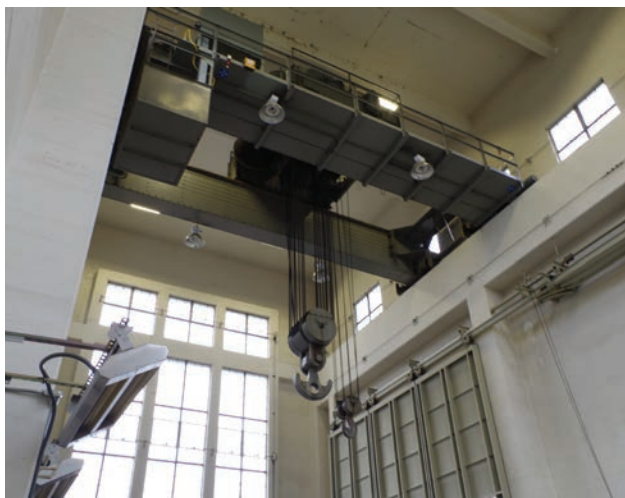
Untanking tower crane at Chehalis Substation (1941).
