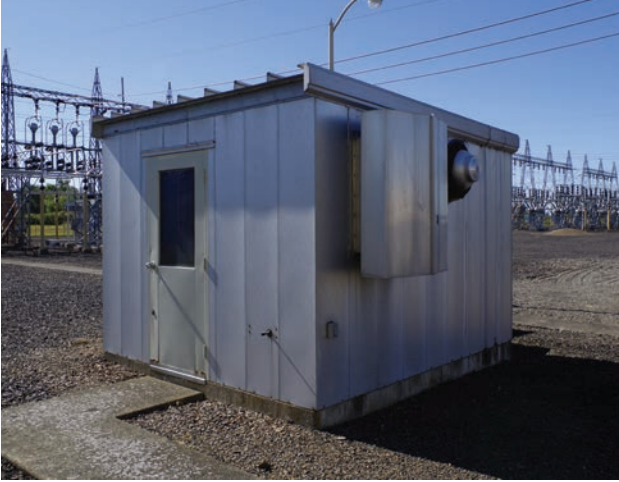
Engine generator building constructed in 1963 at Chemawa Substation (1954) in Keizer, Oregon.
