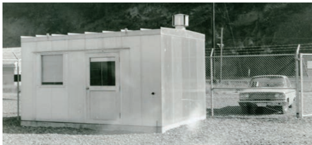
Tier I: Gardiner Substation Control House in 1964. Historic photo.
