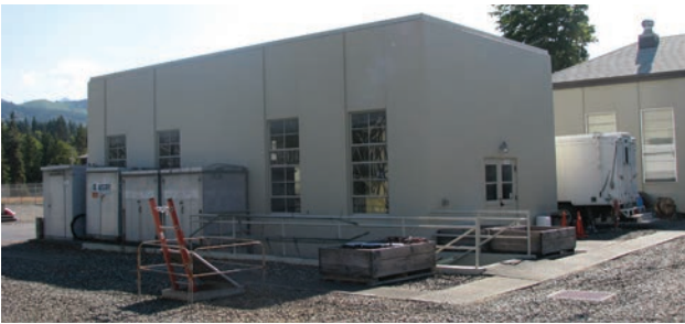
Maintenance building (built 1950) at Port Angeles Substation and Maintenance Headquarters.
