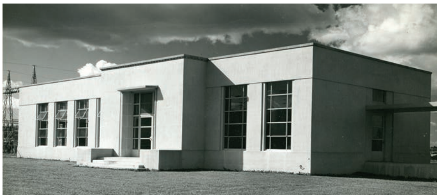
Historic photo, control house.
