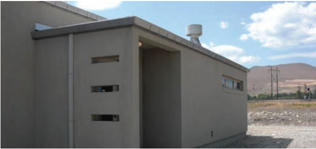
Anaconda Substation Control House (1950).
