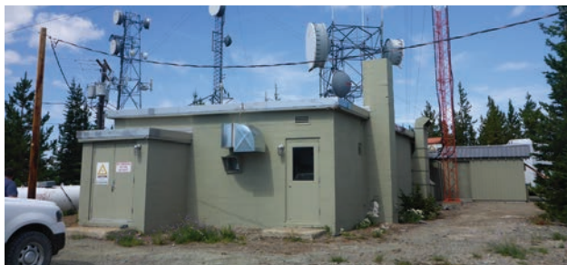
Blacktail Peak Microwave Radio Station (1968) contains a historic station building (shown in foreground) and microwave antenna towers.
