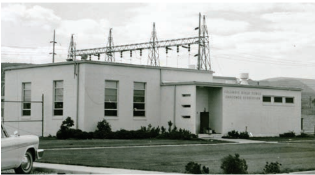
The Anaconda Substation (1953) was built to power the Anaconda Aluminum Company plant in Montana. The substation was part of BPA's expansion into Montana and contributed to midcentury development of the Pacific Northwest's aluminum industry. The control house is architecturally significant for its modern industrial design.
