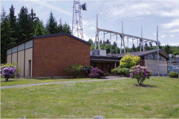
Modern/Contemporary Control House and maintenance building at C.W. Paul Substation (1971) in Centralia, Washington.
