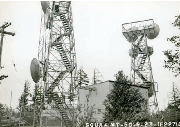
BPA pioneered midcentury microwave technology. Microwave radio station site locations were selected to enable associated stations and equipment to maintain their "line of sight," a key element of microwave communication technology. BPA's microwave radio station sites that retain and use their original station buildings and antenna towers, such as Squak Mountain Microwave Radio Station (1950), are historically significant. Historic photo.
