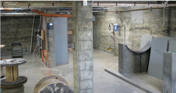
Board form concrete construction visible in basement interior.
