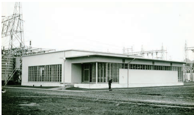
Alvey Substation and Maintenance Headquarters (1952) near Eugene, Oregon, is part of BPA's System Expansion Period. The Tier I control house was built in the International style of architecture and is the only example of its type (BPA Type 180) in the BPA system.
