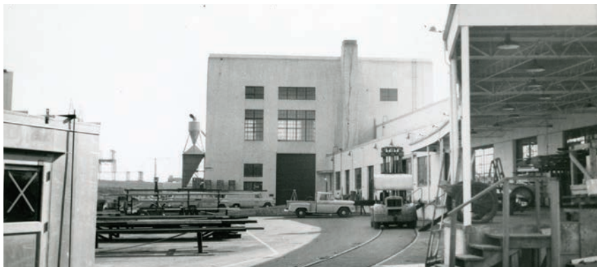
Historic photo, control house.
