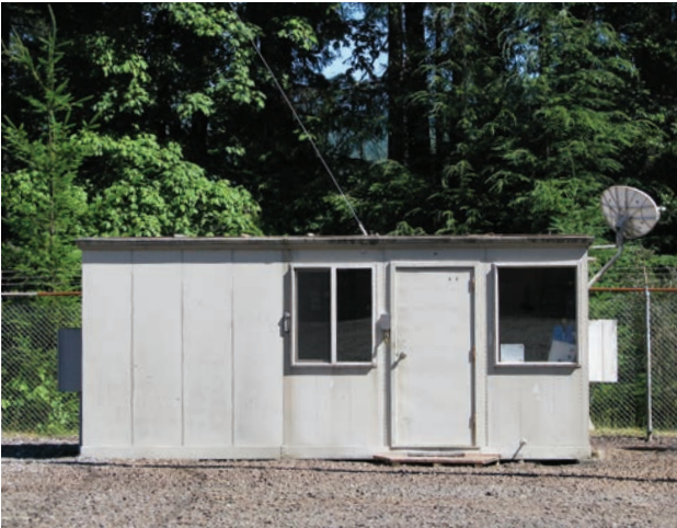
Utilitarian control house at Mapleton Substation (1948) in Oregon.
