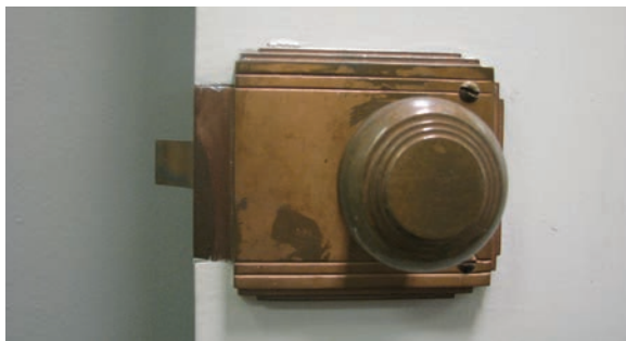
Streamline Moderne door hardware common at Master Grid and early System Expansion substations.
