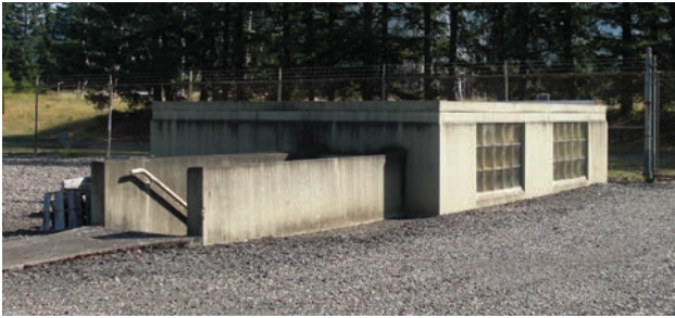
The North Bonneville Substation (1941) in Washington was built during BPA's Master Grid Period (1938–1945). The substation's oil house is a small, semi-subterranean building that reflects features of the Streamline Moderne architectural style.
