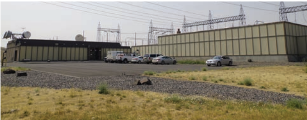
International-style control house and maintenance building at John Day Substation (1968).
