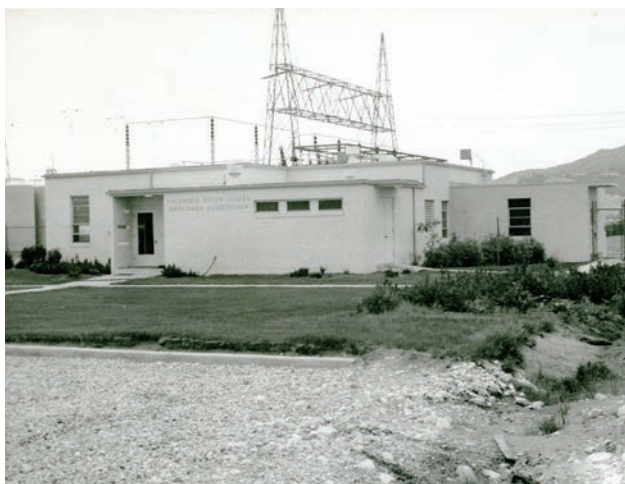
Anaconda Substation Control House (1950). Historic photo.
