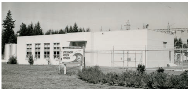
Tier II: Oregon City Substation. Historic photo.
