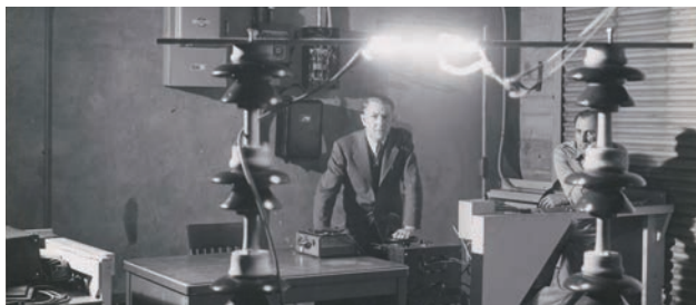
J.D. Ross Substation (Ross Complex) High Voltage Test Laboratory, c. 1946. Historic photo.
