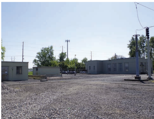
St. Johns Substation (1940) was built during the Master Grid Period with an oil house, storage building, and control house as well as rails and a cart.
