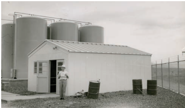
Tier II: Chief Joseph Substation, oil house and tanks in 1971. Historic photo.
