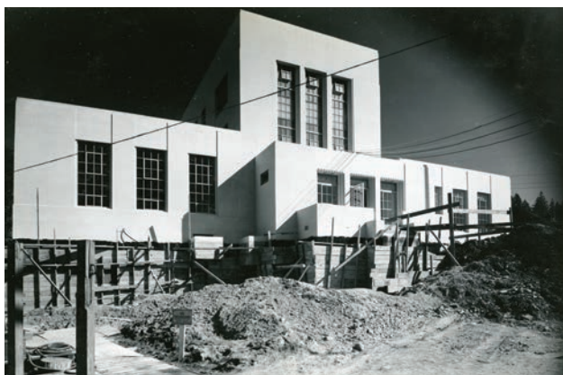
Salem Substation (1942) under construction. The untanking tower, which forms the control house's central block, is flanked by two one-story wings. Historic photo.
