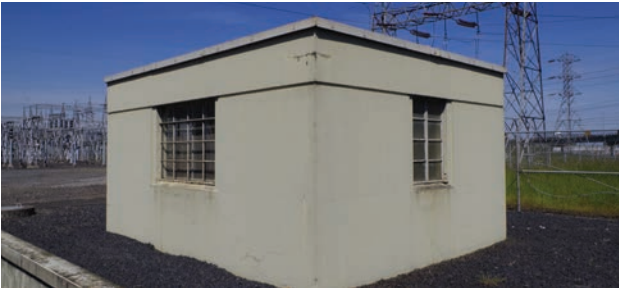
St. Johns Substation Oil House (1940).
