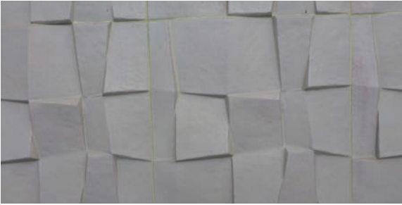
Modern cast stone interior wall panels.
