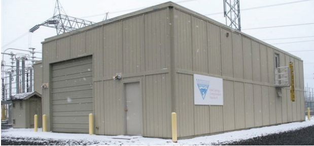
Sand Spring Compensation Station Control House (1969).
