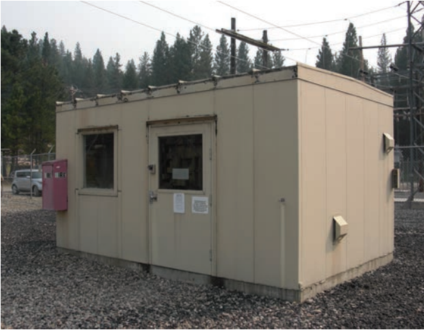
Republic Substation (1953) in Washington is significant in the area of Politics/Government for providing reliable power to the local Ferry County public utility district for distribution to rural communities in eastern Washington.
