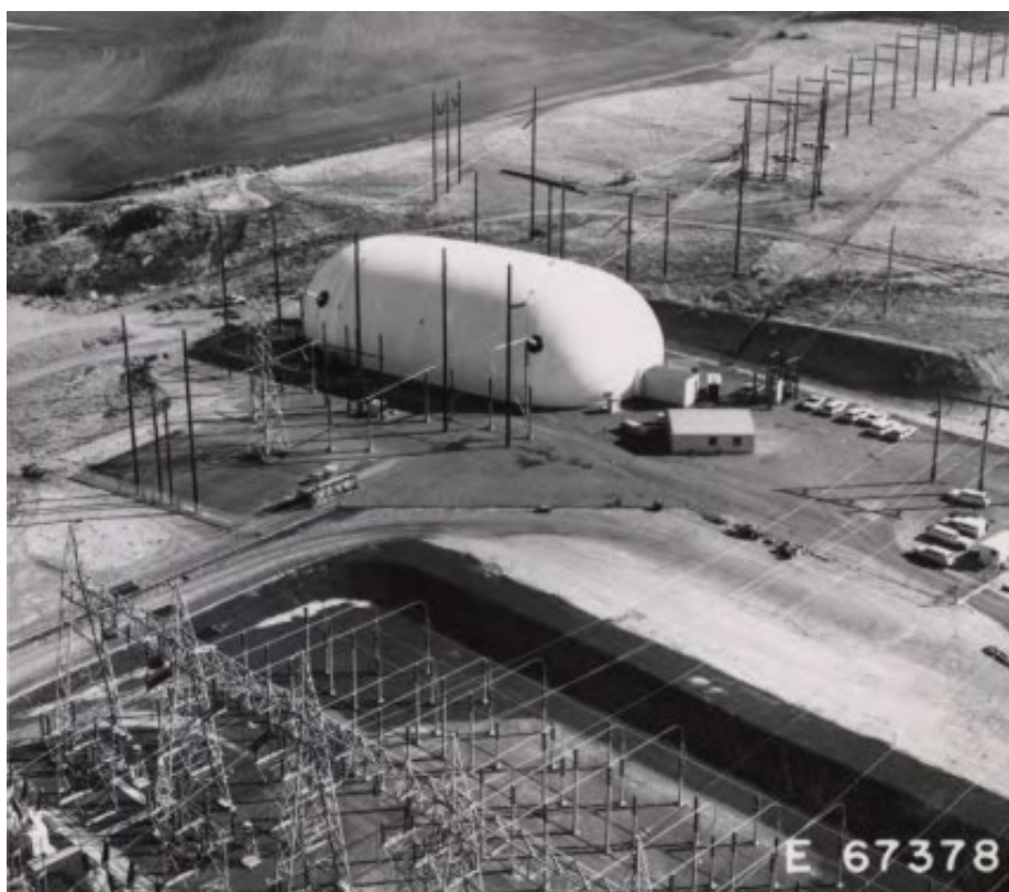
Figure 24. Photograph of the original air bubble and greater facilities at the HVDC Test Center, 1963. 146
