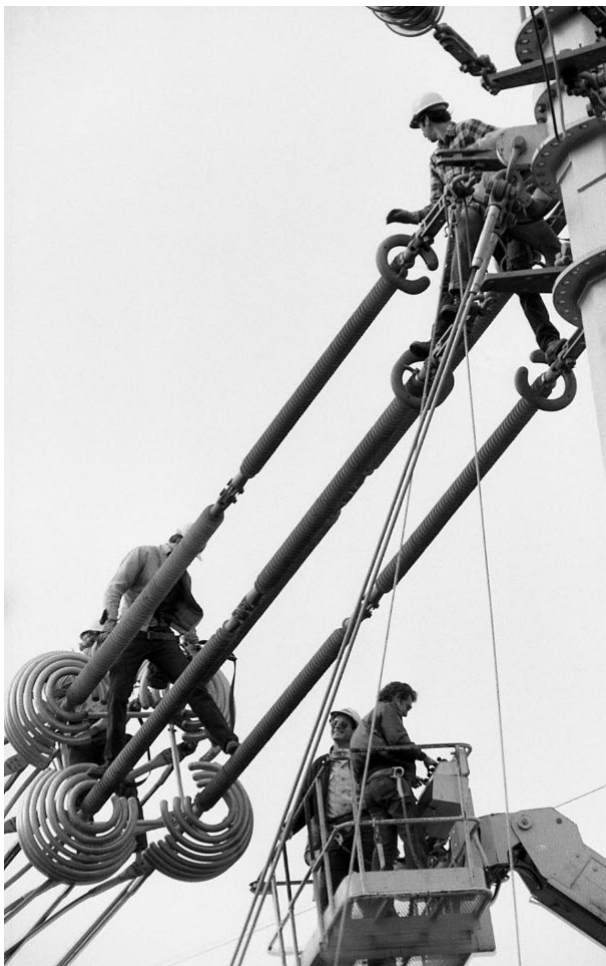
Figure 11. Workers on a test line at the Lyons Test Facility, October 4, 1982. 92
