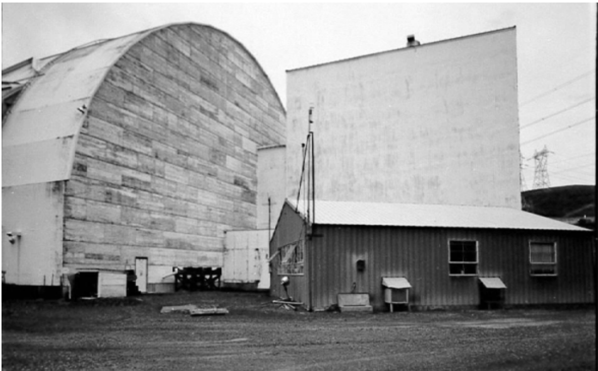
Figure 26. The Control House (right foreground), as documented in the 2016 HAER. The Fog Chamber (right background) is also visible. 153
