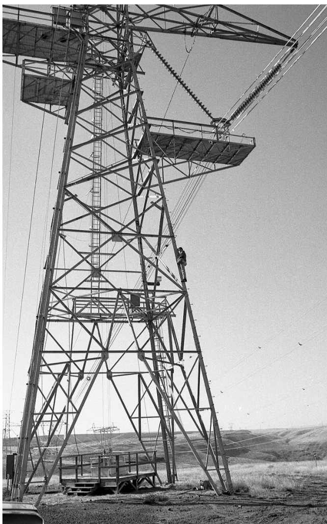
Figure 41. Photograph from ca. 1980 showing the unique platform feature (top right) present on testing towers at the Moro Mechanical Test Facility, which allowed workers to have easier access to equipment. 204
