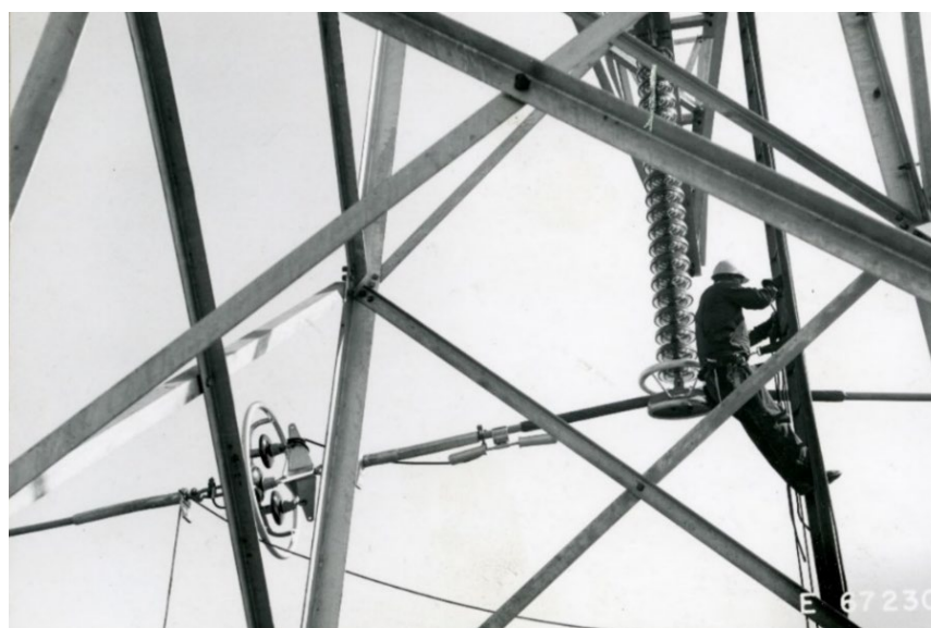
Figure 6. Test line at the HVDC Test Center, September 26, 1963. 62
