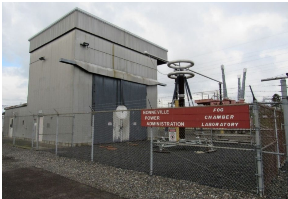
Figure 18. The Fog Test Chamber and attached Test Yard. 122
