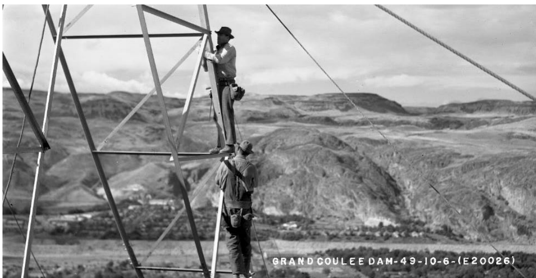
Figure 3. Workers installing a transmission structure at Grand Coulee Dam, 1949. 15
