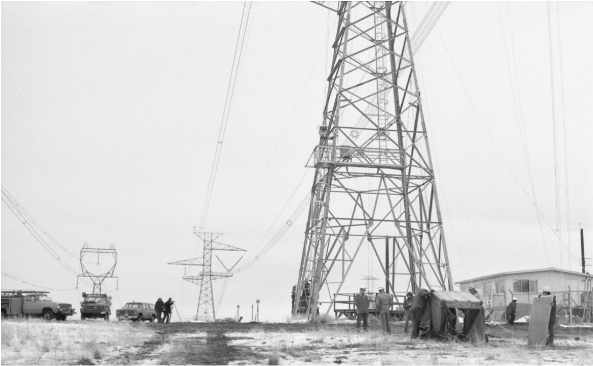
Figure 40. Moro Mechanical Test Facility in November 1978. 196
