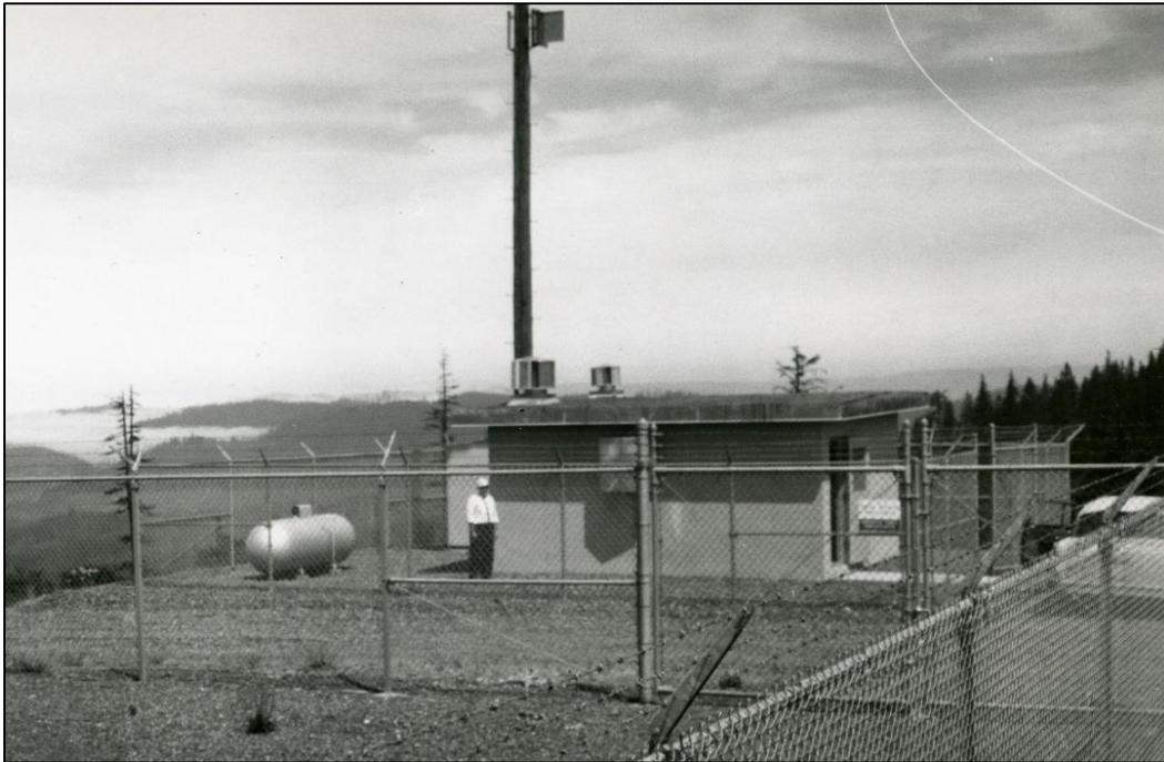
**Figure 70. Wood Monopole Antenna Tower at Kenyon Mountain Microwave Radio Station, 1960 (NARA:KenyonNARAbbox14of52-001)**
