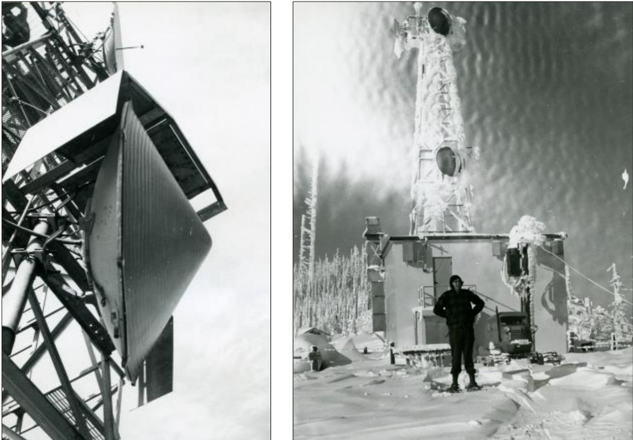
**Figure 17. BPA's thermo-microdome antenna cover (detail left) provided antenna protection in icy conditions at Augspurgen microwave/radio station (right) (NARA:AugspurgenMW1NARAbbox7-025, -035).**
