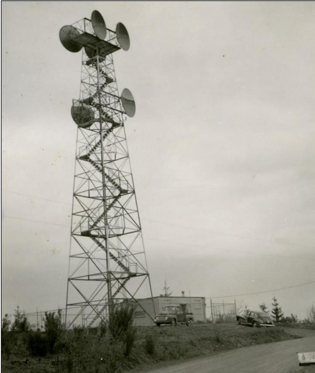
**Figure 68. Four-leg Steel Lattice Antenna Tower with Internal Staircase at Rainier Microwave Radio Station, 1951 (NARA:Rainier4X-002)**
