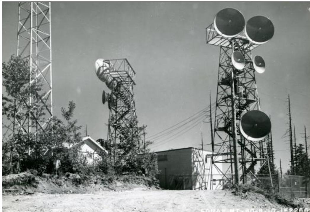
**Figure 12. Squak Mountain radio station, August 10, 1950 (NARA:Squak1NARAbbox27of52-021). Squak Mountain was built as one of three radio “repeater” stations within BPA’s Ross – Snohomish microwave link. New steel towers with parabolic microwave antennas, such as those found at Squak Mountain, inspired references to “flying saucer attachments” mounted on “giant antenna towers” (Currey 1951).**
