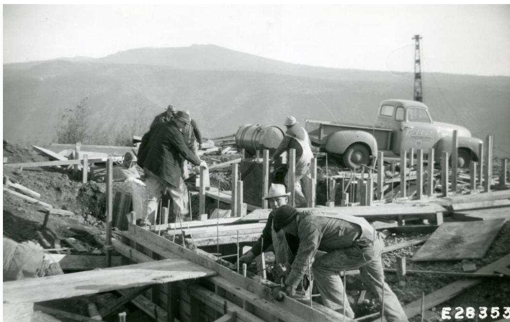
**Figure 3. Biddle Butte Microwave Substation, 1951, workers forming building foundation (NARA:BiddleBNARAbbox10-023)**
