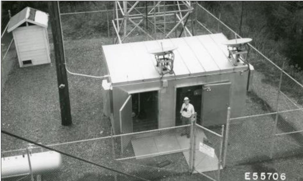
**Figure 22. Goodwin Peak Radio Station, April 28, 1961 (NARA:GoodwinPeakNARAbx31-03). The radio station building is secured to the ground with guy cables. The radio and emergency power equipment rooms have separate exterior entrances.**
