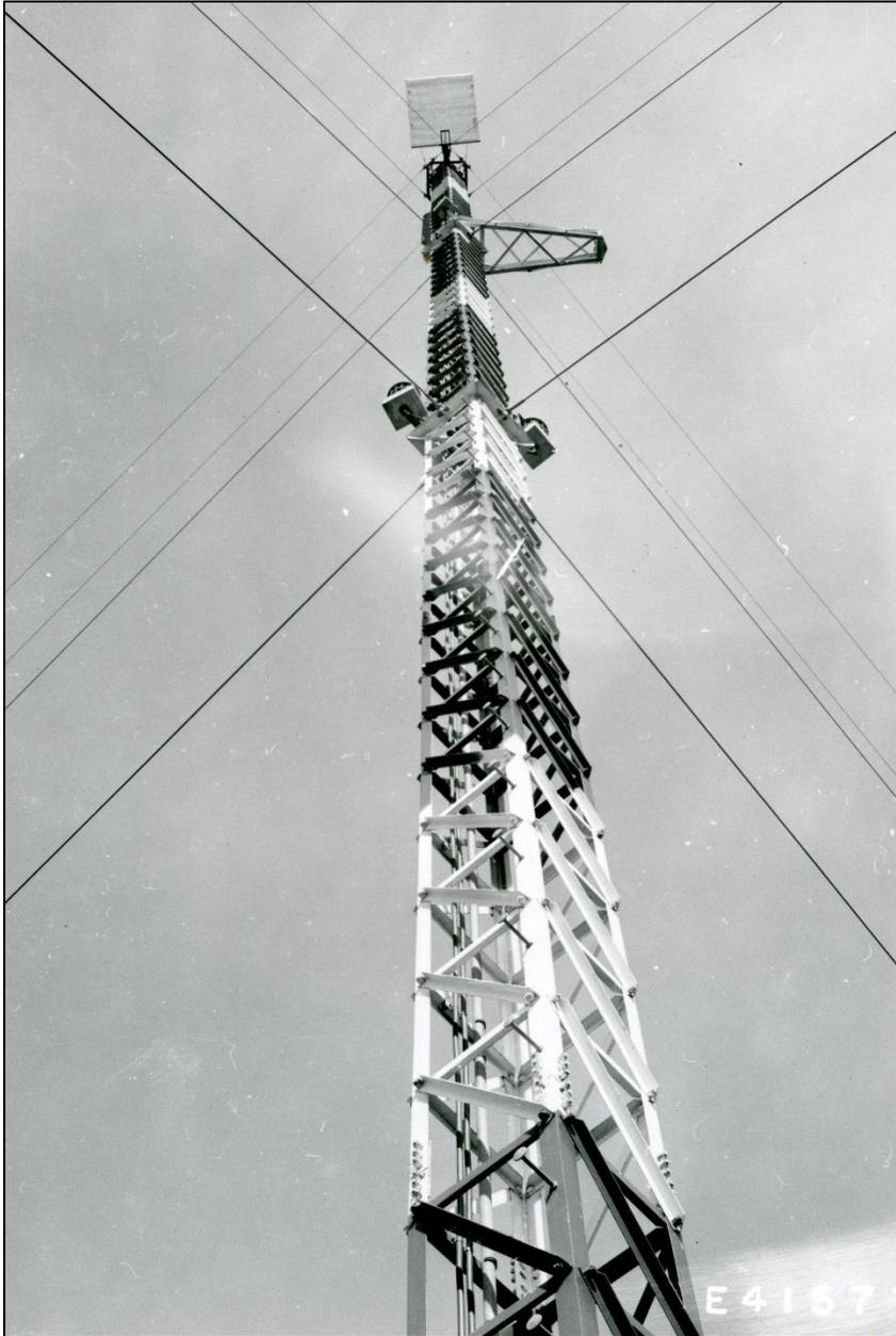
**Figure 69. Steel Lattice Antenna Tower with Guyed Wires at Leneve Microwave Radio Station, 1956 (NARA:LeneveNARAbbox15of52-009)**
