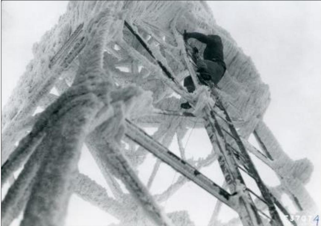
**Figure 14. Augspurgen Mountain Radio Station, February 5, 1954, showing BPA personnel removing ice from the tower ladder (NARA:AugspurgenMW2NARAbbox7-008).**
