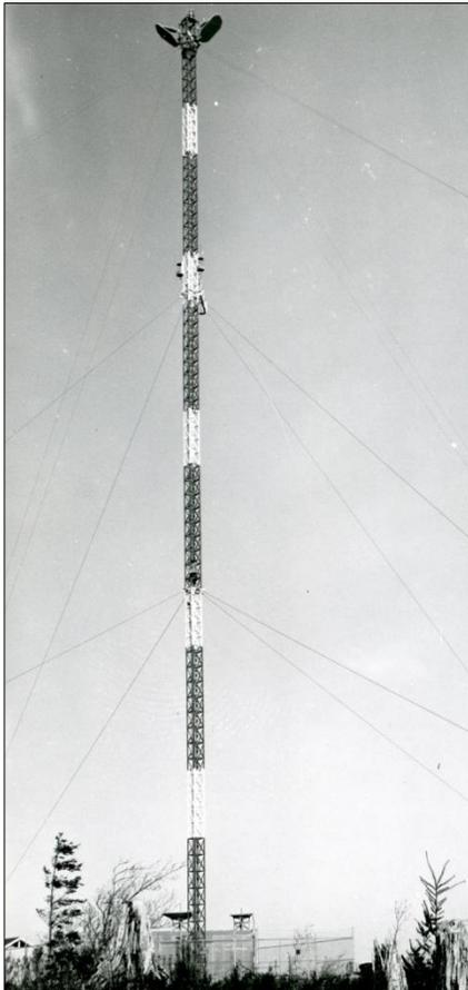
1. The 50-foot self-supported lightweight steel transmission tower with top-mounted platform was installed at Noti and Goodwin Peak radio stations. This type of tower supported the two reflector antenna combinations used at these stations (Marihart and Wylie 1956:534).
