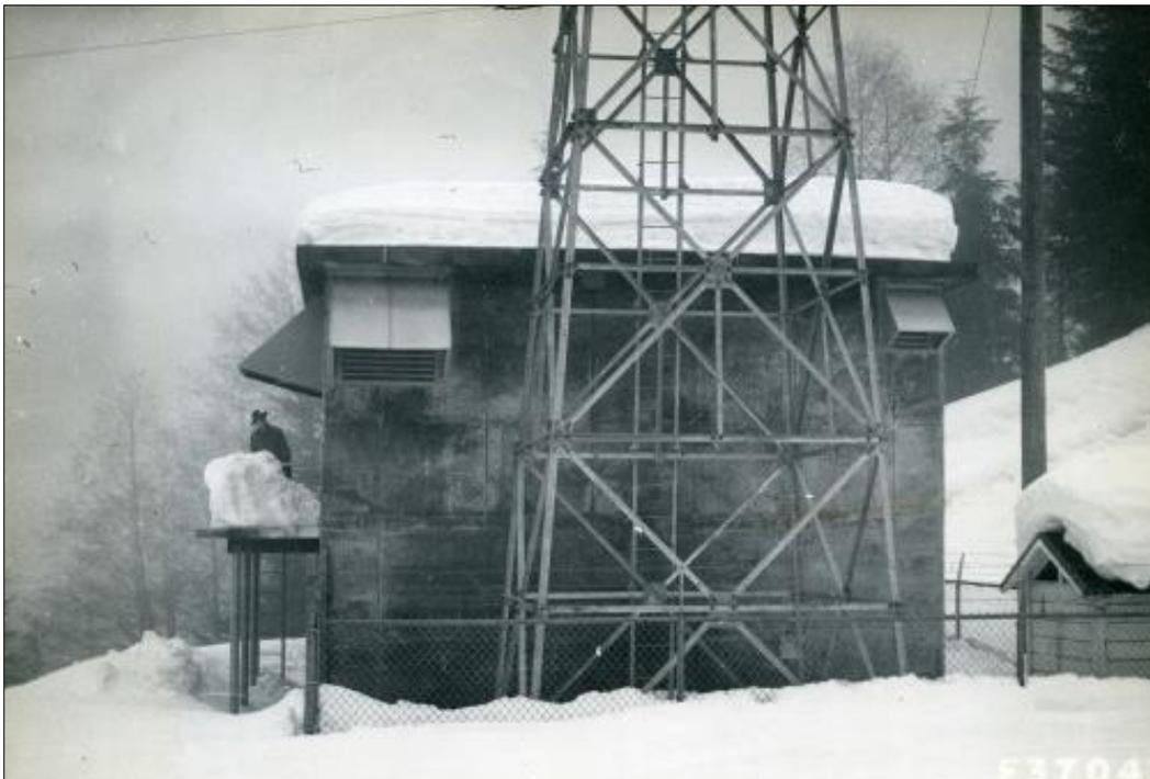
Figure 16. Rockdale Radio Station on February 9, 1954. Even the platform in front of the second-story entrance has an accumulation of snow. The exhaust vents are located near the roofline to prevent obstruction by snow (NARA:Rockdale2NARAbbox21of52-013).
