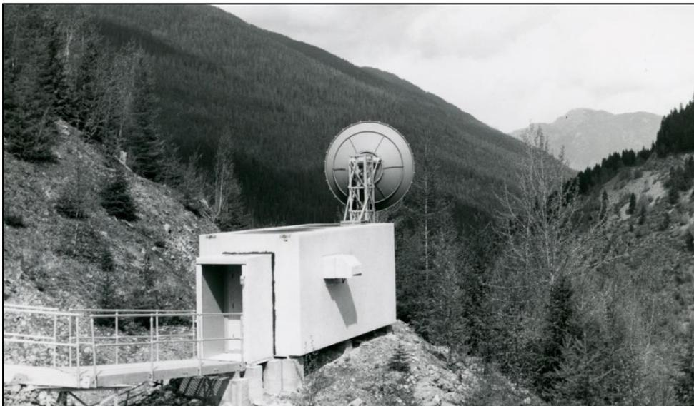
**Figure 4. Hungry Horse Dam Microwave Radio Station with line of sight to Teakettle Mountain Passive Repeater.**
