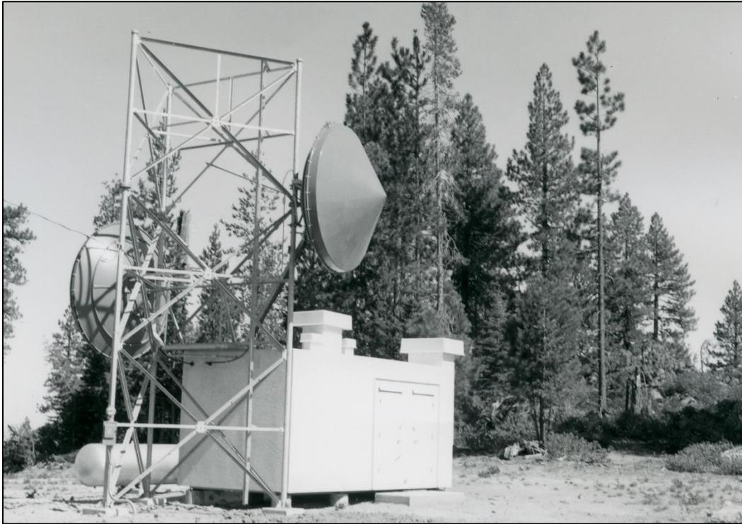
**Figure 66. Three-leg Antenna Tower at Applegate Butte Microwave Radio Station, 1967 (NARA:ApplegateX-001)**
