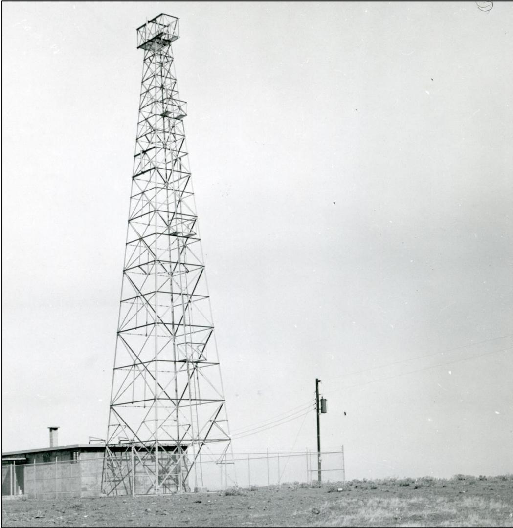
**Figure 67. Four-leg Steel Lattice Antenna Tower at Wasco Microwave Radio Station, 1953 (BPA Library)**
