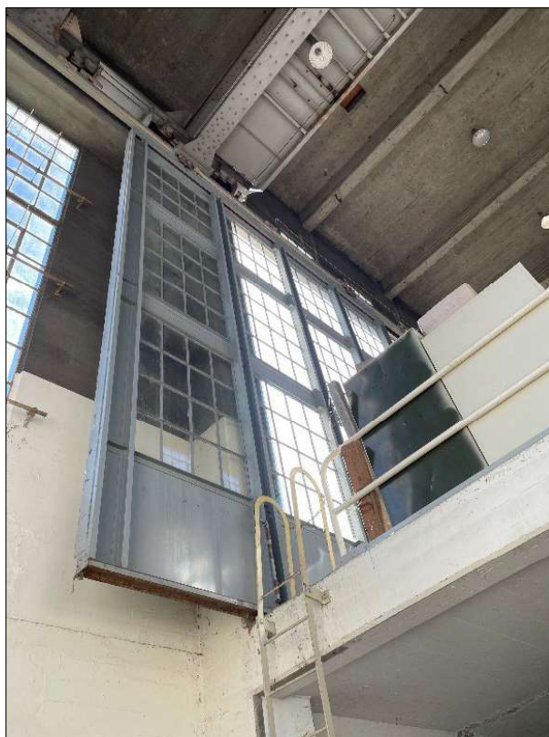
Photograph 24 of 46: OR_PolkCounty_SalemSubstation_0024 View of sliding untanking tower door from transformer pit, looking northeast (2024)
