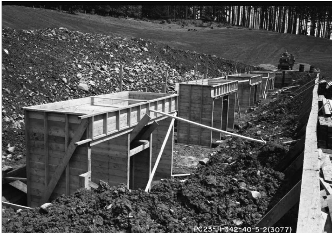
Figure 22: "Salem Substation. Foundations for 115kV oil circuit breakers. Looking west." (1940) Source: Bonneville Power Administration via National Archives Seattle
