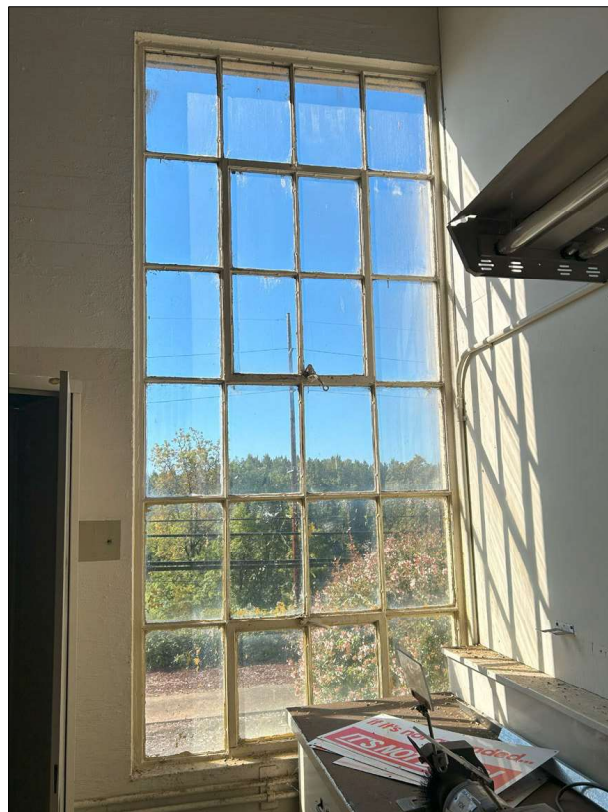
Photograph 32 of 46: OR_PolkCounty_SalemSubstation_0032 Close-up of 24-light fixed steel sash with hopper and awning features typical of Control House, looking south (2024)
