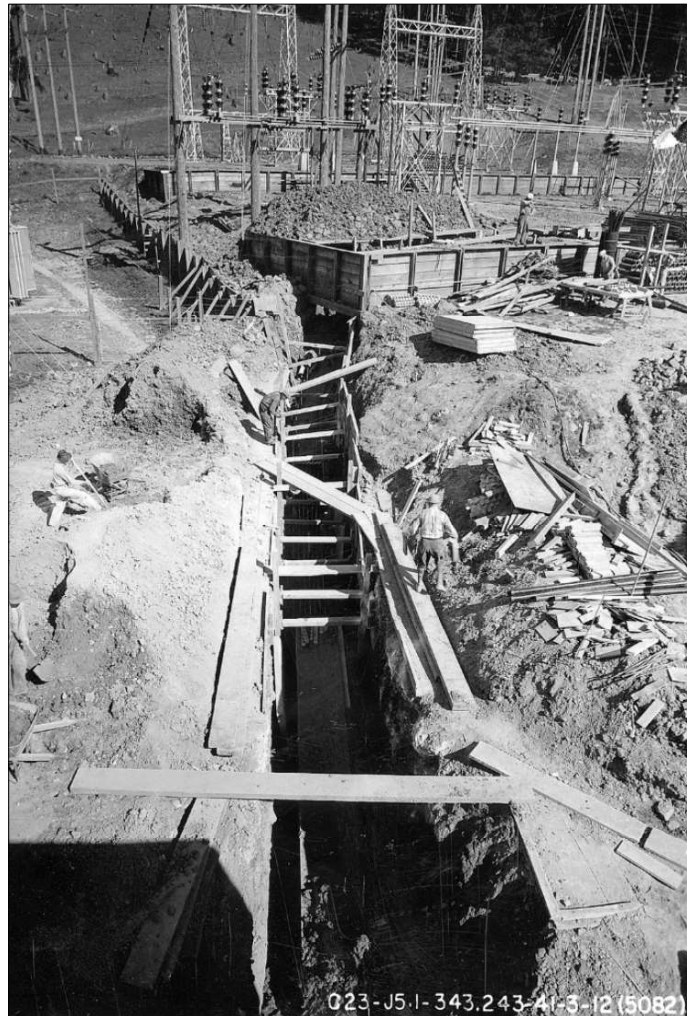
Figure 28: Trenching of Salem Substation Switchyard for drainage (1941)
