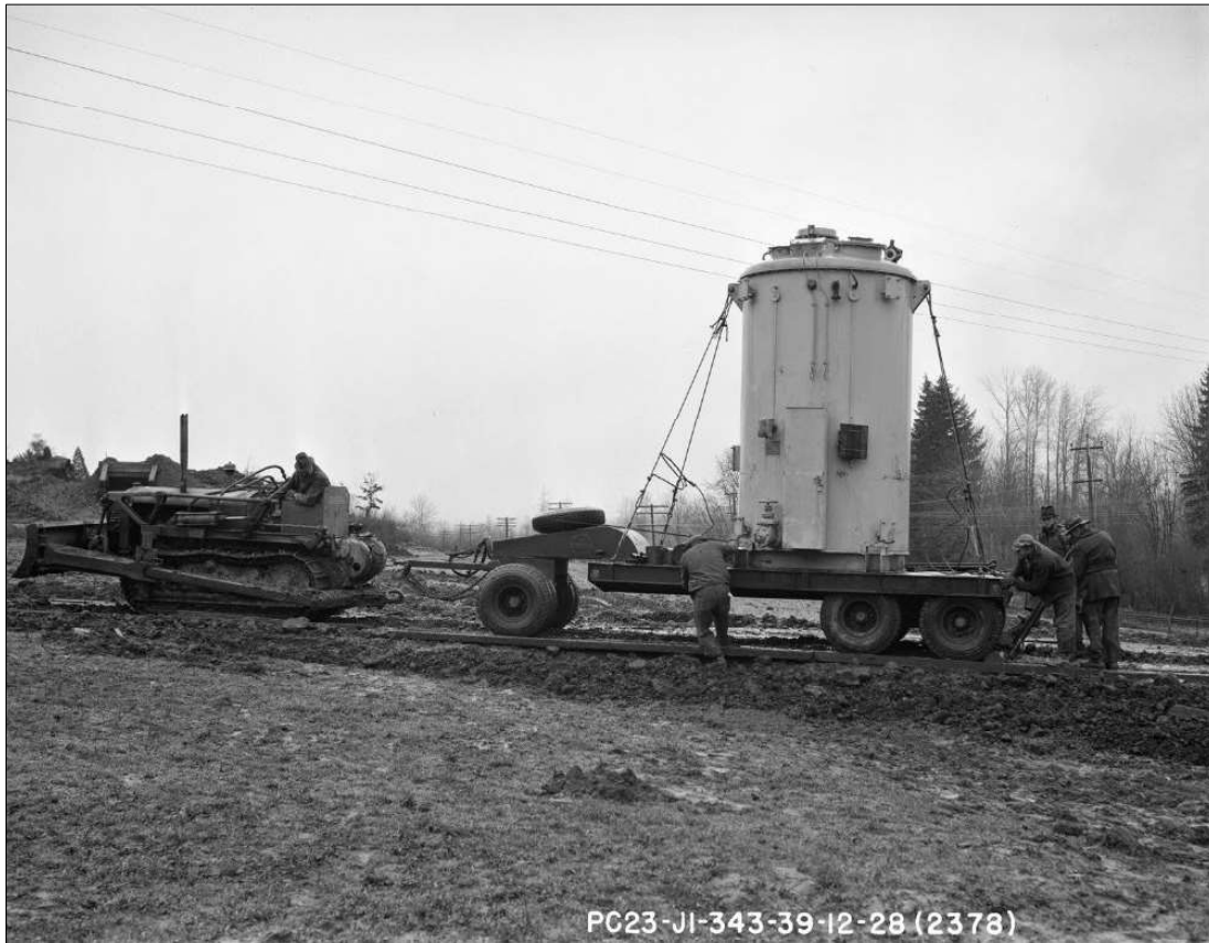
Figure 18: Circuit Breakers for temporary switchyard rolled into place (1939)
