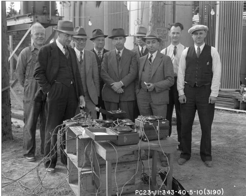
Figure 21: Testing equipment used for phasing in transformer bank (1940)
