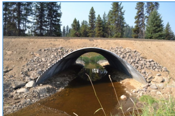
2015004 Elk Creek Culvert Replace (After)
