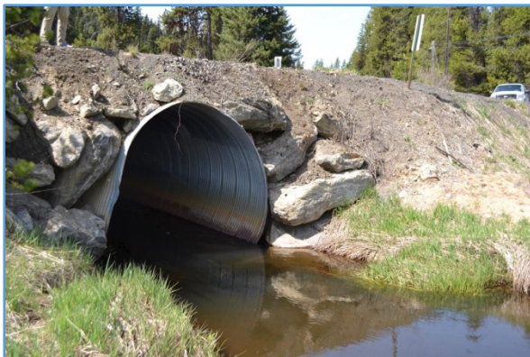
2015004 Elk Creek Culvert Replace (Before)
