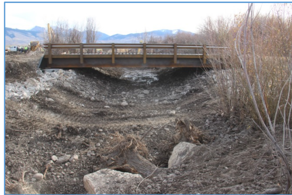
2015067 McCoy Creek culvert replacement (after)
