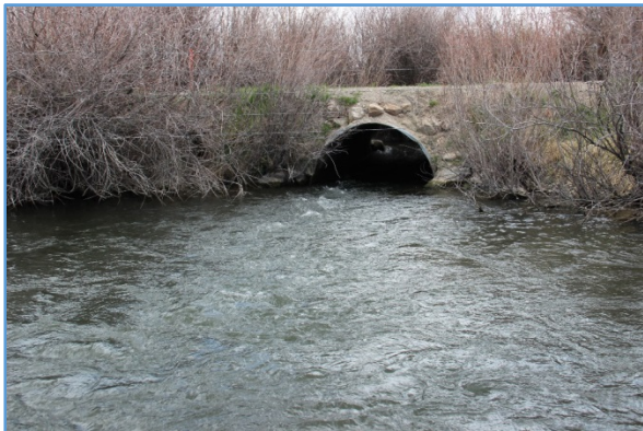
2015067 McCoy Creek culvert replacement (Before)
