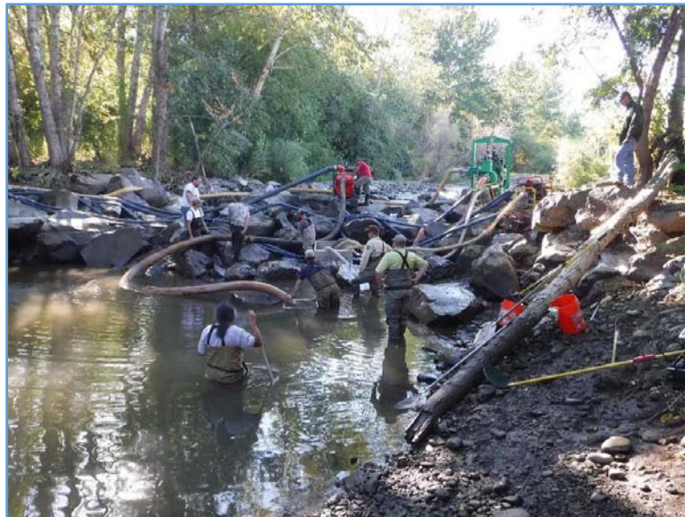
2015075 Smith Sill Riffle Widening Work Area Isolation
