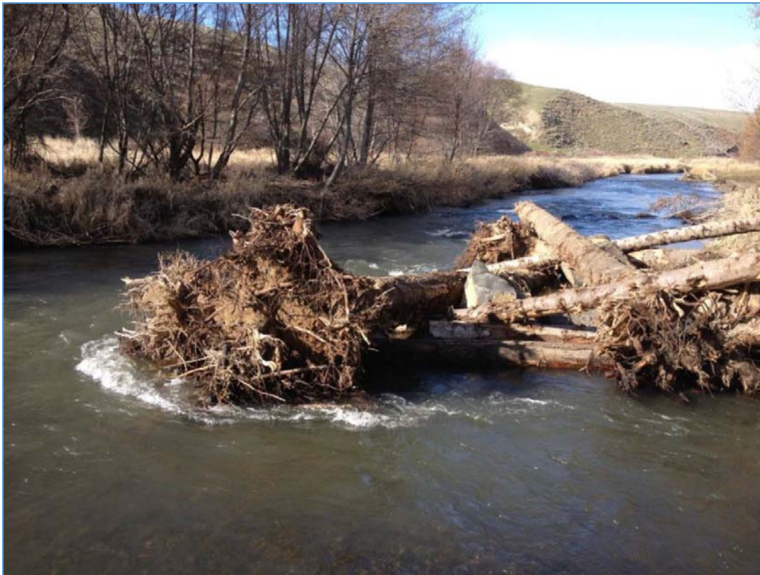
2015001 Tucannon River Large Wood Structure
