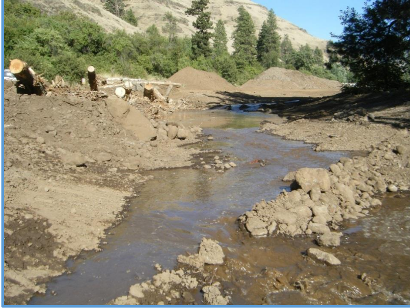
2018063 – Hutchinson Project – Extensive earthwork
