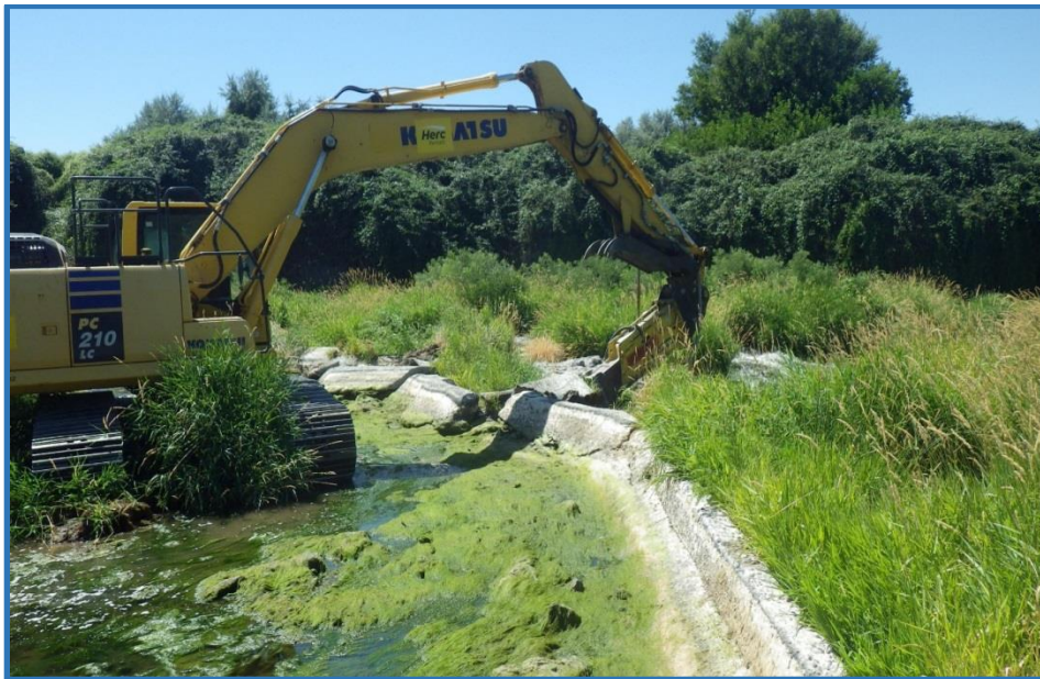
2018035(Brownell Dam Removal)
