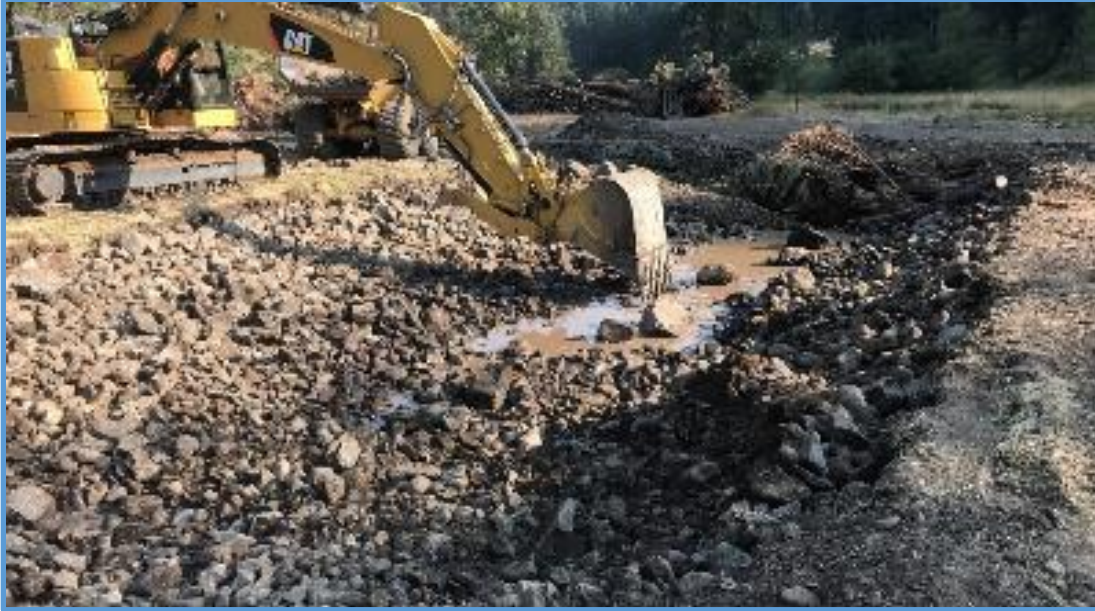
2018033(Rock Creek)Boulder Placement
