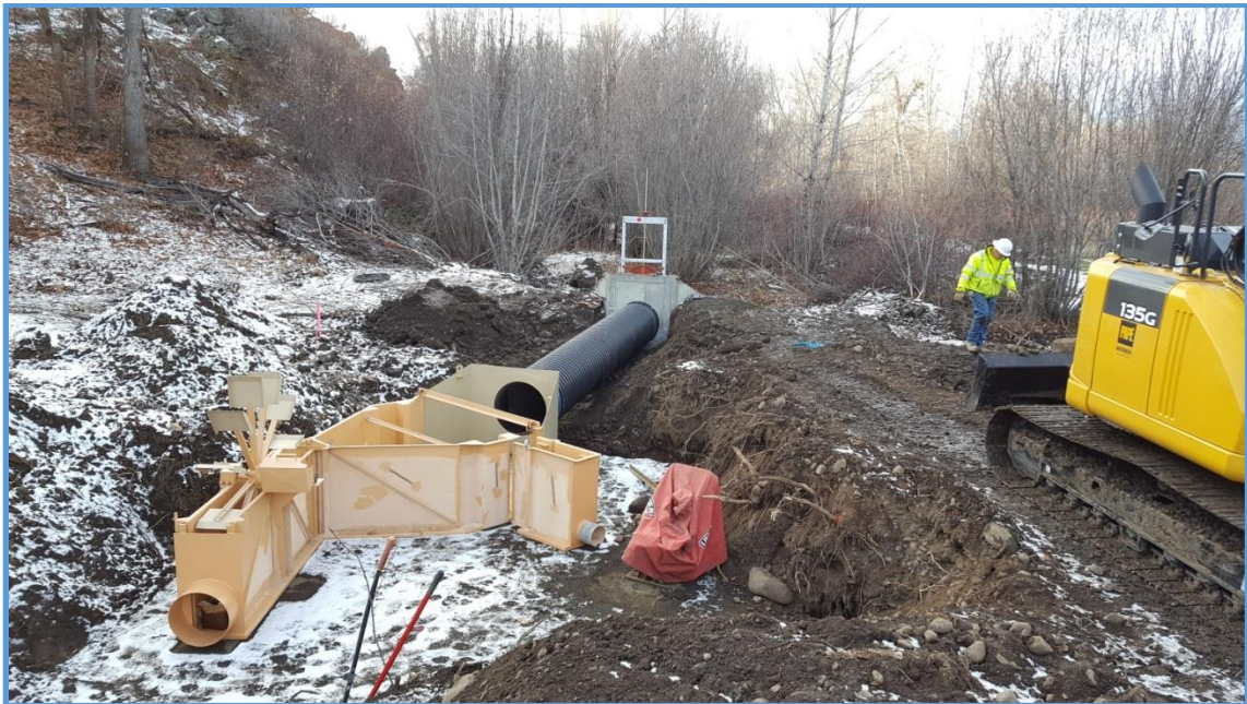
2018098(Placement of Fish Bypass)_2
