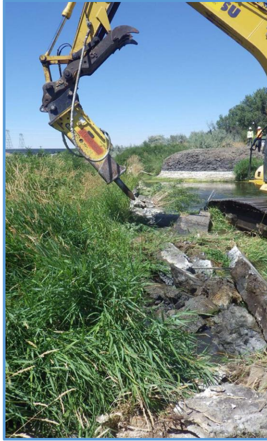
2018035(Brownell Dam Removal)
