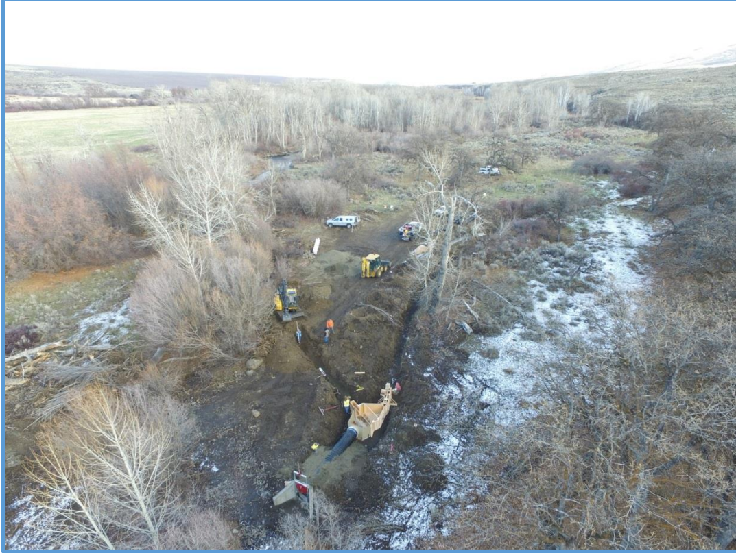
2018098(Placement of Fish Bypass)_1
