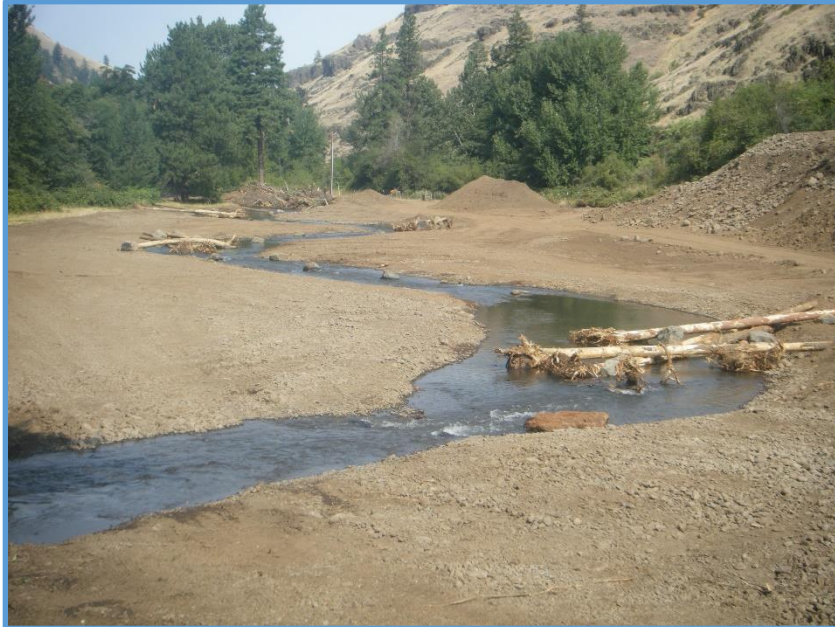
2018063 – Hutchinson Project – Extensive earthwork
