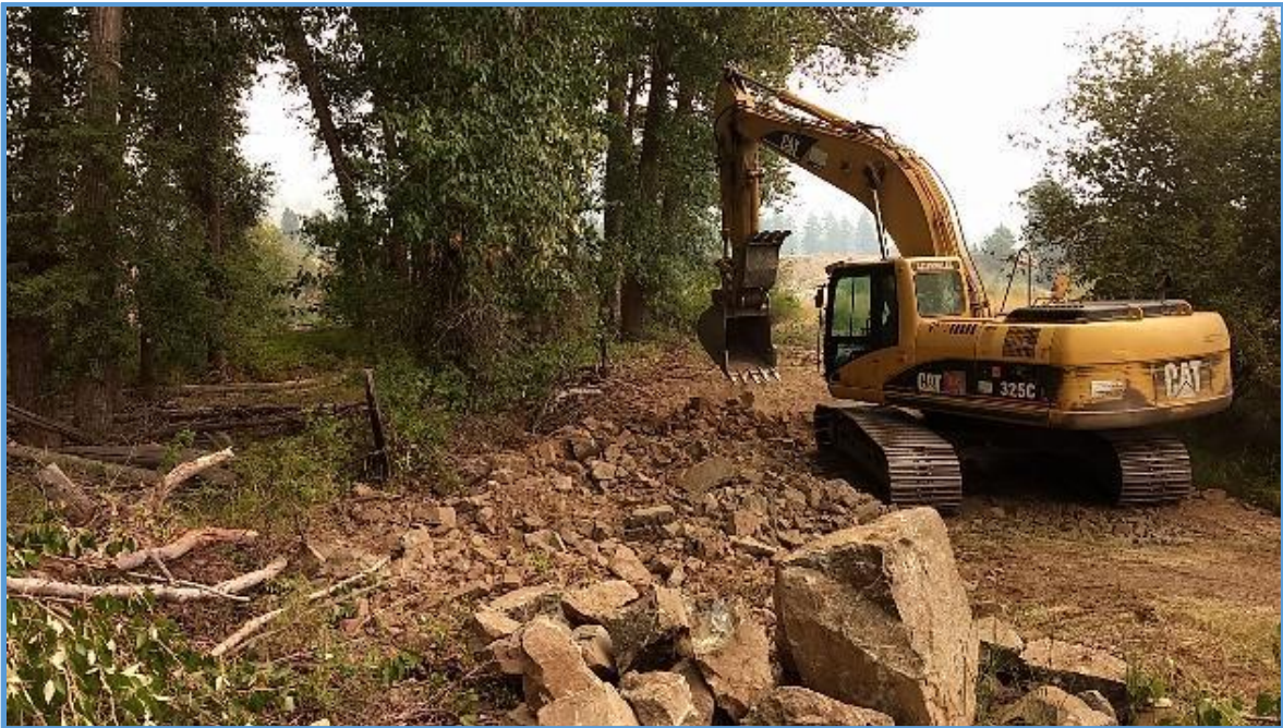
2018101(WDFW Flow Connection)Levee Removal
