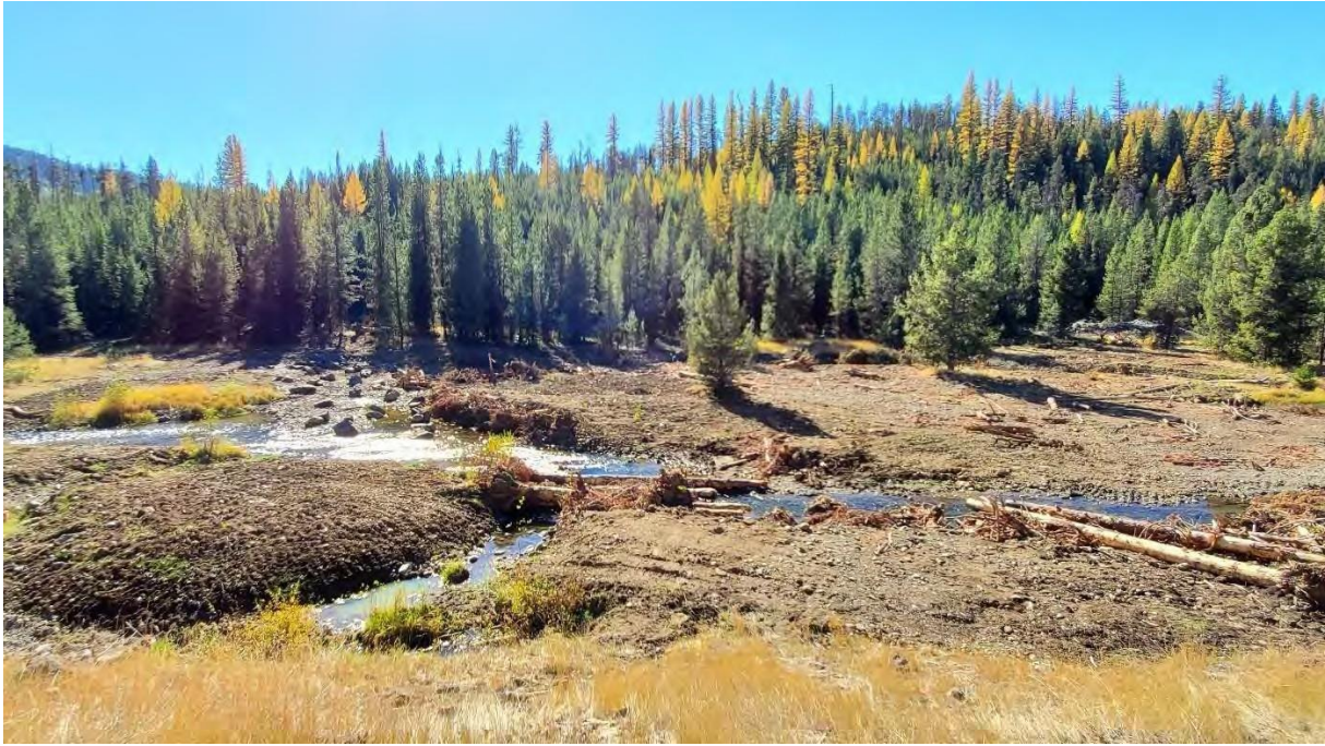
20200070 (Granite Creek) Post Phase 1 Construction
