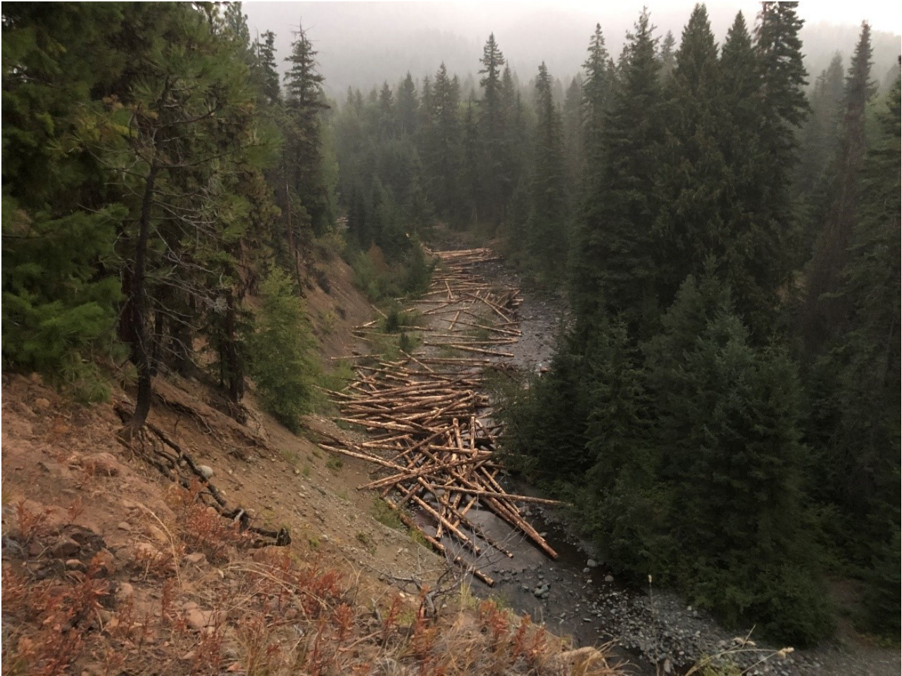
2020077 (NF Teanaway) Loose Wood Placement
