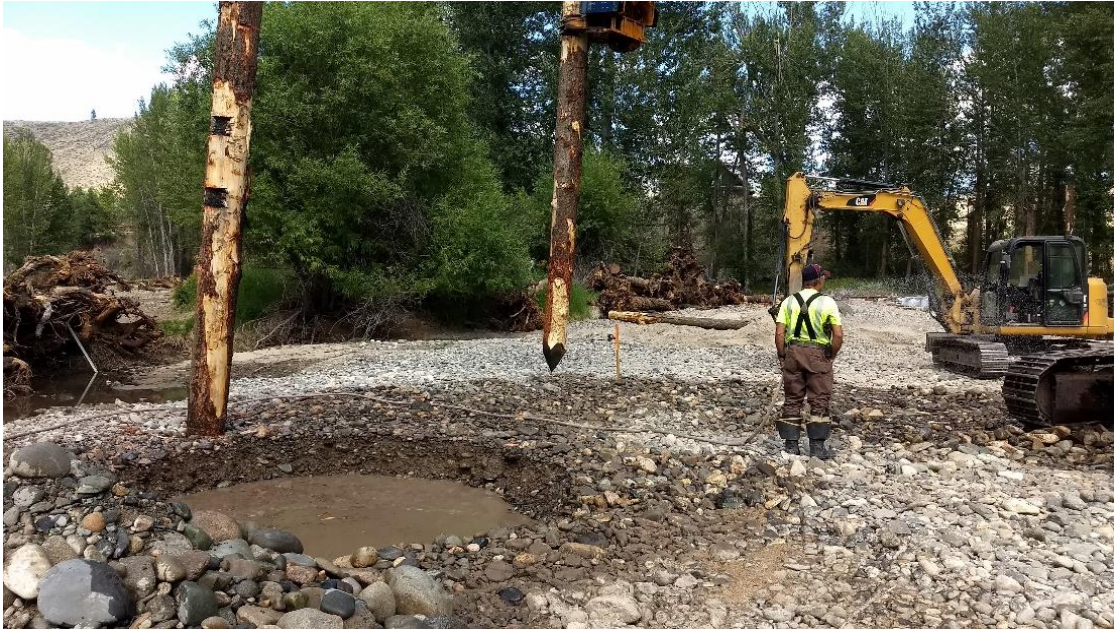
2020046 (M2 Barkley Bear) Driving Piles for Engineered Log Jam
