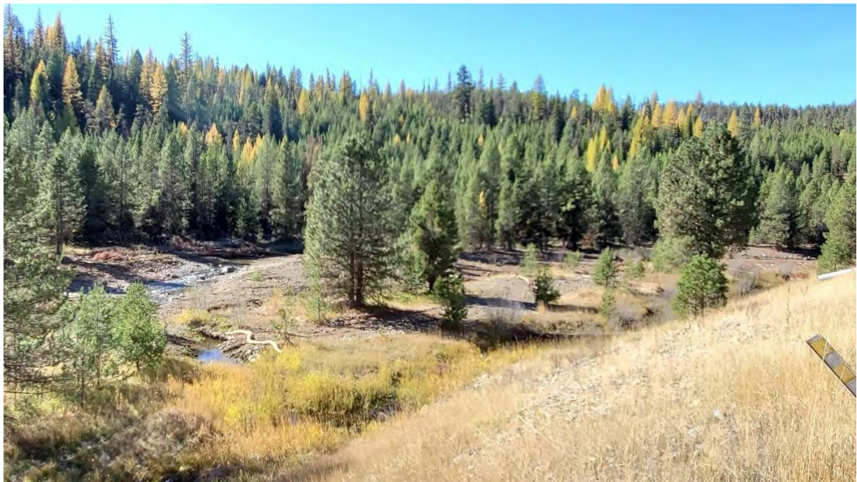
20200070 (Granite Creek) Post Phase 1 Construction downstream
