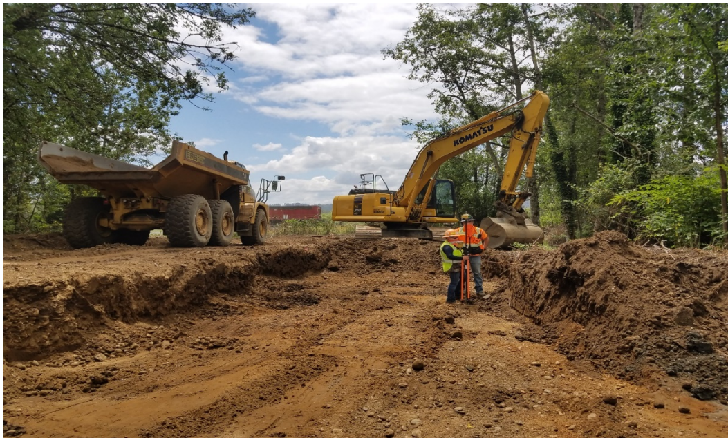
2020074 (Stiegerwald) Aerial View South of Gibbons Creek after realignment and excavation
