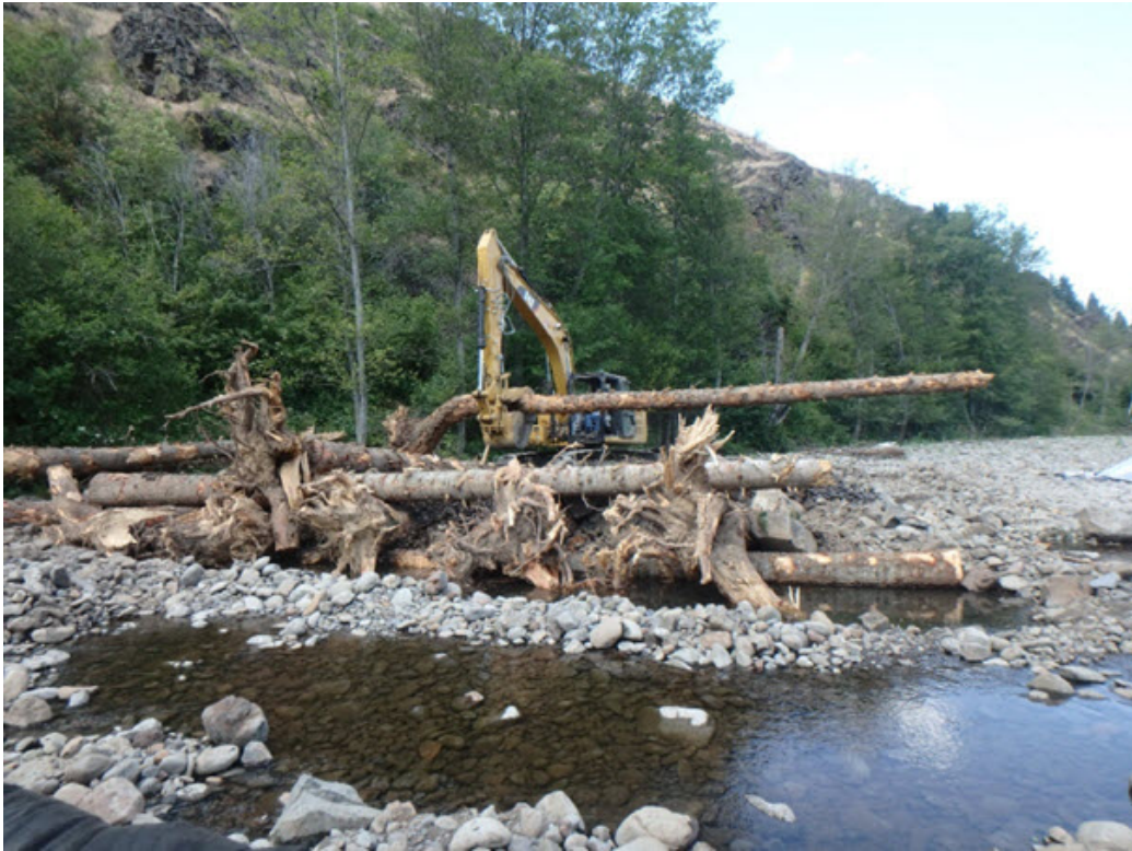
2020092 (Umatilla Anadromous Fish) Log Jam Installation
