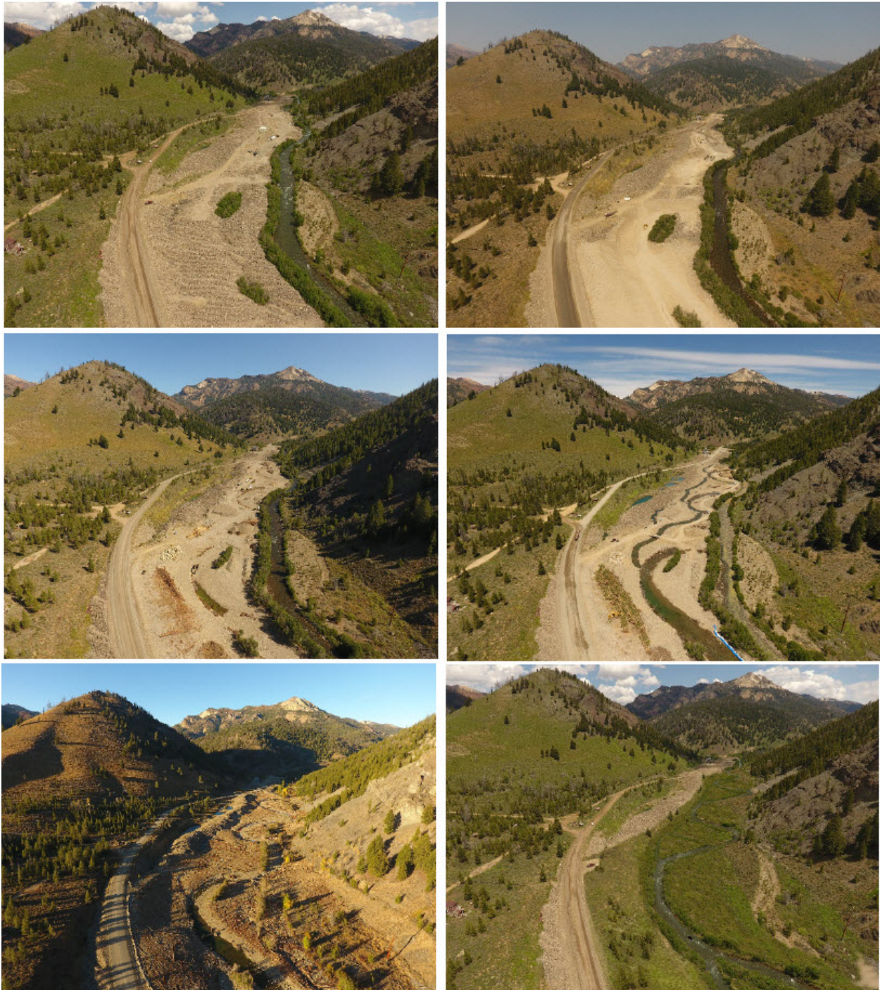
Bonanza City Floodplain Restoration. Before any work (Top Left), end of phase 1 (Top Right). End of phase 2, middle left, during phase III bottom left, artist rendering after 10 years (Bottom right).
