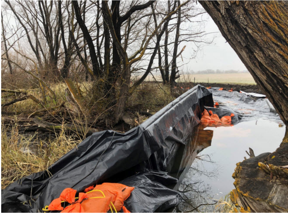
2020101 (Coleman Creek) Work Area Isolation
