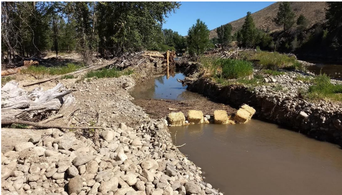
2020046 (M2 Barkley Bear) Newly Constructed Side Channel sediment control
