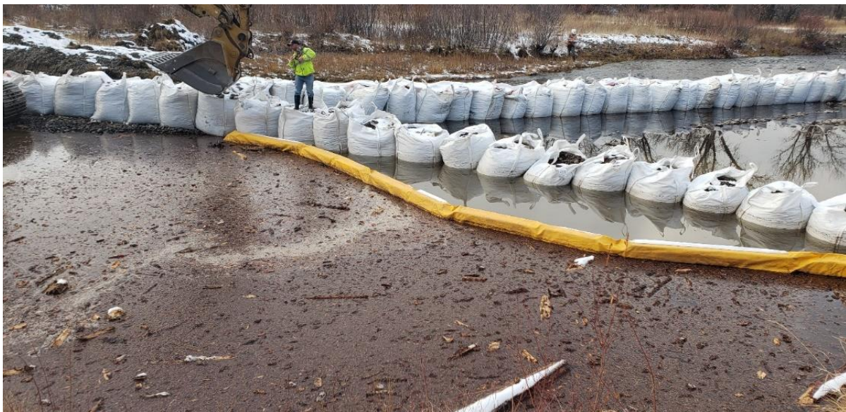
2020032 (Longley Meadows) Cofferdam and Silt Fence
