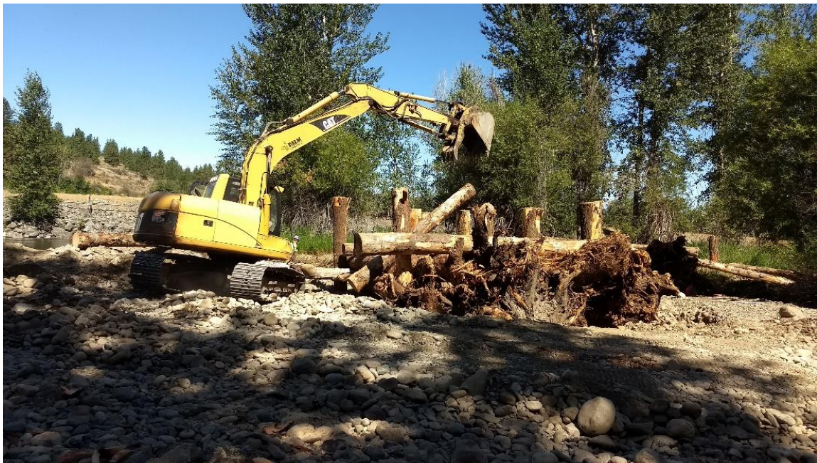
2020046 (M2 Barkley Bear) Constructing Side Channel Engineered Log Jam
