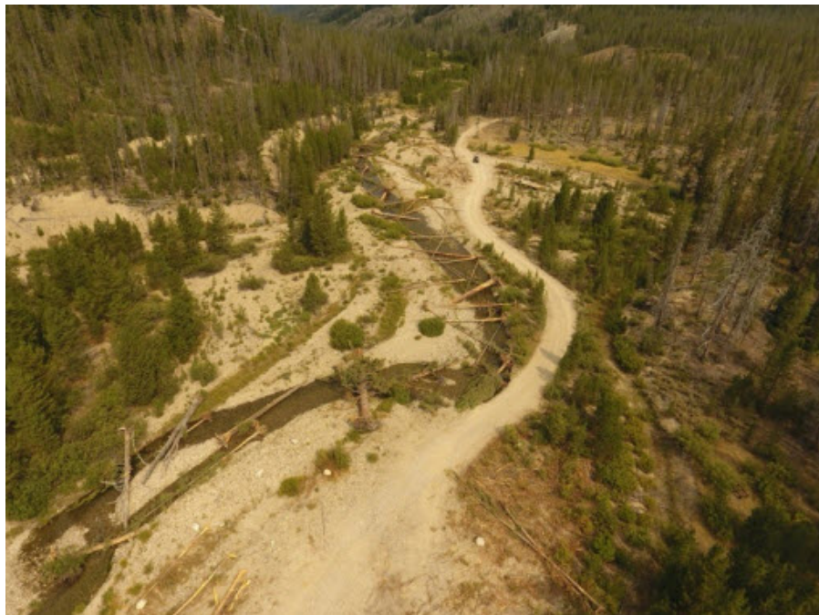
2020069 (Eightmile Creek) Reach A After
