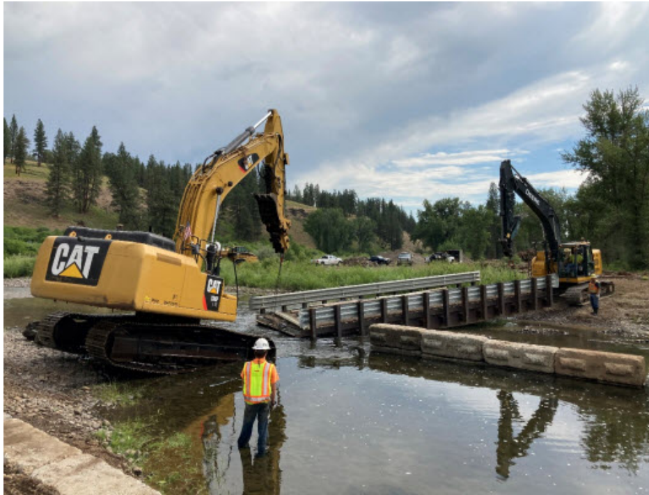
2020032 (Longley Meadows) Temporary Bridge Placement
