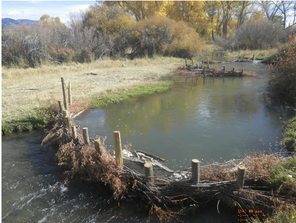
2020065 (Lower Page) Channel Spanning BDAs
