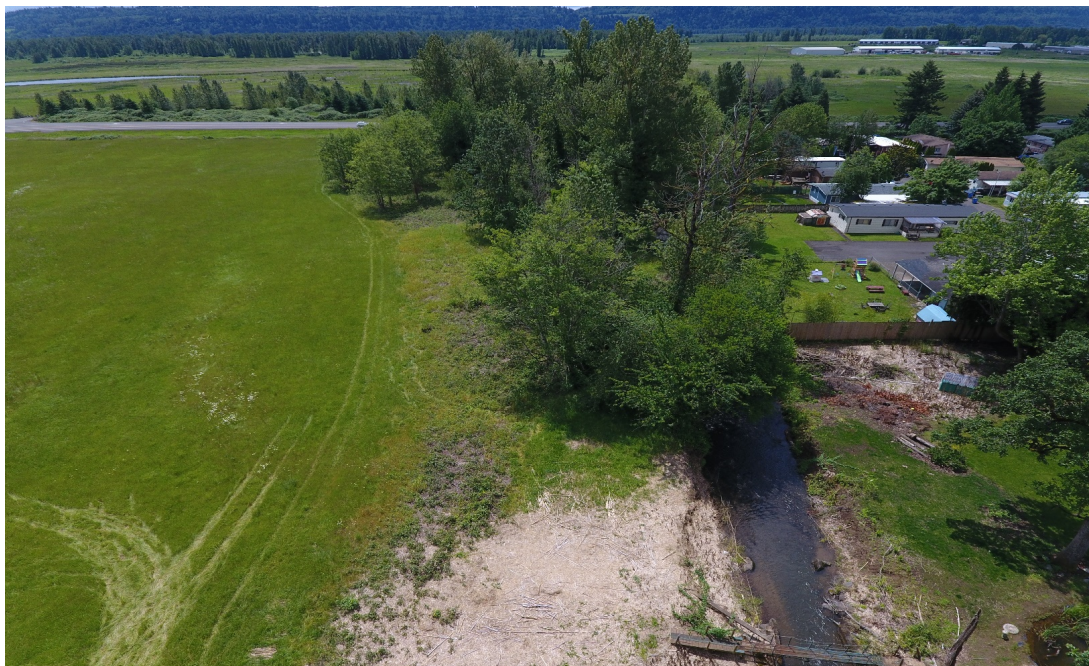
2020074 (Stiegerwald) Aerial View South of Gibbons Creek before realignment and excavation
