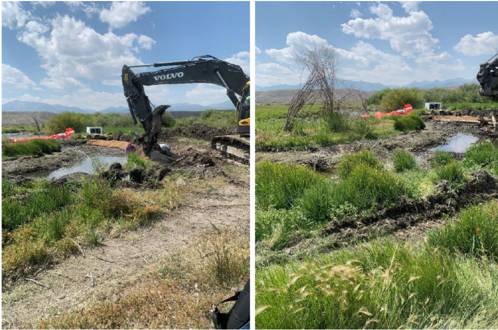
2020094 (Lemhi River Big Springs Confluence) During
