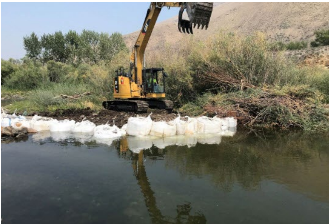
Figure 19: 2021072(Henry Reach) Isolated Work Area
