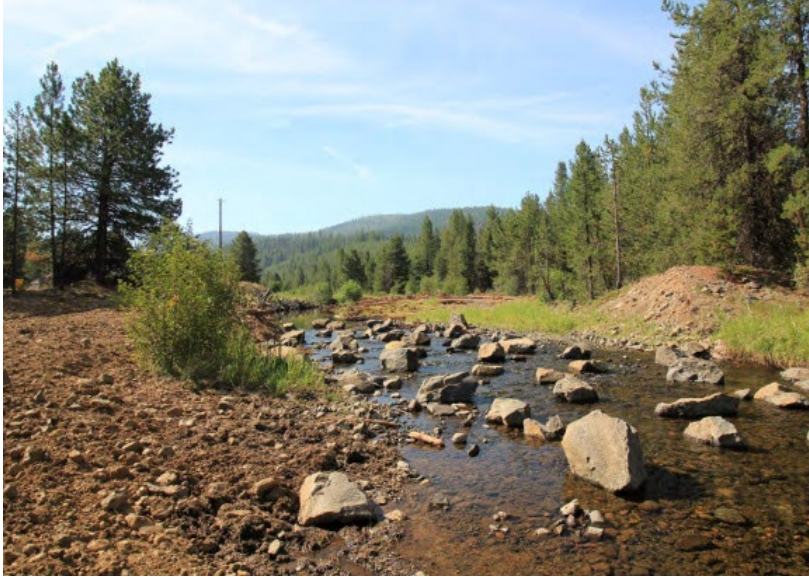
Figure 33: 2021110(Granite Creek)Floodplain Rock Placement
