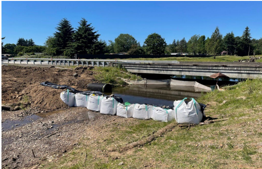
Figure 14: 2021(Stiegerwald)Work Area Isolation
