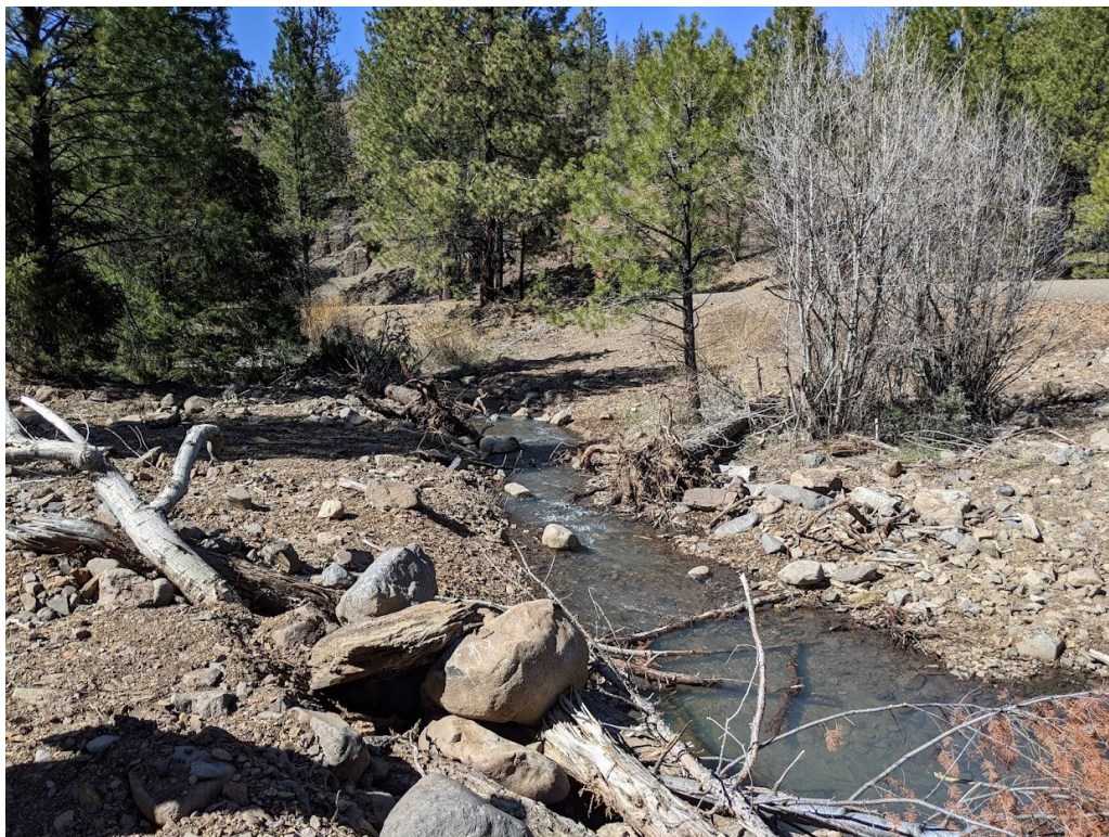
Figure 7: 2021045 (Trout Opal Creek) Remeandering Stream Channel
