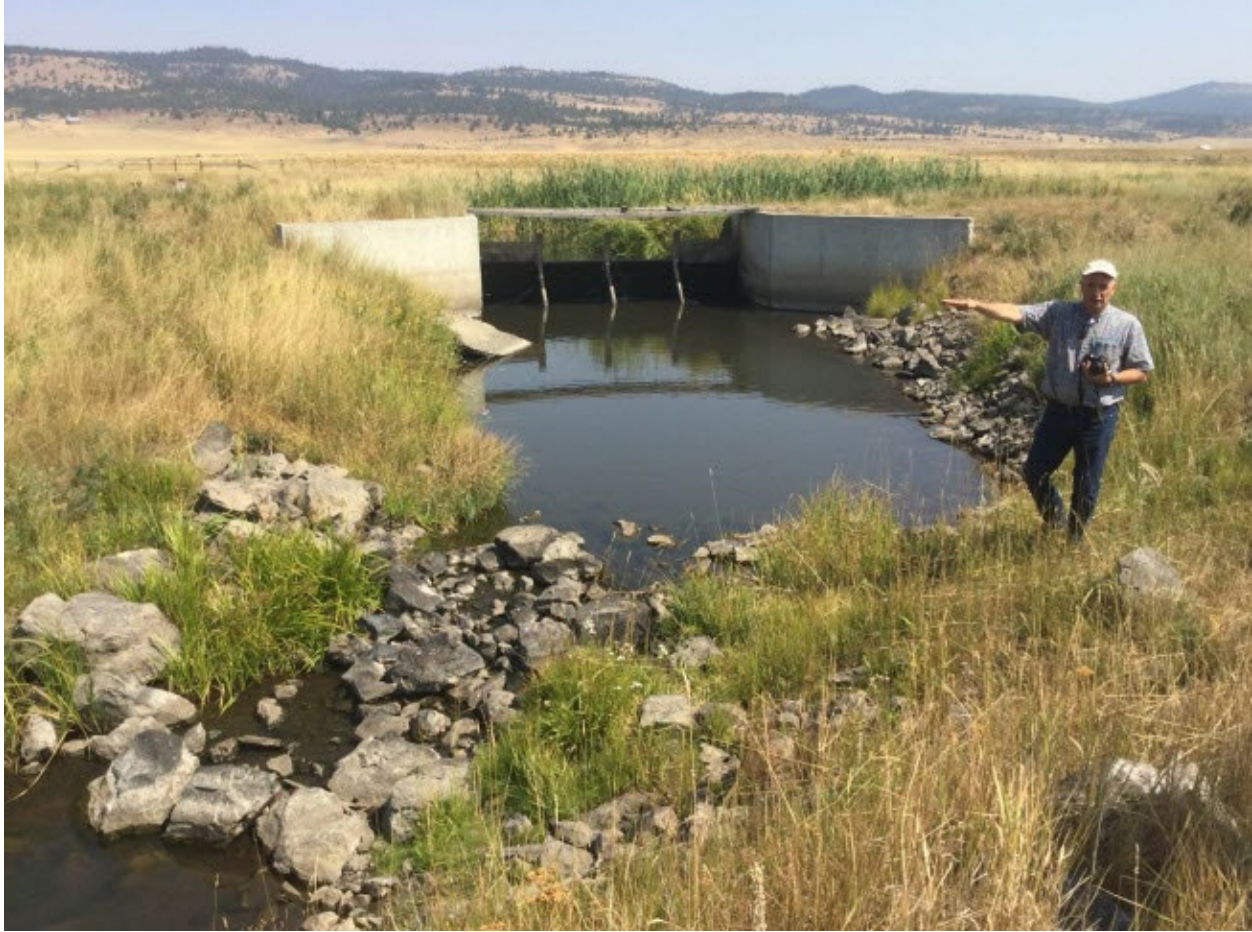
Figure 27: (2021024)Fox Creek McGirr Diversion to be removed
