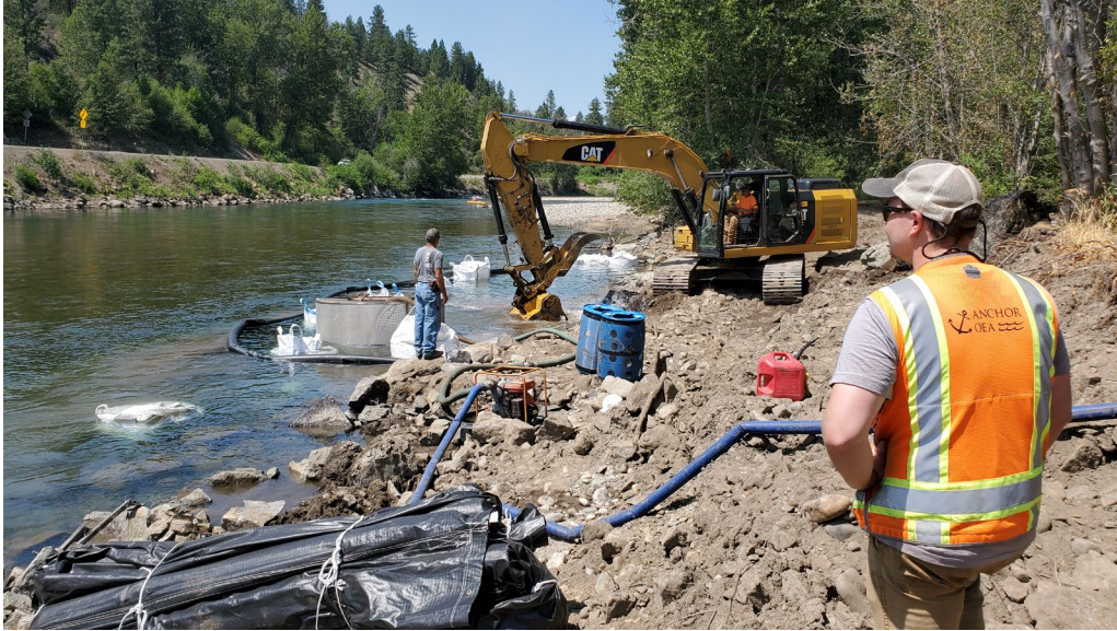
Figure 16: 2021054(Barkley Bear) Work Area Isolation
