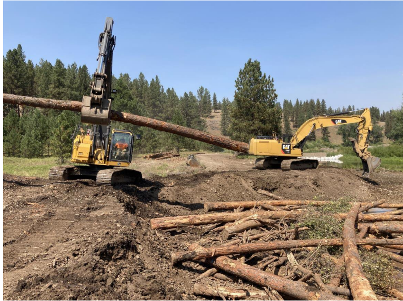
Figure 41: 2021075(Longley Meadow)LWD Install
