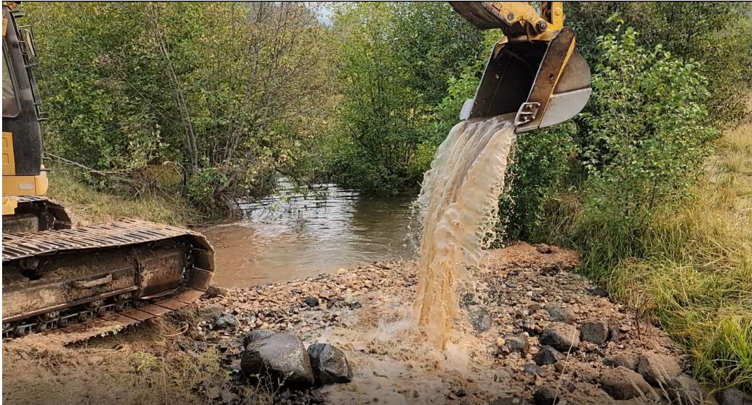
Figure 29: 2021106(Lower Fry Meadow)Riffle Construction
