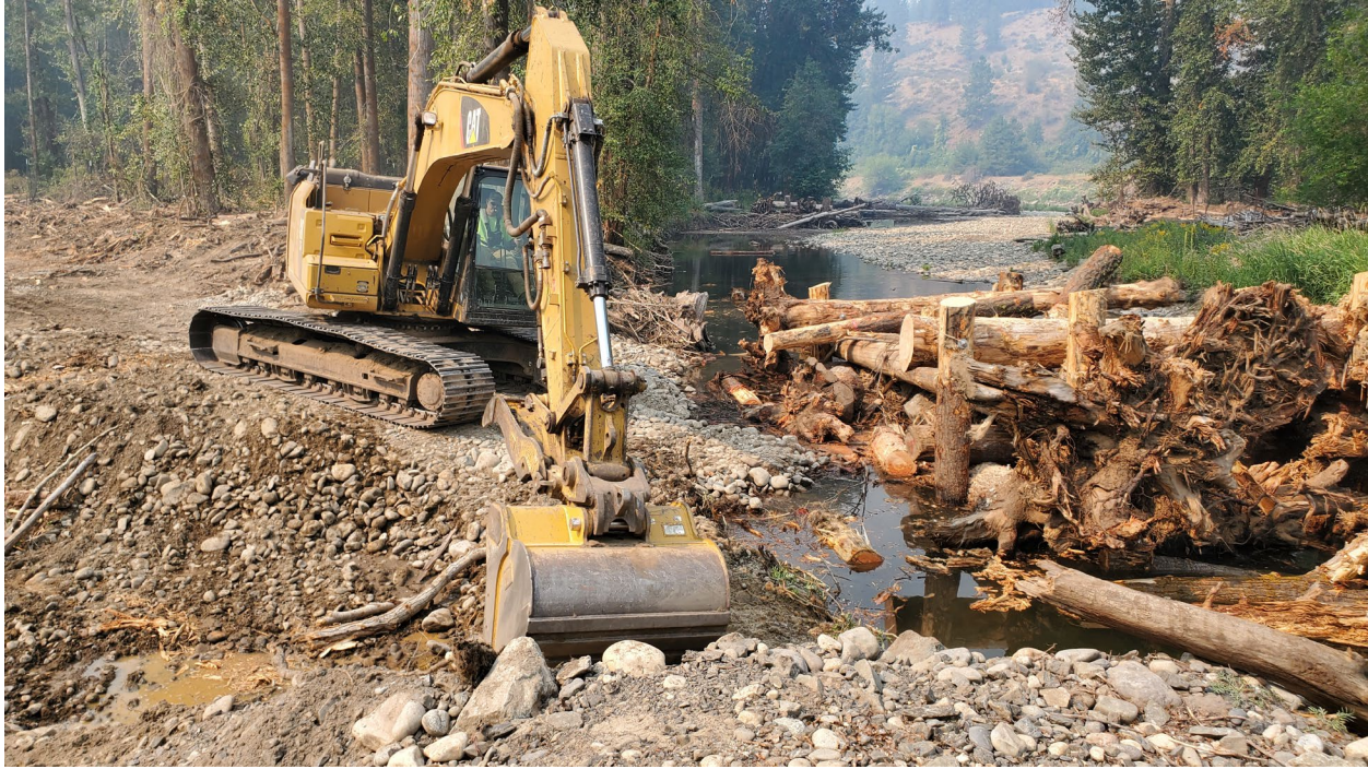
Figure 17: 2021054(Barkley Bear) Engineered Log Jam
