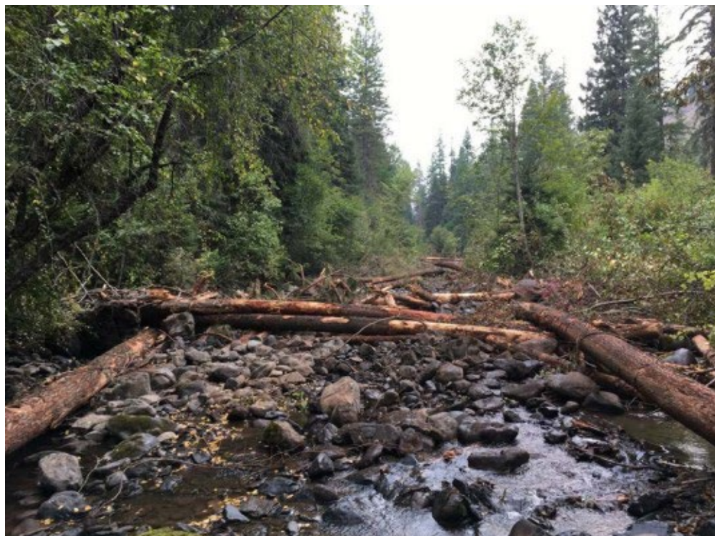
Figure 3: 2021008(Indian Creek) Dam Removal After
