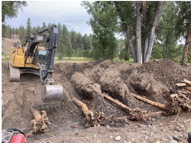
Figure 42: 2021075(Longley Meadow)LWD Installation
