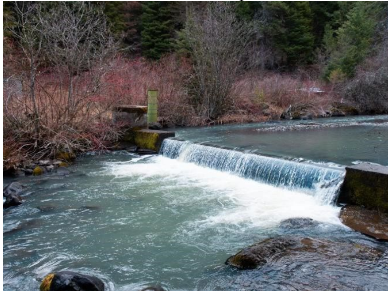
Figure 2: 2021008(Indian Creek) Dam Removal Before
