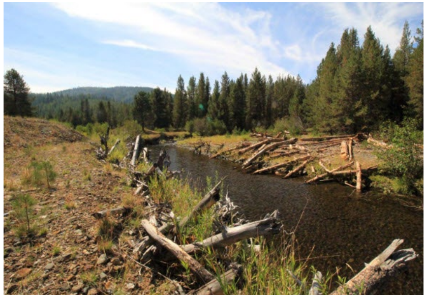
Figure 34: 2021110(Granite Creek)Floodplain Wood Placement
