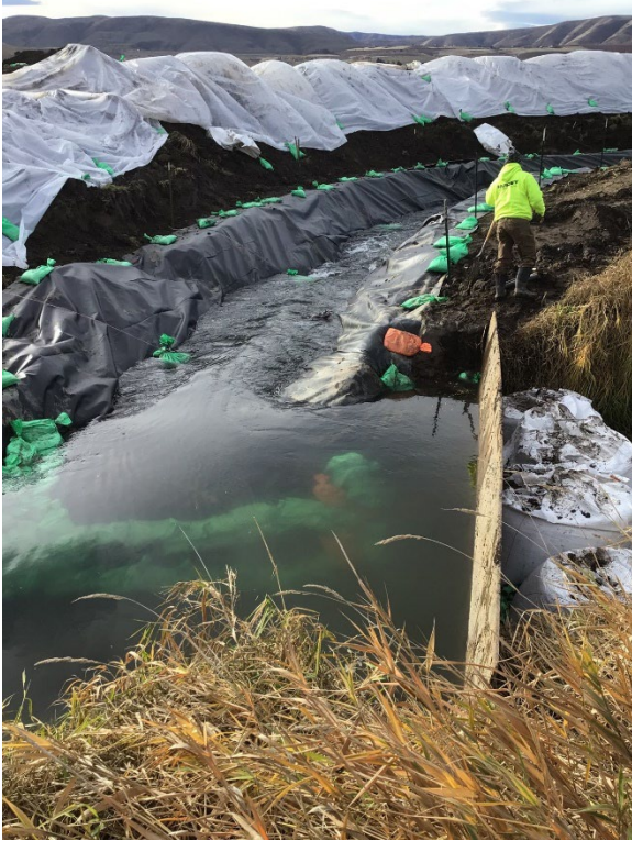
Figure 39: 2021122(Parke Creek)Bulk Bags to divert water
