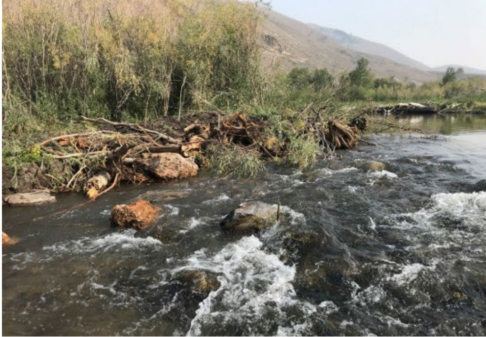
Figure 18: 2021072(Henry Reach)Completed Riffle
