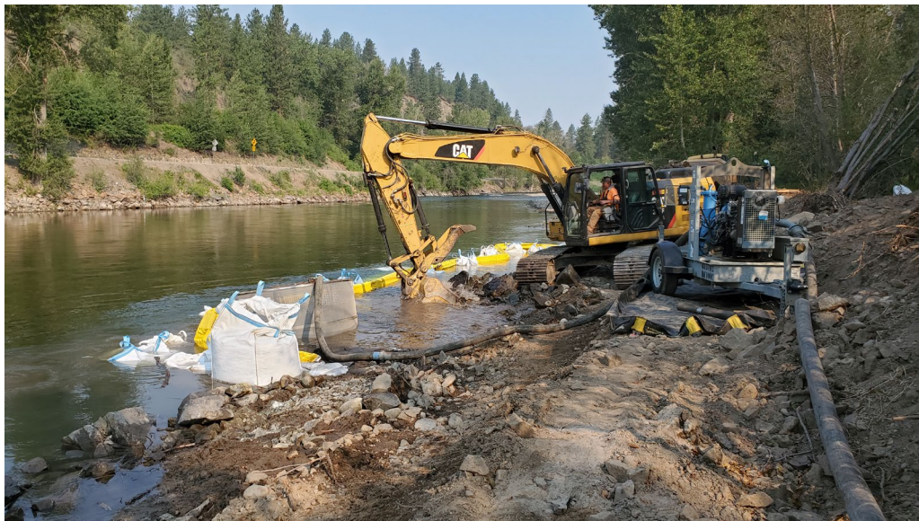
Figure 15: 2021054(Barkley Bear) Work Area Isolation
