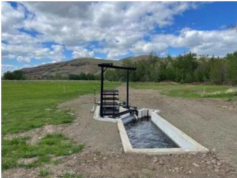
Figure 24. 2024049: New fish screen for the South Fork Walla Walla River POD
