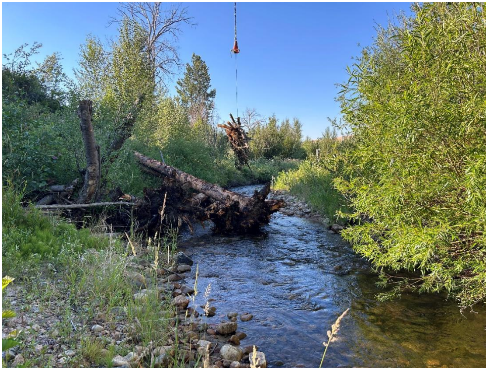
Figure 29. 2024077: Logs and slash bundles being dropped in Beaver creek site 3, slash bundles positioned in creek perpendicular to flow for ease of PAL construction.
