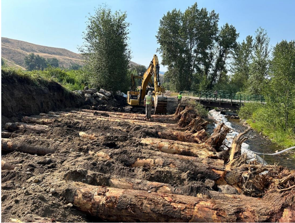
Figure 30. 2024077: Bank attached jam under construction with bridge in background.
