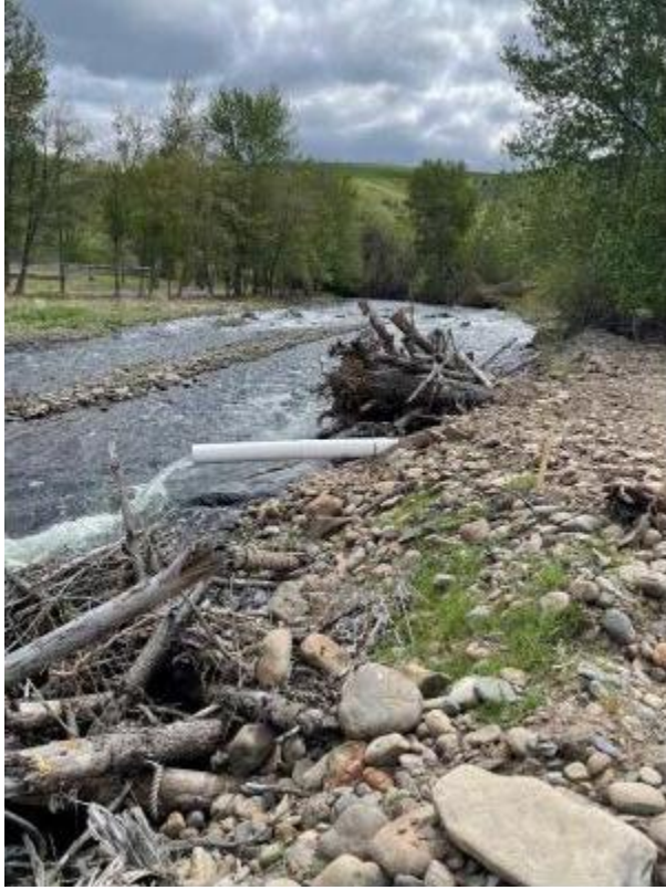
Figure 25. 2024049: New fish bypass pipe discharging to pool near large wood structure
