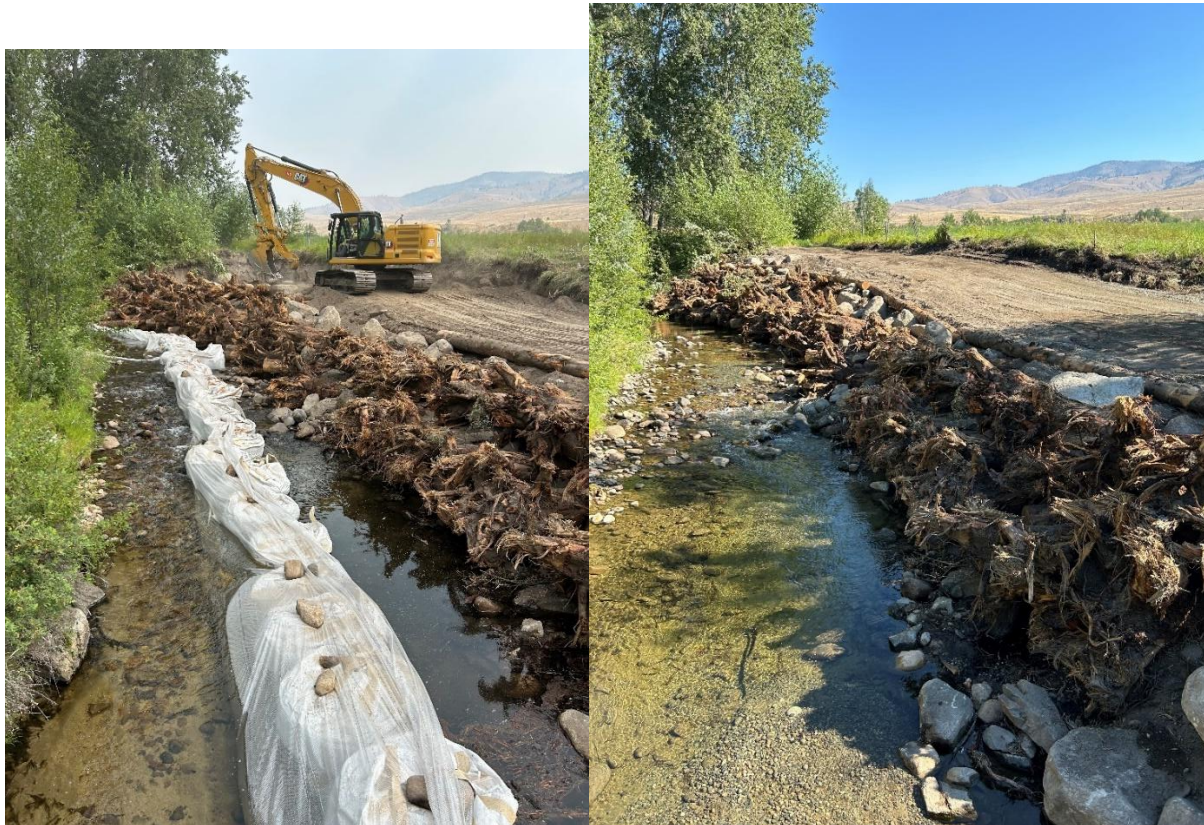
Figure 31: 2024077: Cofferdam positioned to exclude fish from the jam.
