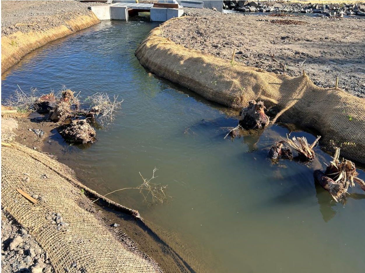
Figure 36. 2024086: Channel with rootwads between point of diversion and fish screen
