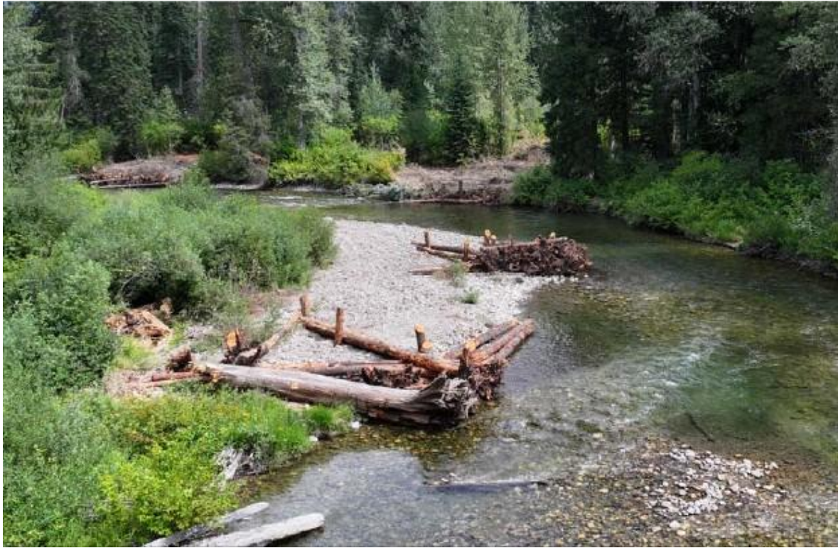
Figure 1. 2024002: Large wood structures on the Chiwawa River for the Chiwawa Outlet Fish Habitat Restoration Project.
