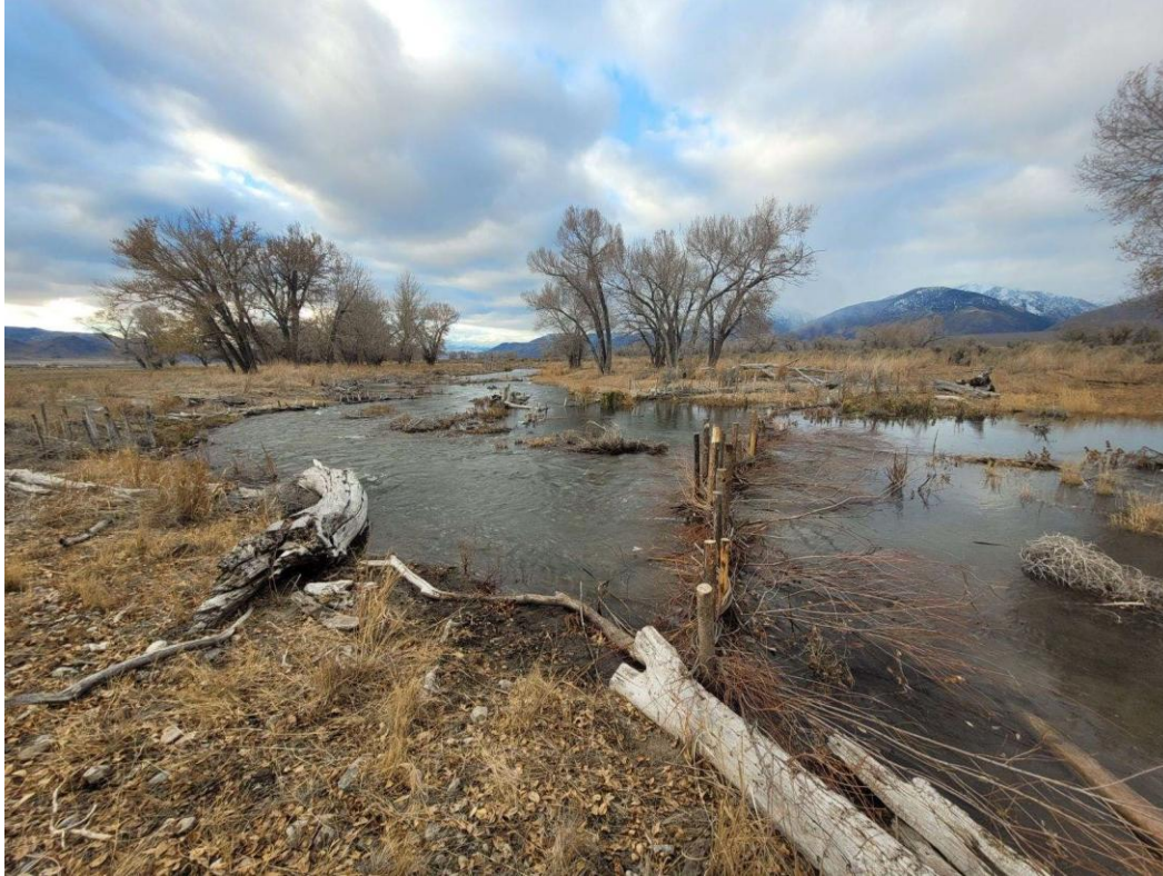
Figure 5. 2024076: BDA structure with willows on the Pahsimeroi River in Idaho.
