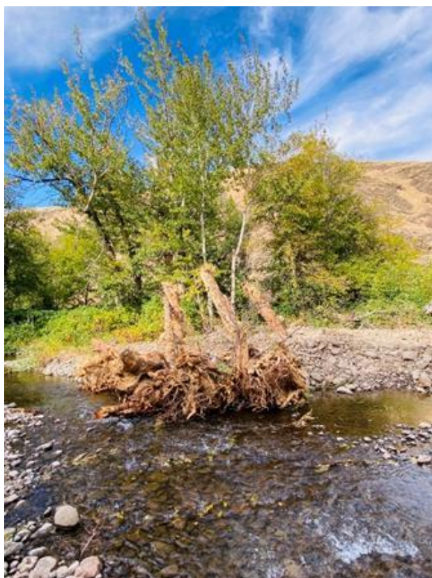
Figure 34. ELJ structure near RM 5.2 provides fish habitat uplift
