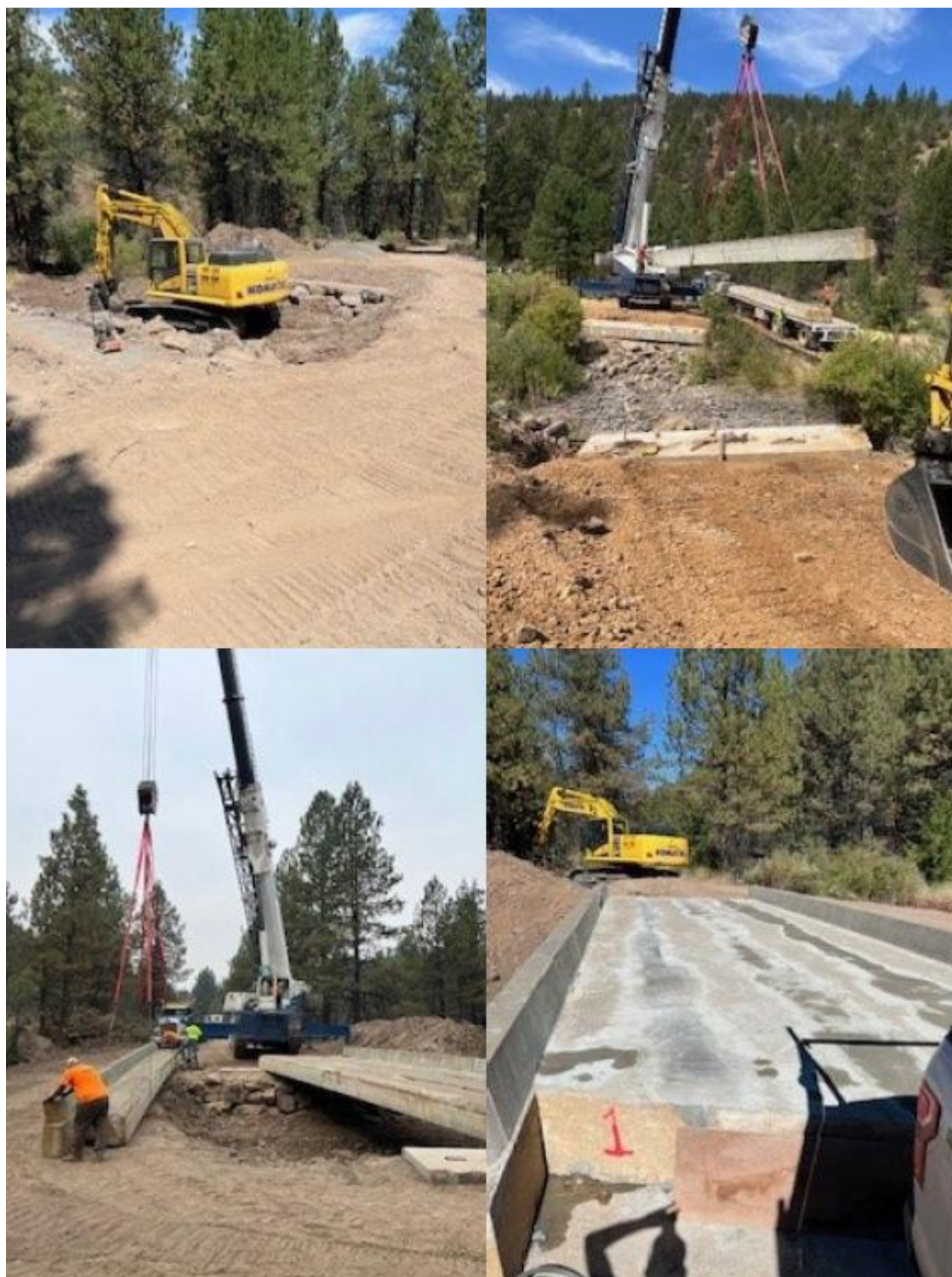
Figure 12. 2024009: Bridge installed at the Dutchman Creek crossing
