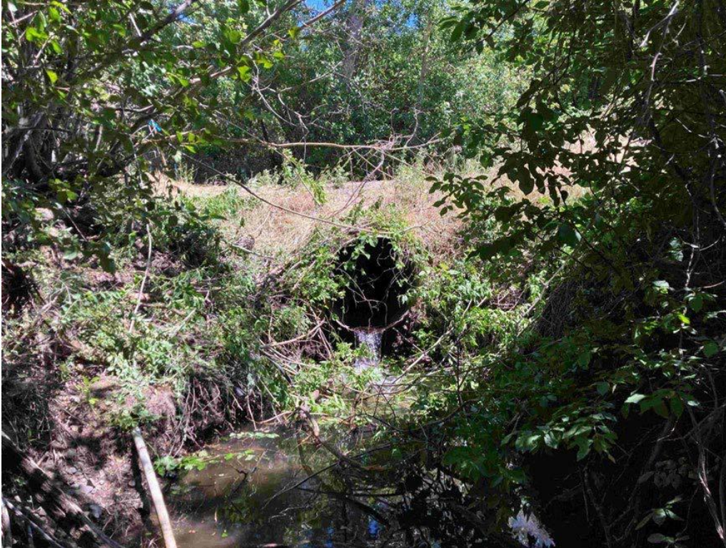
Figure 20. 2024039: Culvert to be removed prior to construction
