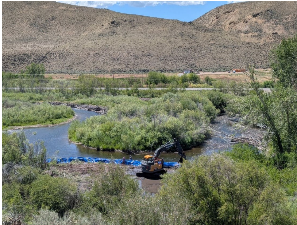
Figure 10. 2025058: Installation of in-water construction isolation measures (cofferdam and turbidity control) to support Phase 2 construction in the Lemhi River.
