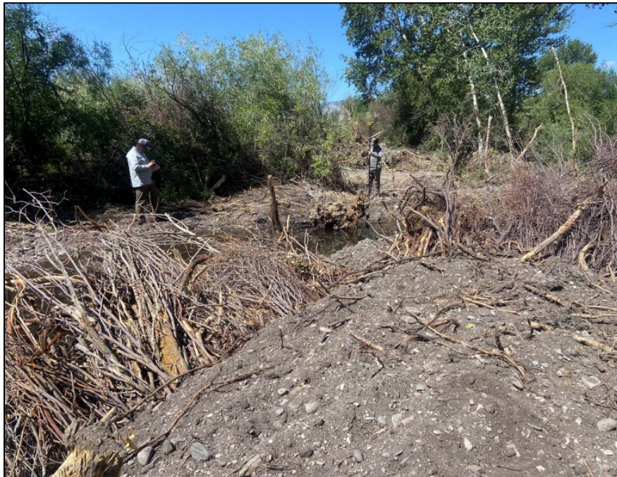
Figure 4. 2025031: Engineers checking finished grade of installed structures.
