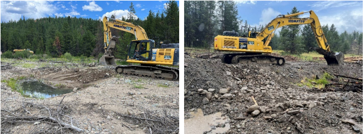
Figure 22. 2025078: Contractor excavating floodplain pools (left) and developing debris control structures (right).
