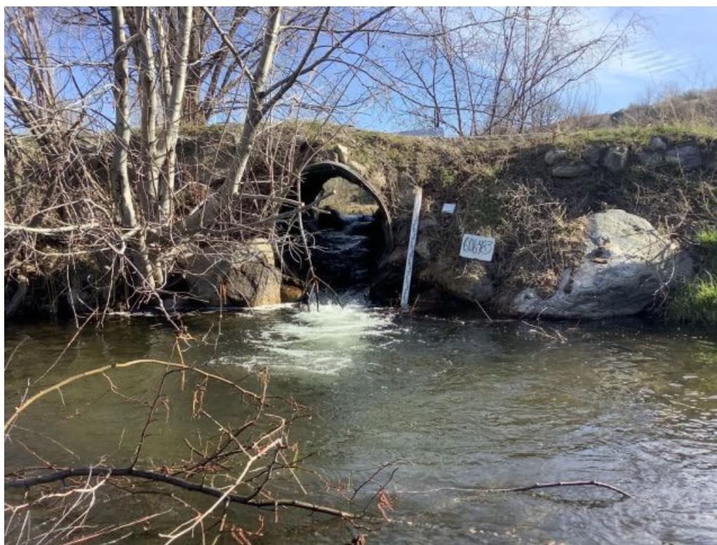
Figure 25. 2025095: Pre-project view of the Whiskey Cache Rd. culvert that was replaced as part of the project.
