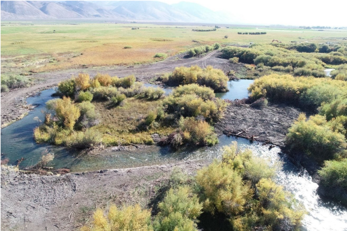
Figure 6. 2025034: Channel plug and newly excavated channel on the main Pahsimeroi River, with view of downstream riffle in the new channel.
