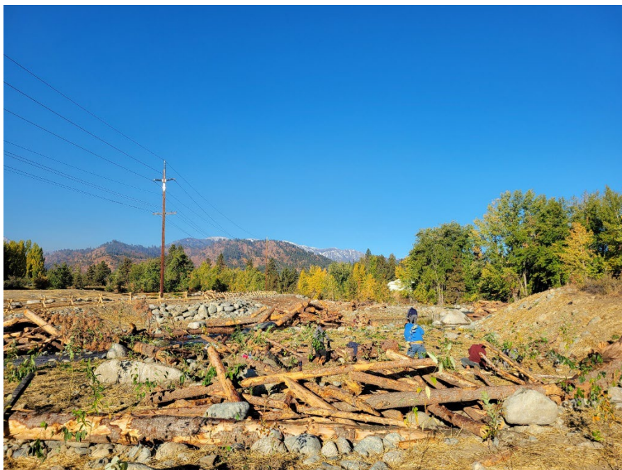
Figure 9. 2025052. Floodplain plant installation.
