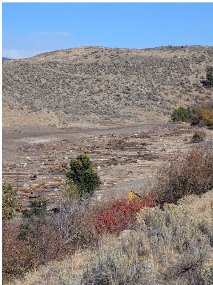
Figure 26. 2025095: Post-project overview of a newly created 215-foot-wide floodplain with buried logs, slash piles, BDAs and surface roughness features to reduce stream power and channel incision.
