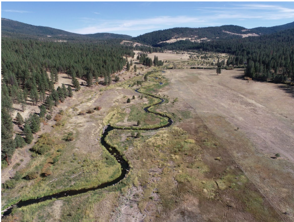
Figure 16. 2025073: Pre-project photo of Middle Fork John Day River at Oxbow Conservation Area.
