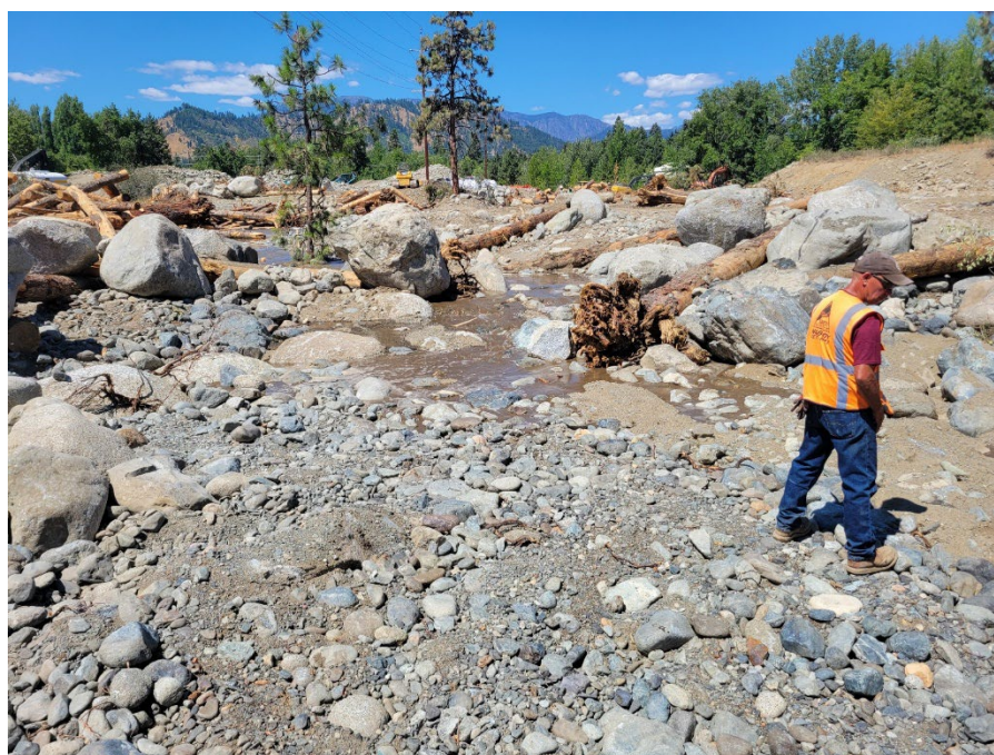
Figure 8. 2025052: Staged rewatering of primary channel.
