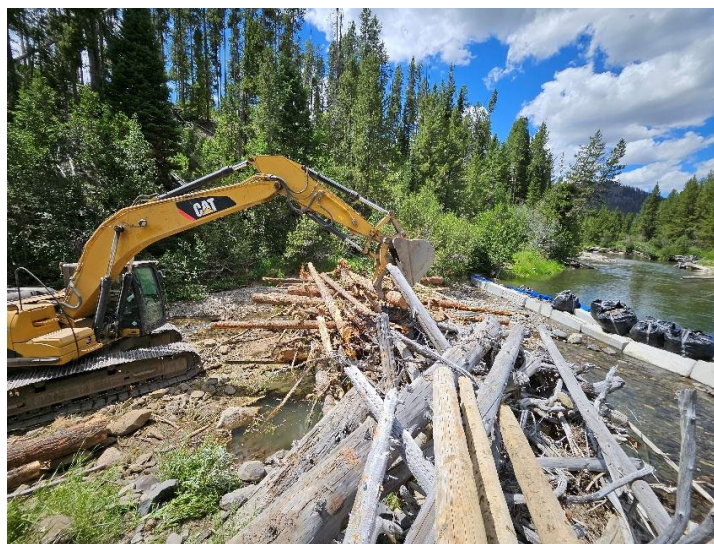
Figure 20. 2025075: Constructing the bleeder jam at the upper meander.
