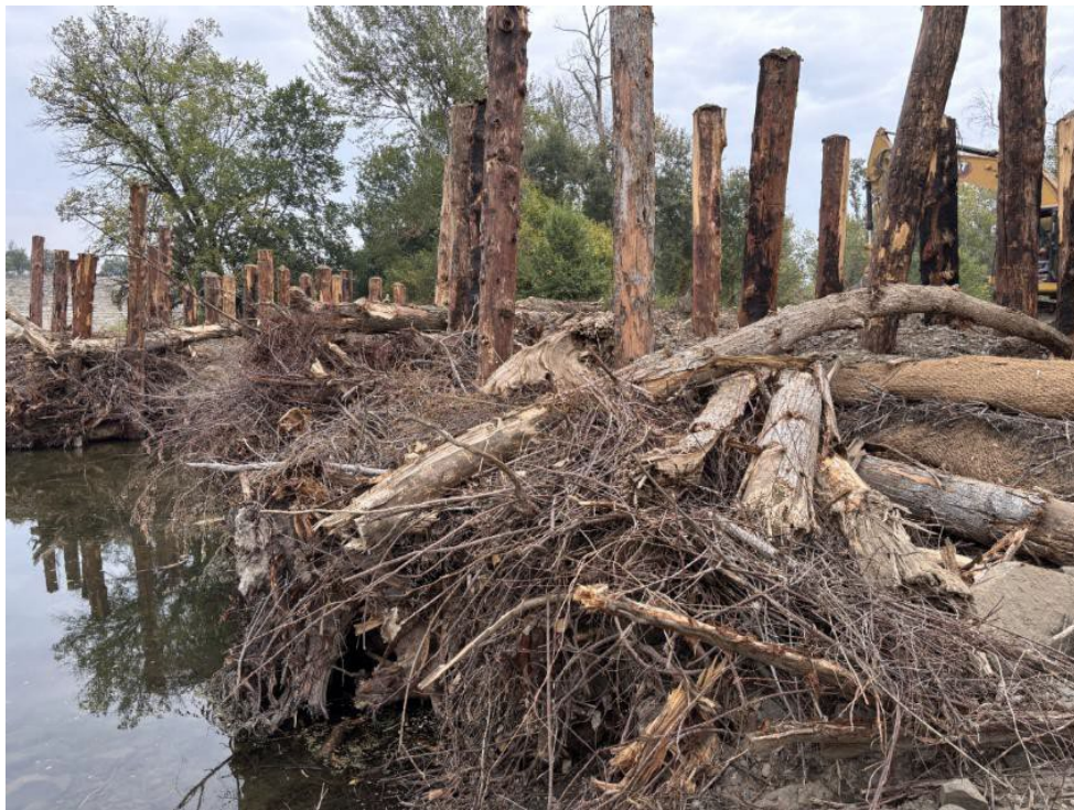
Figure 30. 2025097: Newly installed ELJ at downstream end of project.
