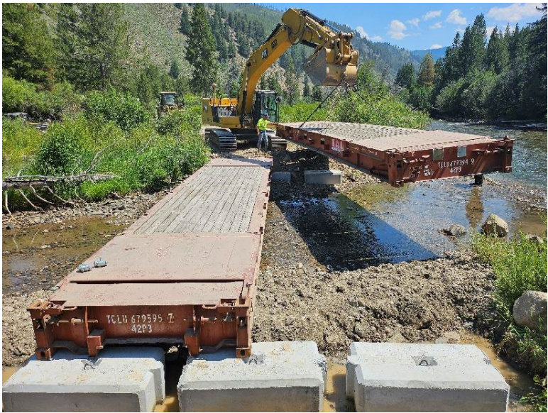
Figure 21. 2025075: Setting the temporary work bridge to access the upper meander area.
