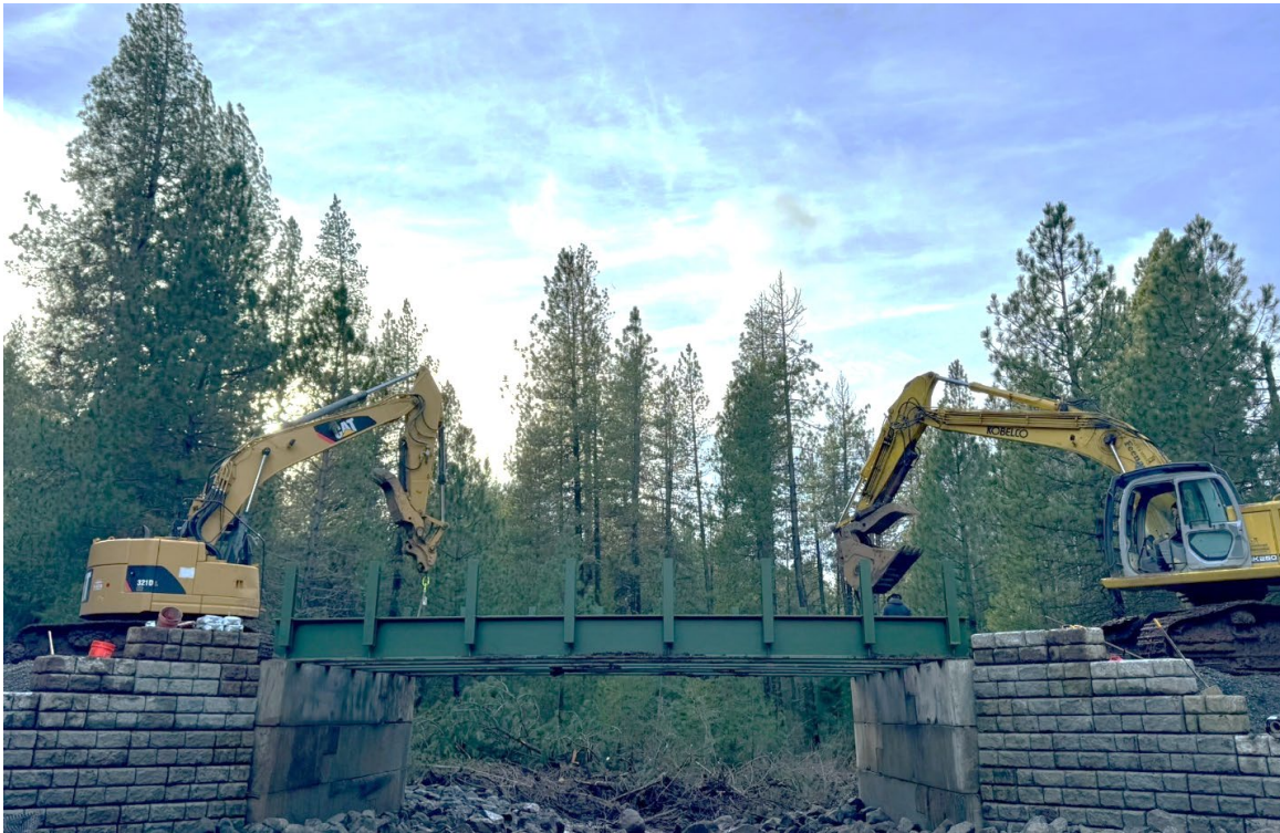
Figure 1. 2025026: Replacement of undersized culverts with this bridge over Brush Creek improved access to 3.5 miles of habitat for ESA-listed steelhead trout.
