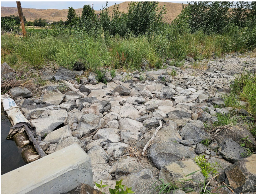
Figure 37. 2024086: Purdin Ditch roughened channel in 2026.
