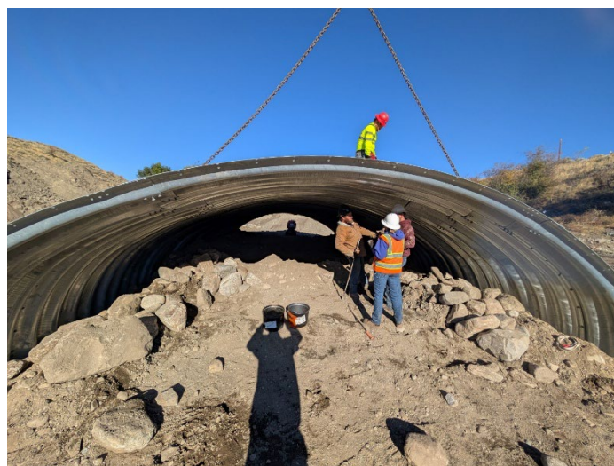
Figure 27. 2025095: Installation of 60-foot-long, 32-foot-span bottomless culvert to replace the undersized culvert at Whiskey Cache Rd.
