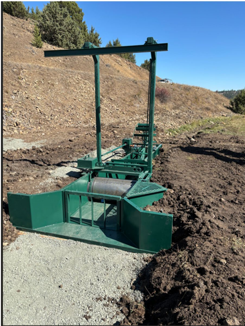
Figure 38. 2025096: ODFW prefabricated fish screen at Badger Creek site.
