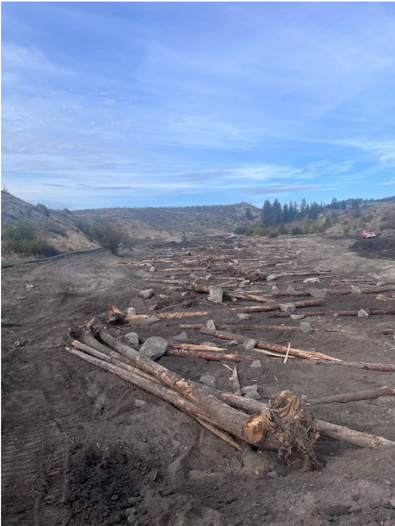
Figure 28. 2025095: Floodplain reconnection upstream of Whiskey Cache Rd culvert.
