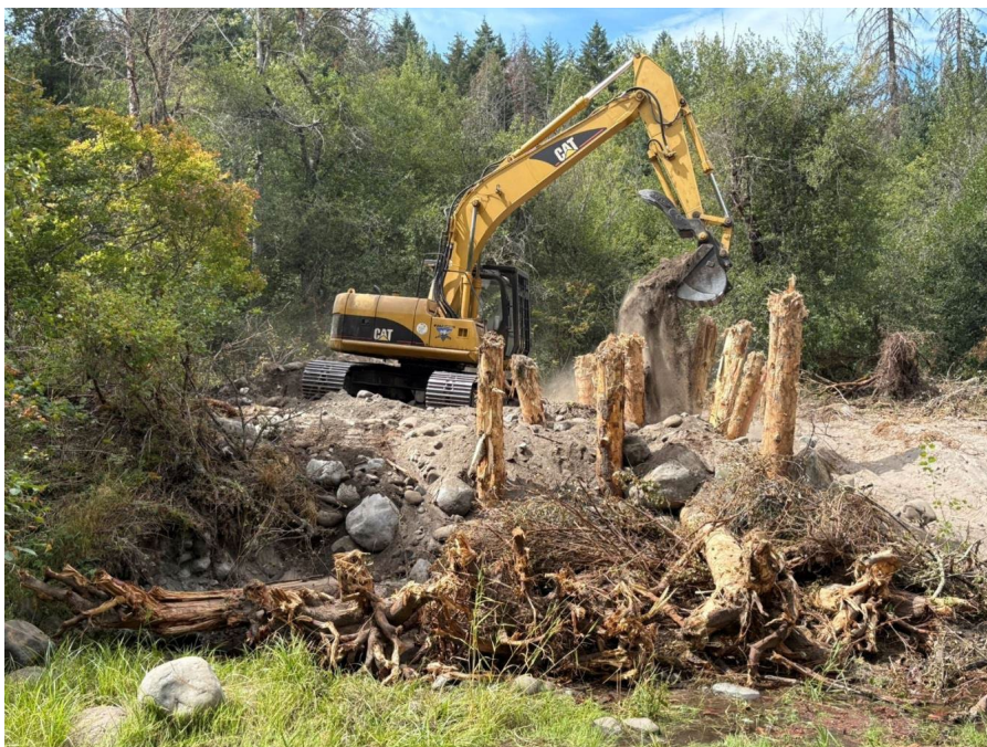
Figure 12. 2025068: Construction of bank habitat structure in dry Kulongoski Channel.
