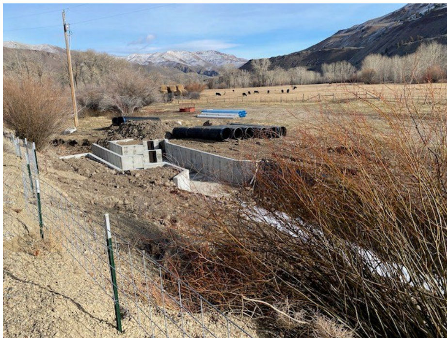
Figure 39. 2025012: Concrete for new IDFG fish screen in upper Salmon River basin.
