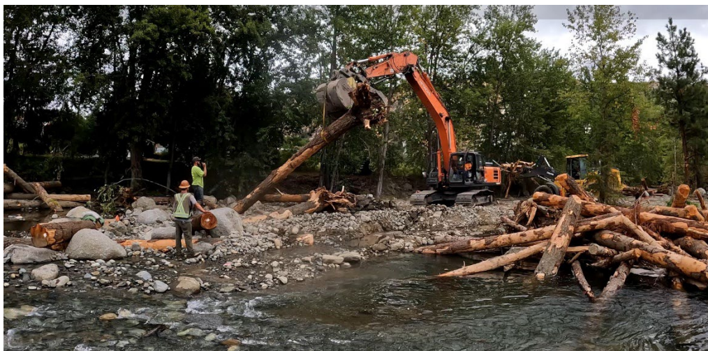
Figure 7. 2025052: Construction of engineered log jam on Peshastin Creek.
