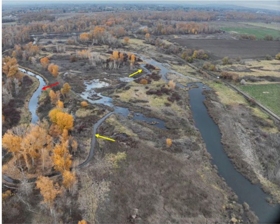
Figure 29. 2025097: Upper portion of project area post-project. Yellow areas indicate newly excavated channels. Red arrow notes an existing side channel.
