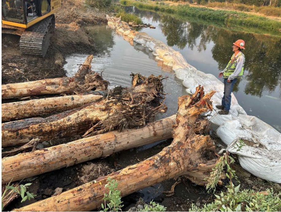
Figure 31. 2025097: ELJ footer log installation within isolated work area.
