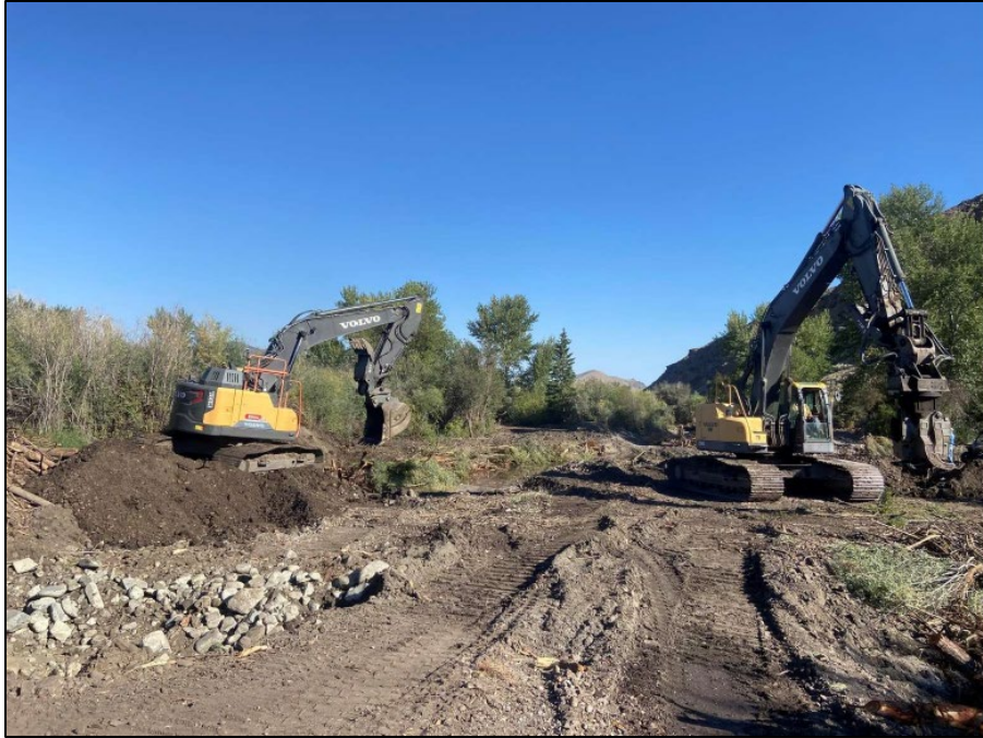
Figure 3. 2025031: Excavators working together to complete structures on the river left bank of the main channel.
