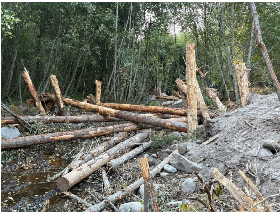
Figure 13. 2025068: Construction of channel-spanning PALS in dry river left Mills Channel.
