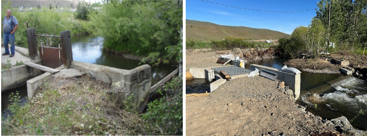
Figure 36. 2024086: Before (top) and after (bottom) photos of the diversion
