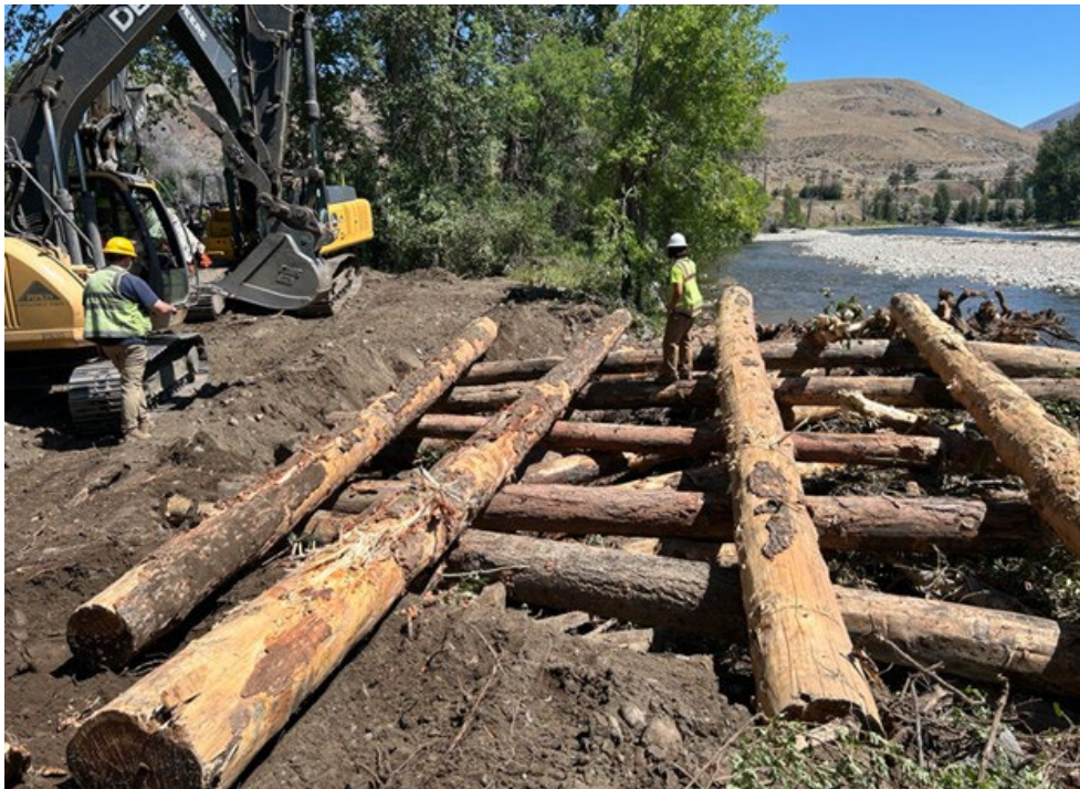
Figure 2. 2025080: Installation of bank-attached log jam on the Methow River.
