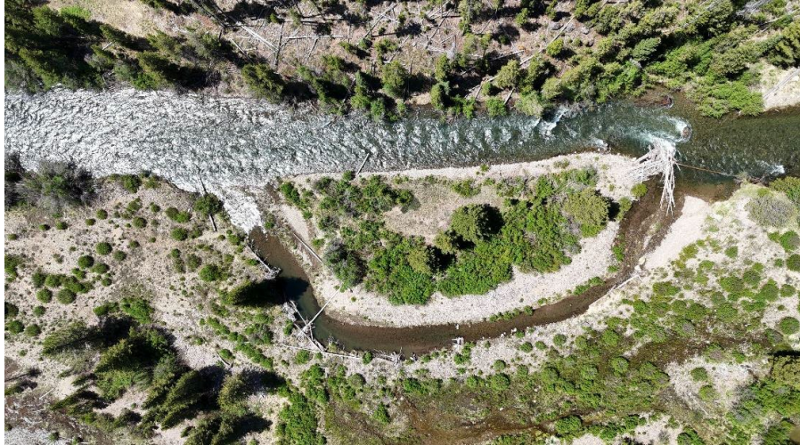
Figure 18. 2025075: Upper meander on the Yankee Fork River before construction.
