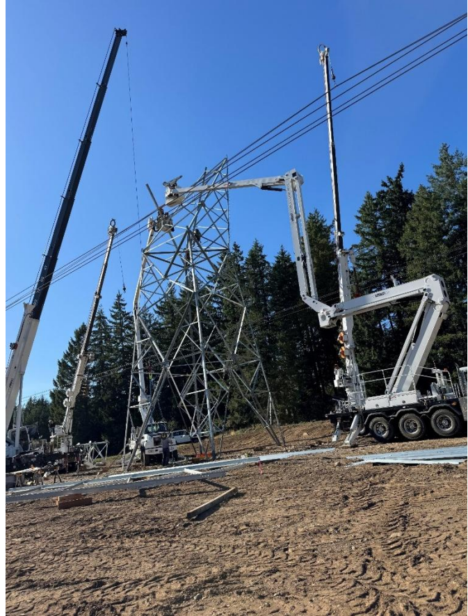
Construction of a prop structure to remediate a clearance concern near Covington, Washington. (Photo by Travis A.)
