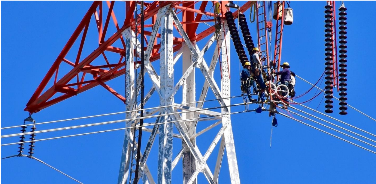
Transmission line insulator replacement near Bonneville Dam. (Photo by Rob M.)
