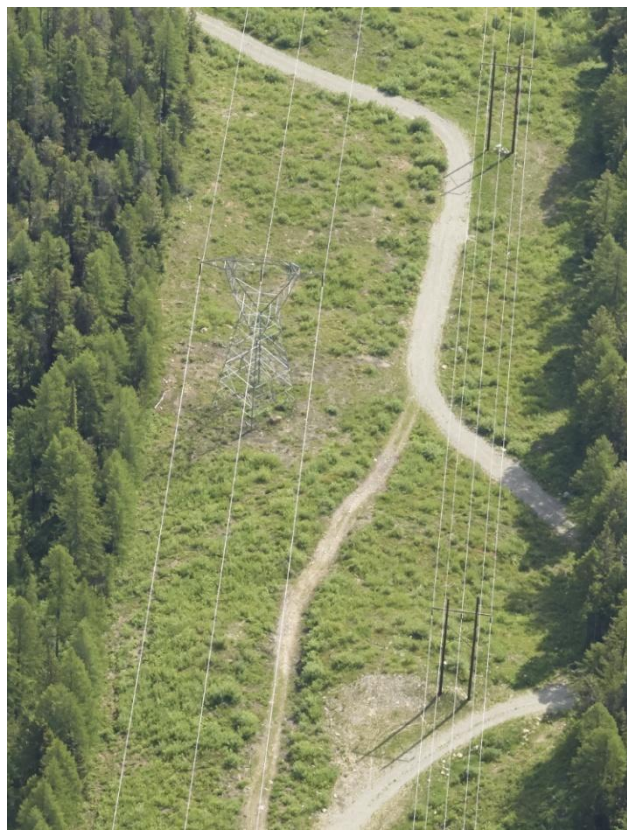
Access road network along BPA transmission lines near Flathead Lake in Montana.
