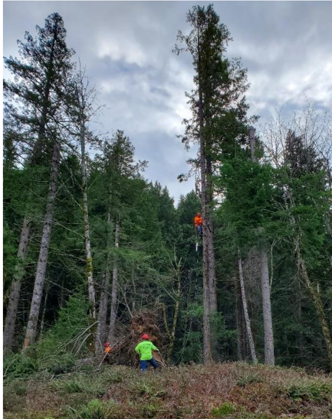
Tree removal along a BPA ROW corridor.
