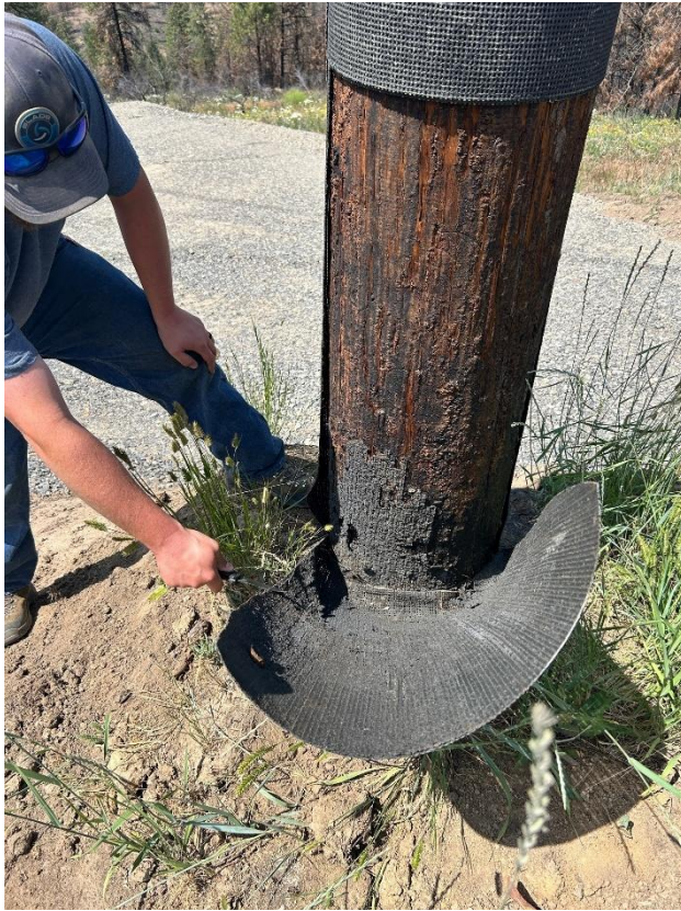
Fire retardant wrap after the 2024 Swawilla I Fire near Keller, Washington.
