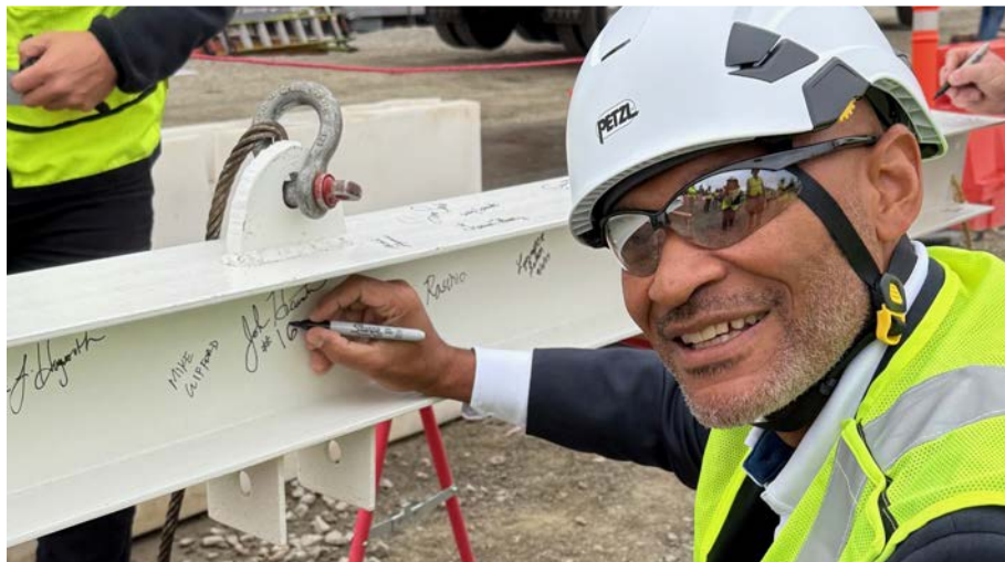
Administrator Hairston signs the final beam before it is placed on top of the new Vancouver Control Center
