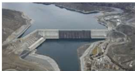
Grand Coulee 33 Units 6,998 MW 1
