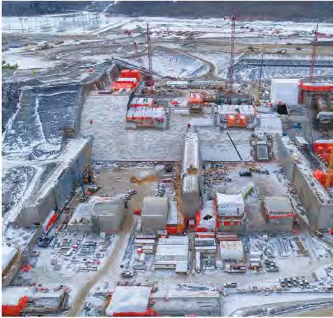
*Site C Hydroelectric Project winter construction in northern BC.
