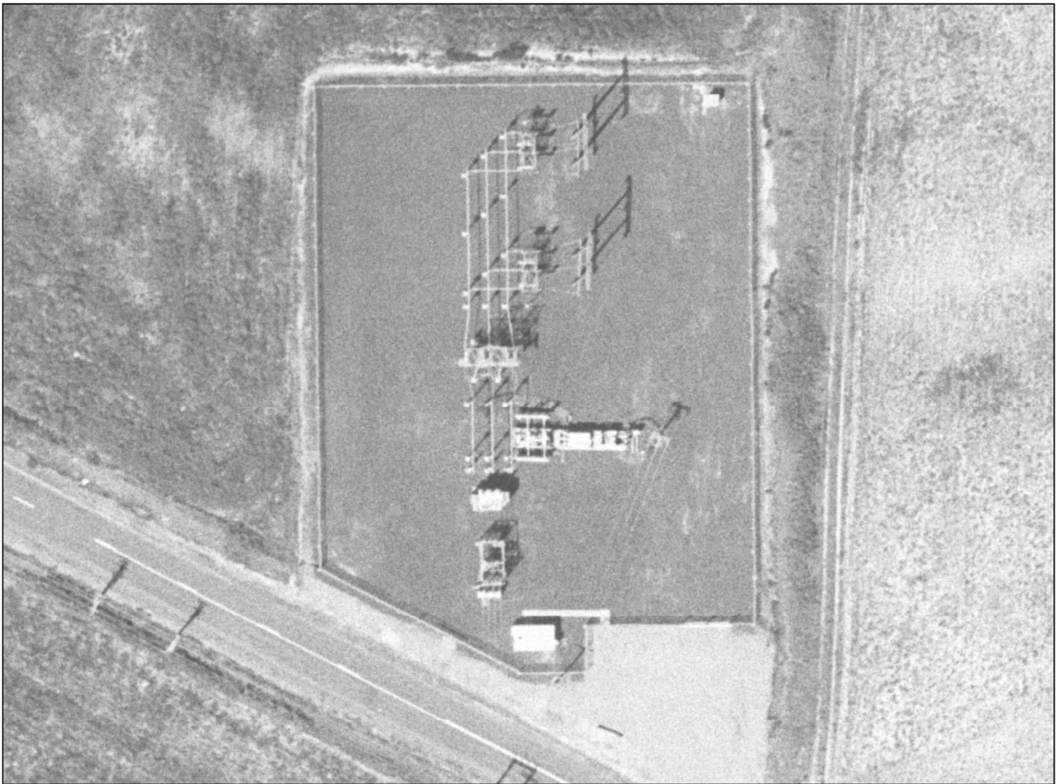
Spring Hill Substation
