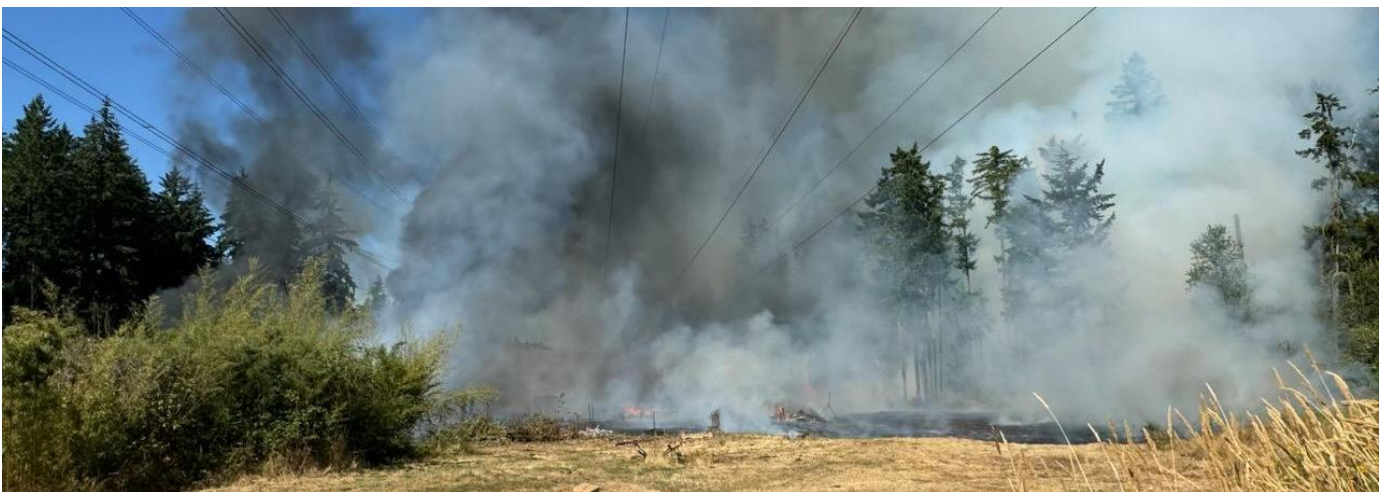
Smoke from a wildfire above BPA transmission lines.
